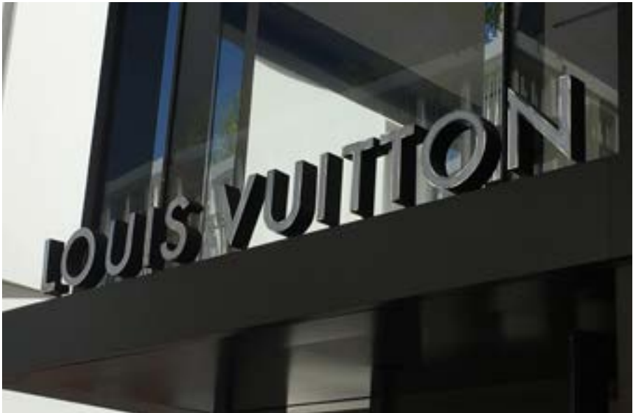
PROJECTING PLEXI FRONT LETTERS WITH METAL BODY ATTACHED TO THE TOP OF THE CANOPY OR AWNING
