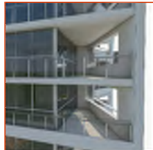
ANODIZED ALUM & GLASS WINDOW-WALL AND BALCONY RAILS
