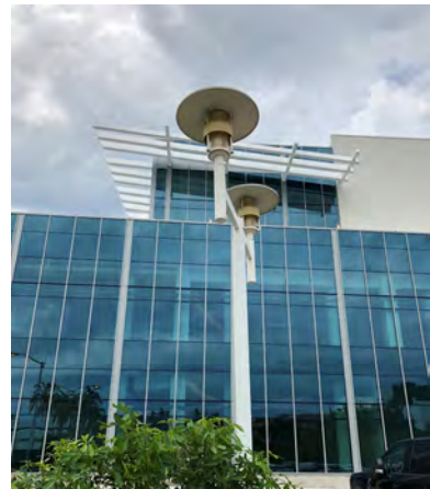
Figure 5 - Typical fixture within the Convention Center District
