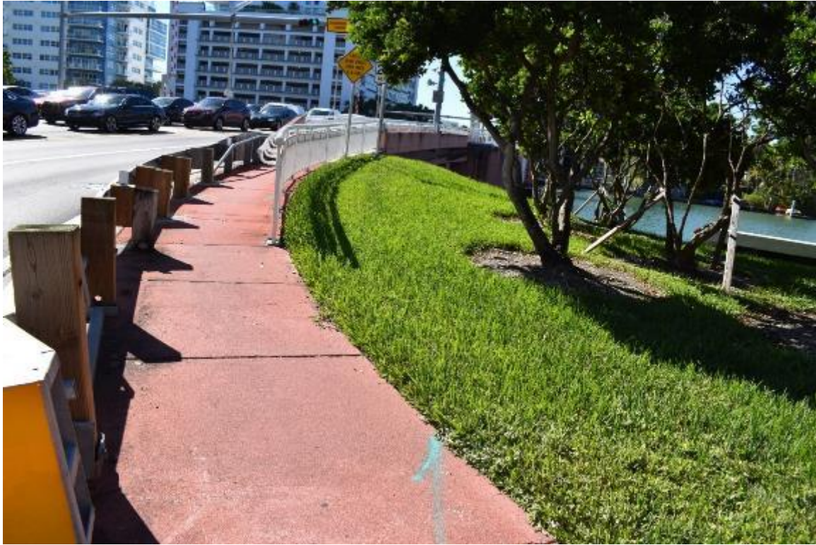
Photo 7 View of sidewalk area and easement area
