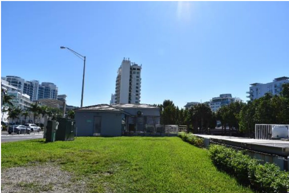
Photo 5 View of pump station looking southerly from driveway
