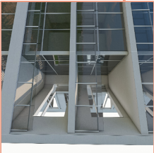
ANODIZED ALUM. GLASS WINDOW-WALL AND BALCONY RAILS
