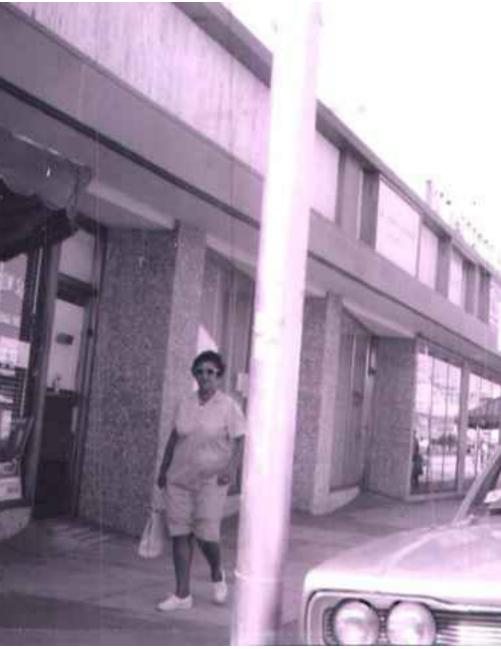
RETAIL WAS ANGLED AND SMALLER SCALED - THIS BUILDING HAS BEEN SUBSTANTIALLY MODIFIED FROM ORIGINAL DESIGN - IT APPEARS THAT NO ORIGINAL GEOMETRY OR MATERIALS WERE KEPT IN EXISTING FACADE.
