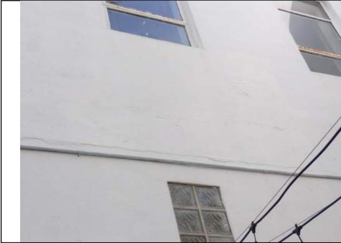
North Elevation Hairline Cracks
