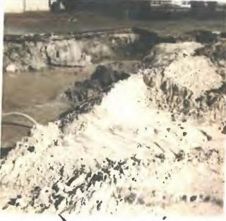
Picture Explanation: View of groundwater with slight layer of emulsified HC.
