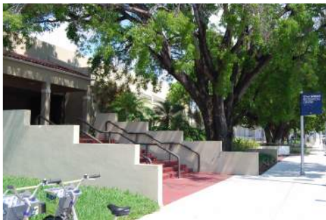
21st STREET RECREATION CENTER
