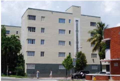
2115 WASHINGTON AVENUE @ (5 floors)
