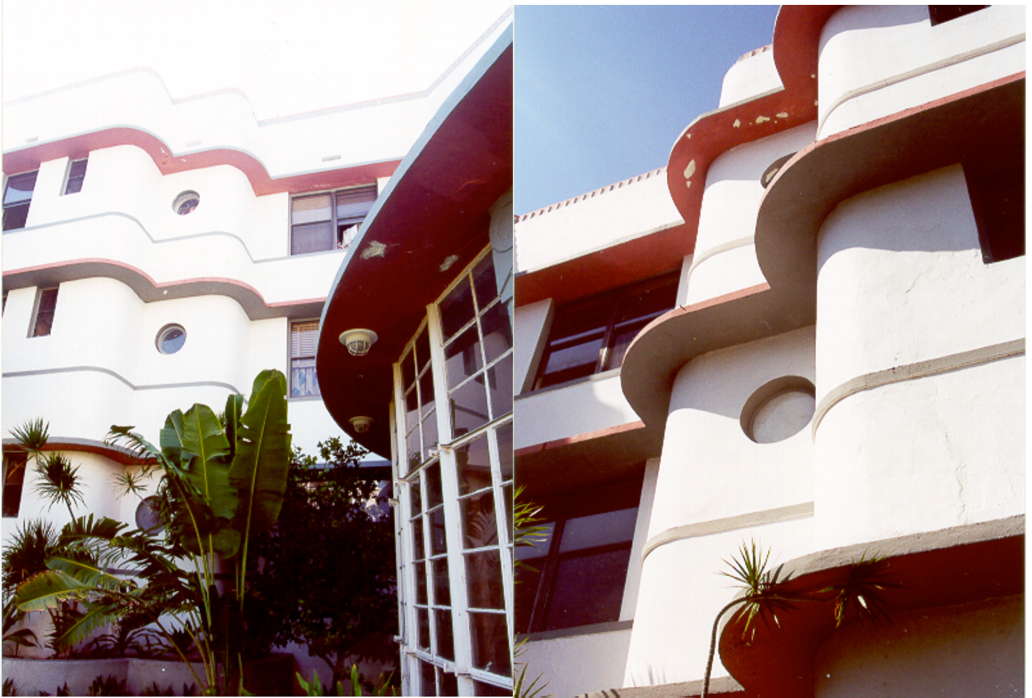
COLLINS PARK: EXTERIOR FRONT ELEVATION VIEWS 1999
