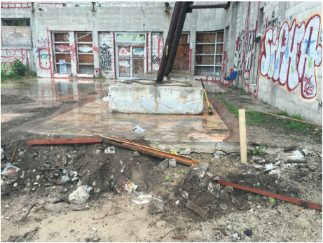
2 2012 PHOTOGRAPH LOBBY VIEW TOWARDS FRONT ENTRANCE
