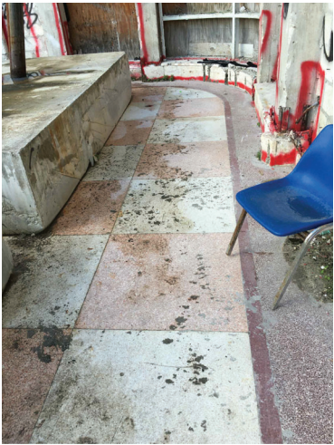
1 2012 PHOTOGRAPH LOBBY TERRAZZO PATTERN
