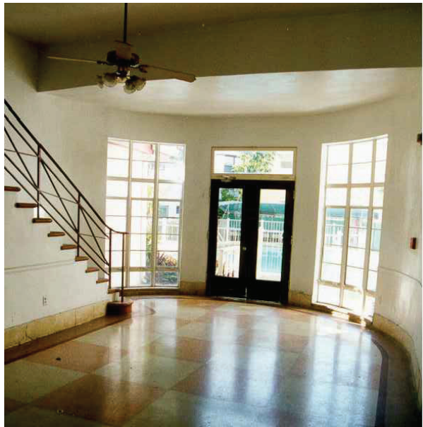
3 1999 PHOTOGRAPH LOBBY TERRAZZO AT REAR
