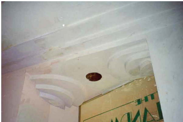
5 1999 PHOTOGRAPH TYPICAL CEILING DETAILS & NON HISTORIC SIGNAGE
