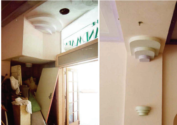
6 1999 PHOTOGRAPH TYPICAL CEILING DETAILS
