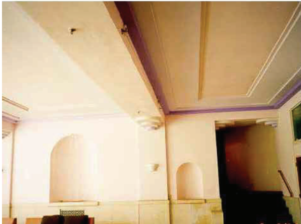
4 1999 PHOTOGRAPH TYPICAL LOBBY TRAY CEILING DETAILS
