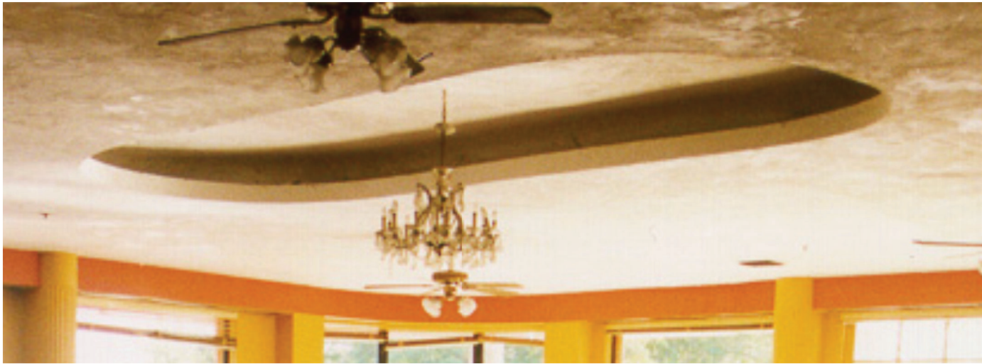
1999 PHOTO OF LOBBY CEILING COVE
