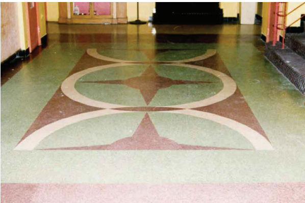
4 2000 PHOTOGRAPH TERRAZZO FLOOR PATTERN
