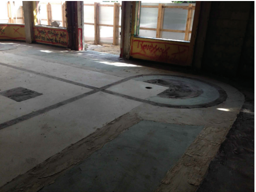
3 2014 PHOTOGRAPH LOBBY TERRAZZO PATTERN
