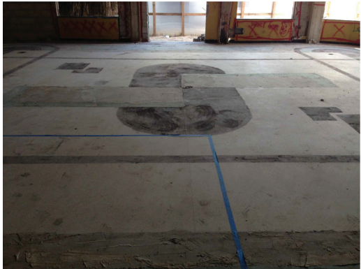
2 2014 PHOTOGRAPH LOBBY TERRAZZO PATTERN
