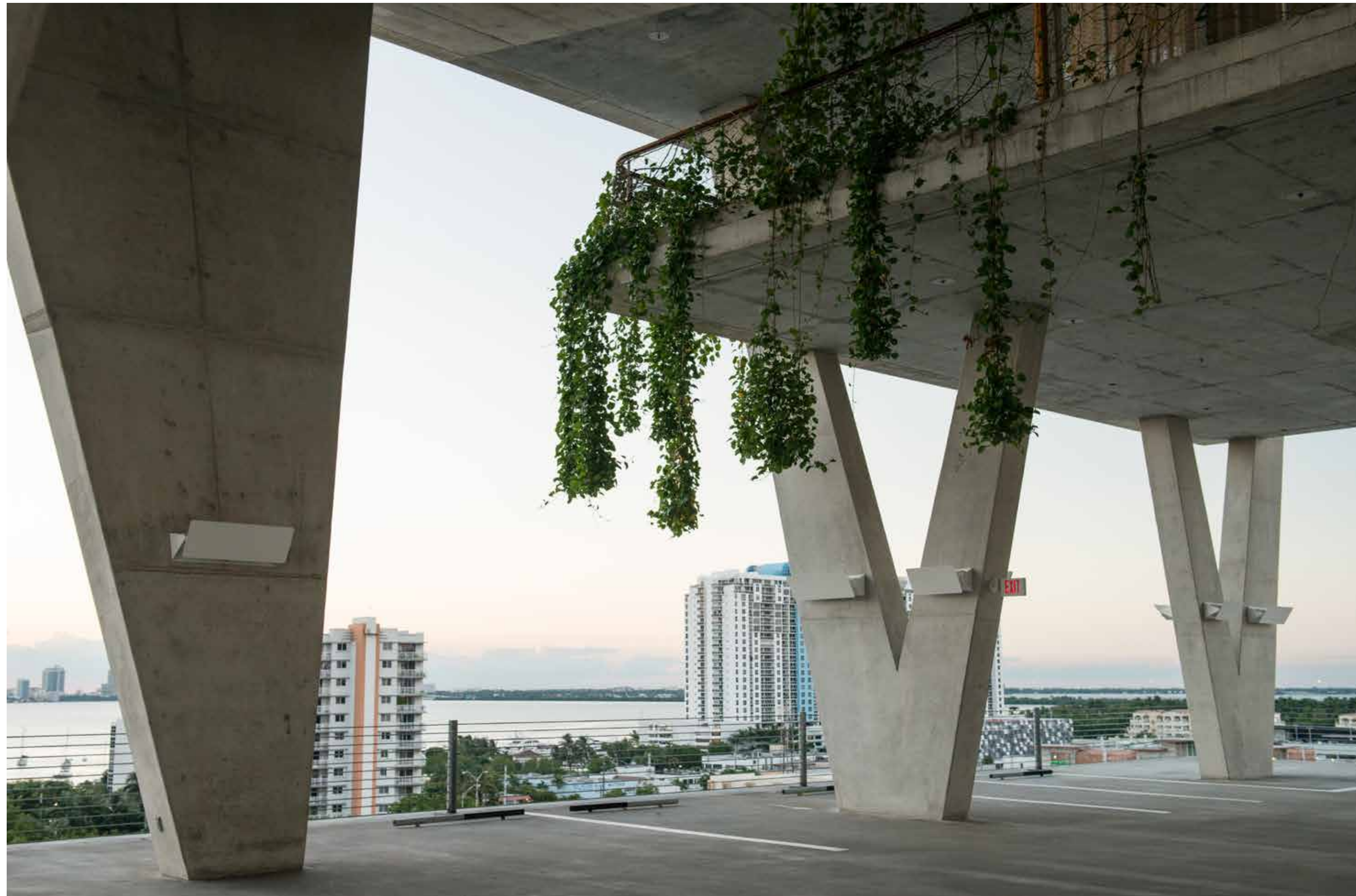
CANTILEVERED CONCRETE ROOF WITH CASCADING VINES
