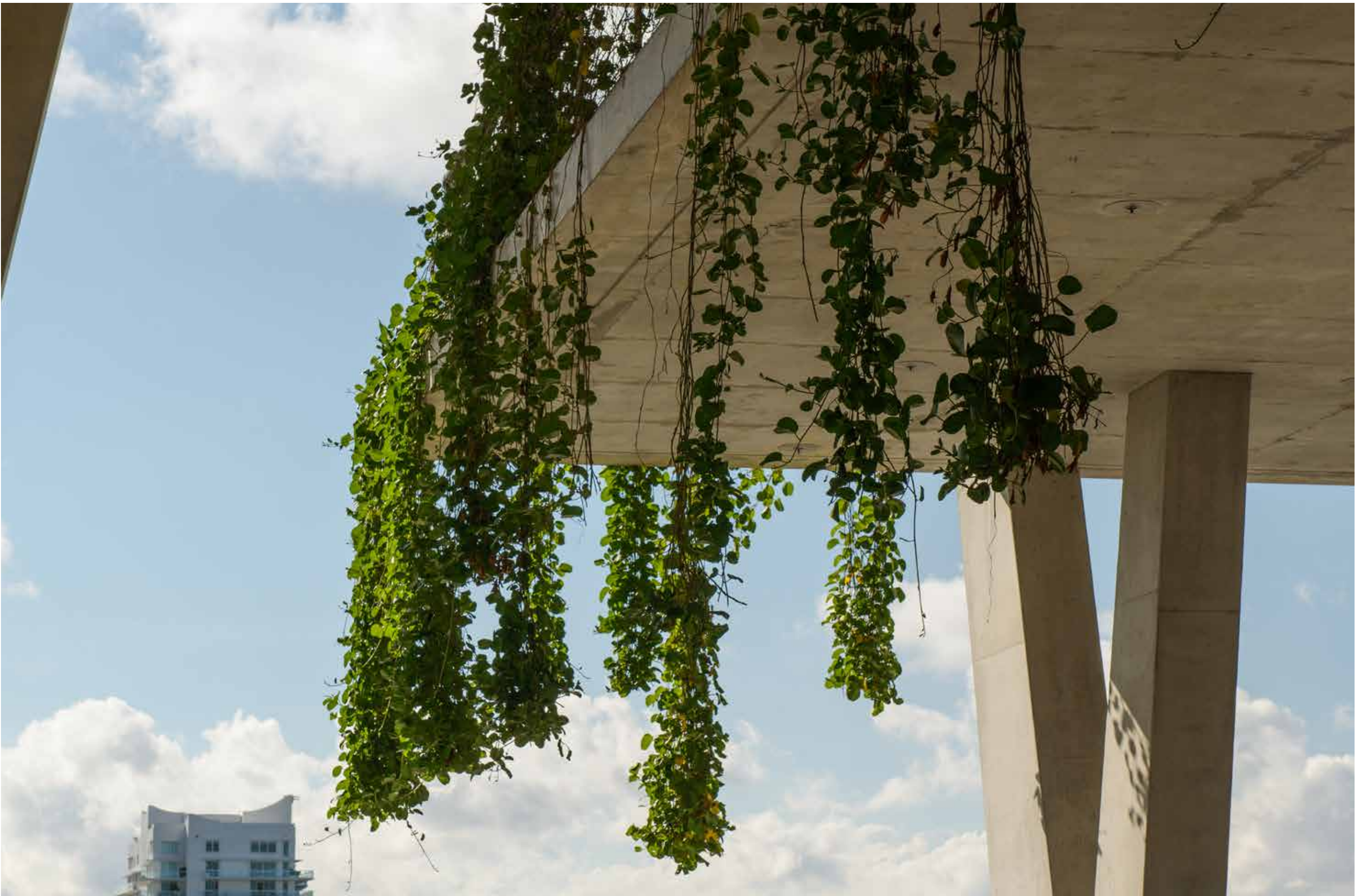
CANTILEVERED CONCRETE ROOF WITH CASCADING VINES
