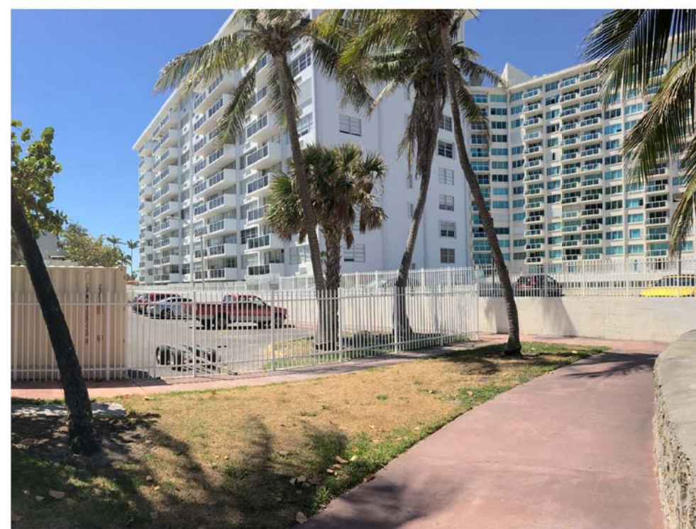
R (04/17/2018) EXISTING FIRE STATION PARKING REAR VIEW 2/2 Scale: N.T.S.
