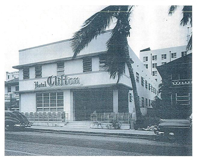
As part of the renovation of the building the applicant is proposing to replace the existing nonoriginal windows with new impact windows with a historically accurate muntin configuration. Additionally, the original neon sign is proposed to be restored. In summary, staff is supportive of the overall project and recommends approval as noted below.
