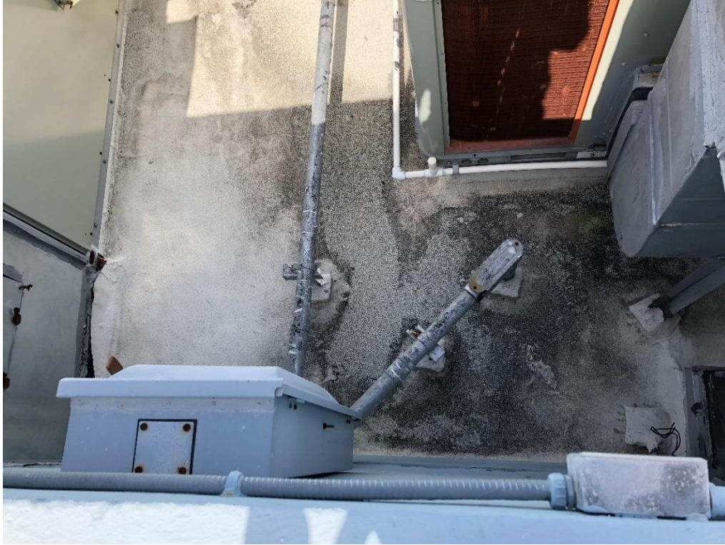
Photograph No. 23 – Deteriorated roofing at Eastern Lower Roof
