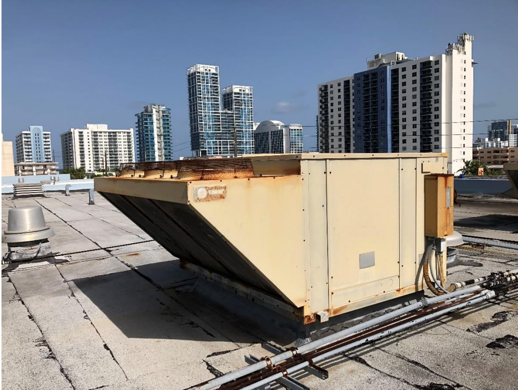
Photograph No. 21 - Rooftop Package Unit at Western Upper Roof
