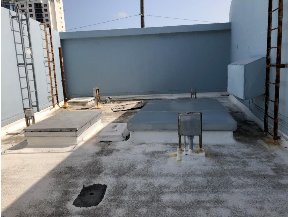
Photograph No. 61 – Covered Opening at Low Roof between East and West
