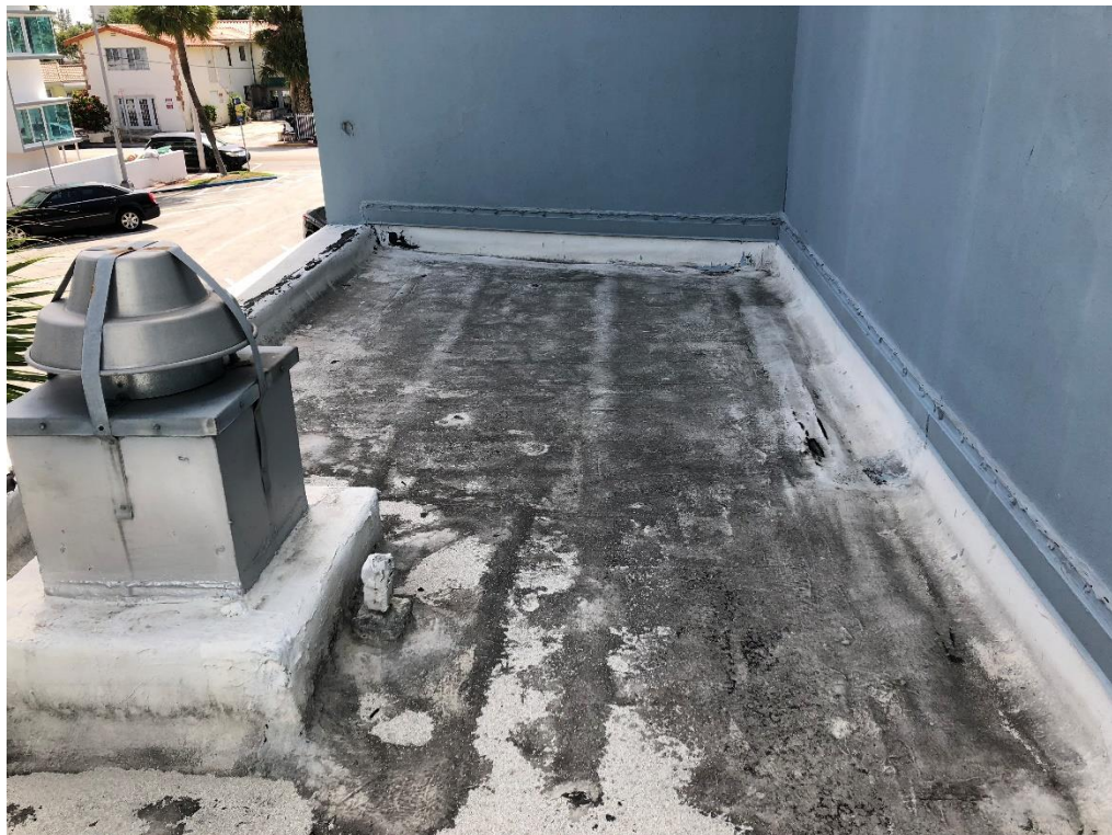
Photograph No. 24 – Deteriorated roofing at Lower Roof at the 2 nd Floor towards South Façade
