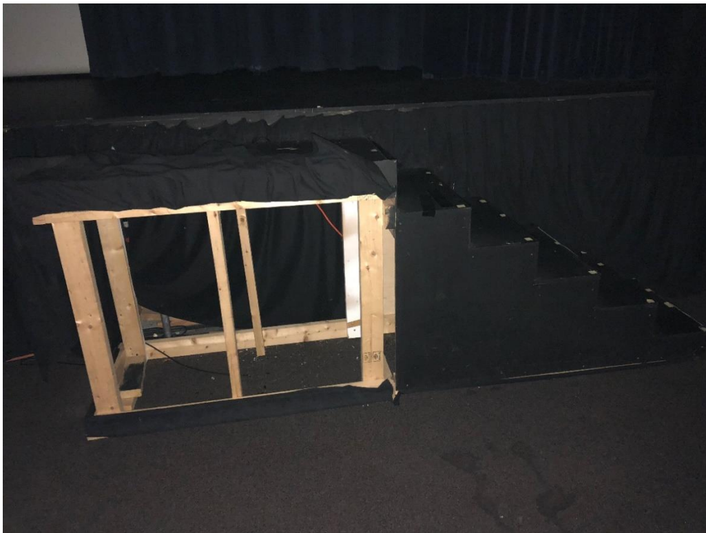
Photograph No. 34 – Wood-framed staircase (East Cinema Theater)
