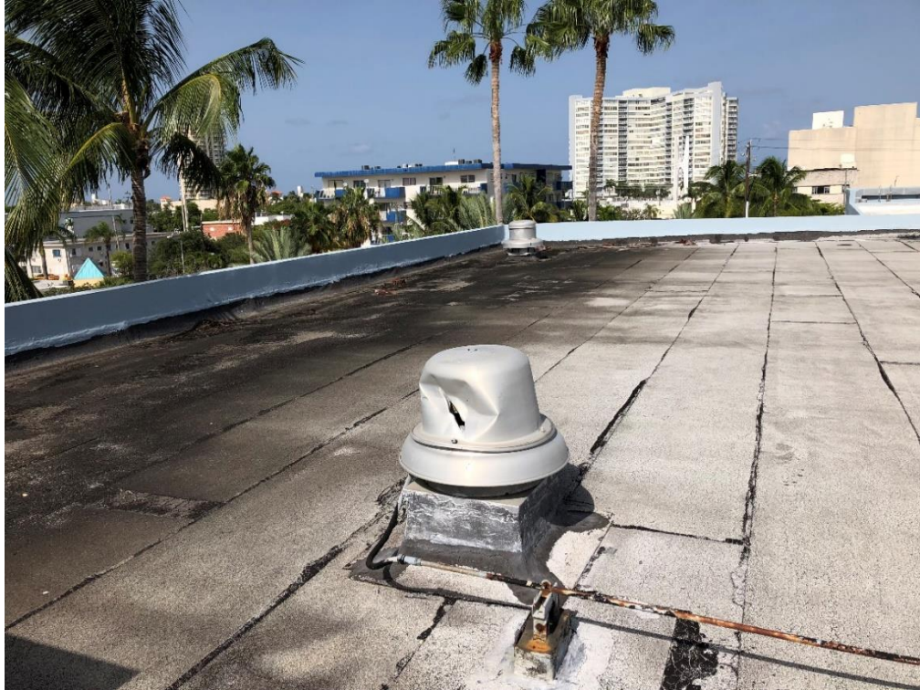
Photograph No. 25 – Deteriorated roofing at Western Upper Roof
