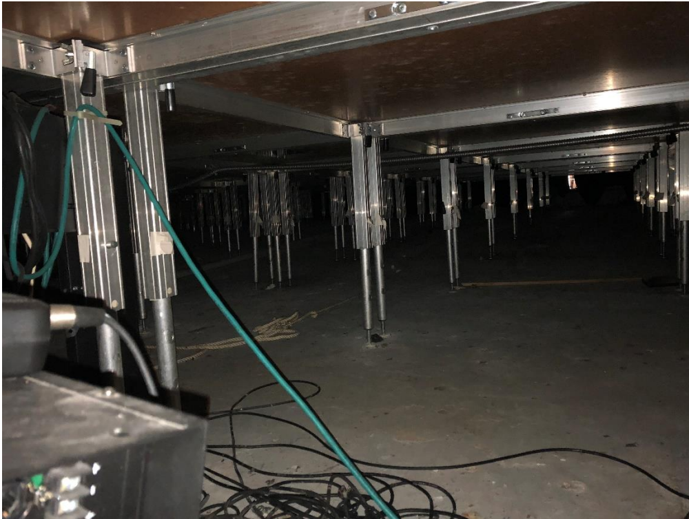
Photograph No. 7 - Aluminum-framed Stage Platform for East Cinema Theater
