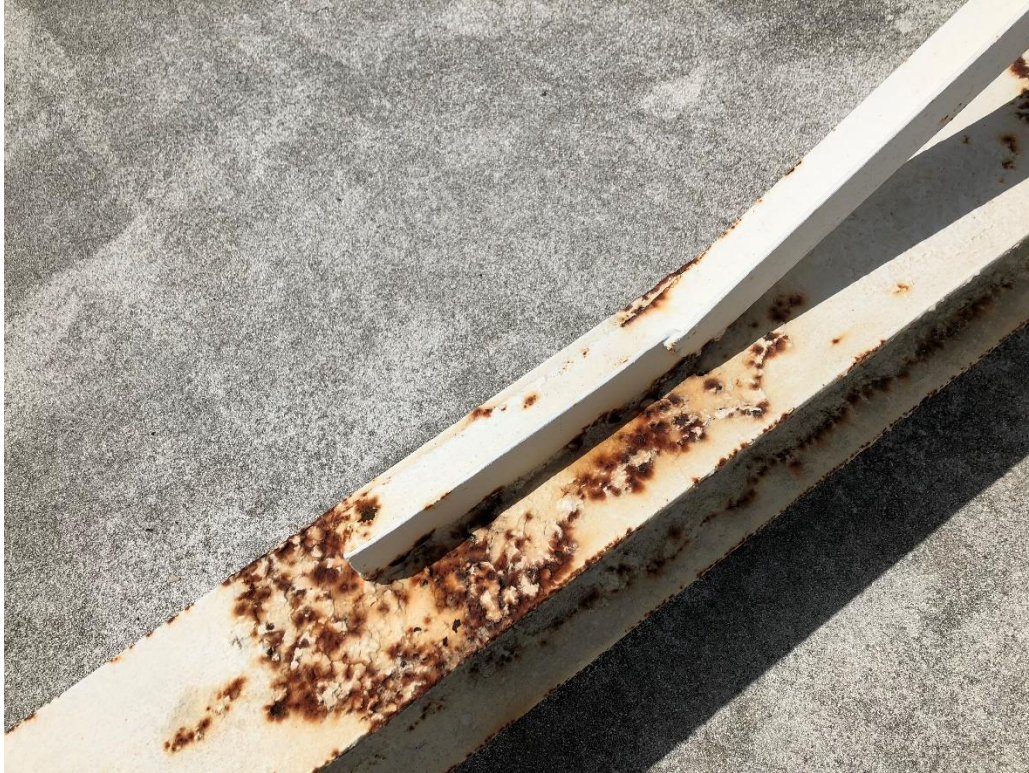
Photograph No. 19 – Corroded Structural Steel Supporting Theater Sign
