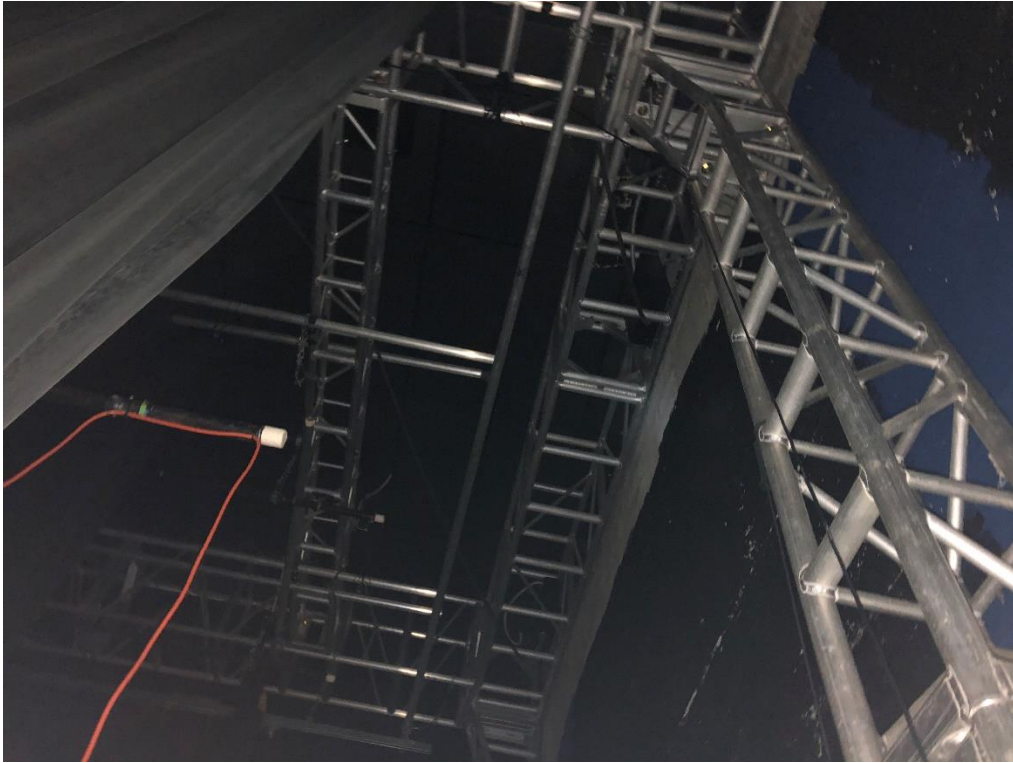
Photograph No. 79 – Aluminum Truss Frame for Lighting Support
