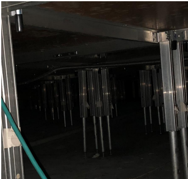
Photograph No. 78 – Crooked Leg of Stage's Aluminum-framed Platform
