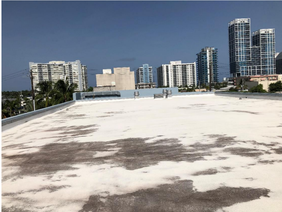
Photograph No. 27 – Deteriorated roofing at Western Upper Roof
