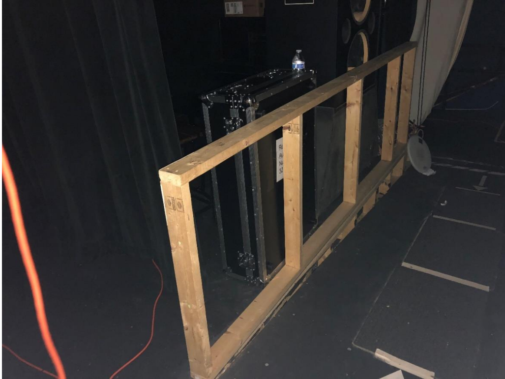
Photograph No. 37 – Loose Wooden Guardrail at East Cinema Theater
