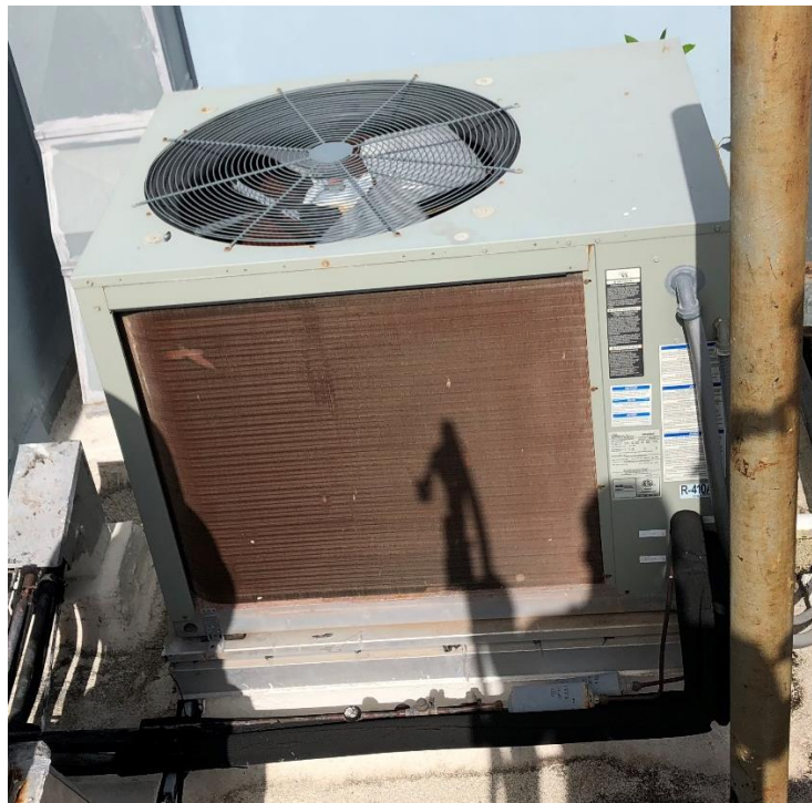
Photograph No. 62 – Condensing Unit Supported on Larger Roof Curb at Low Roof at East Side
