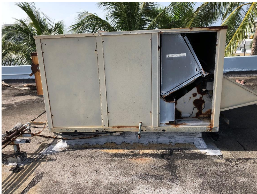
Photograph No. 64 – Package unit Unconnected to Roof Curb at Western Upper Roof
