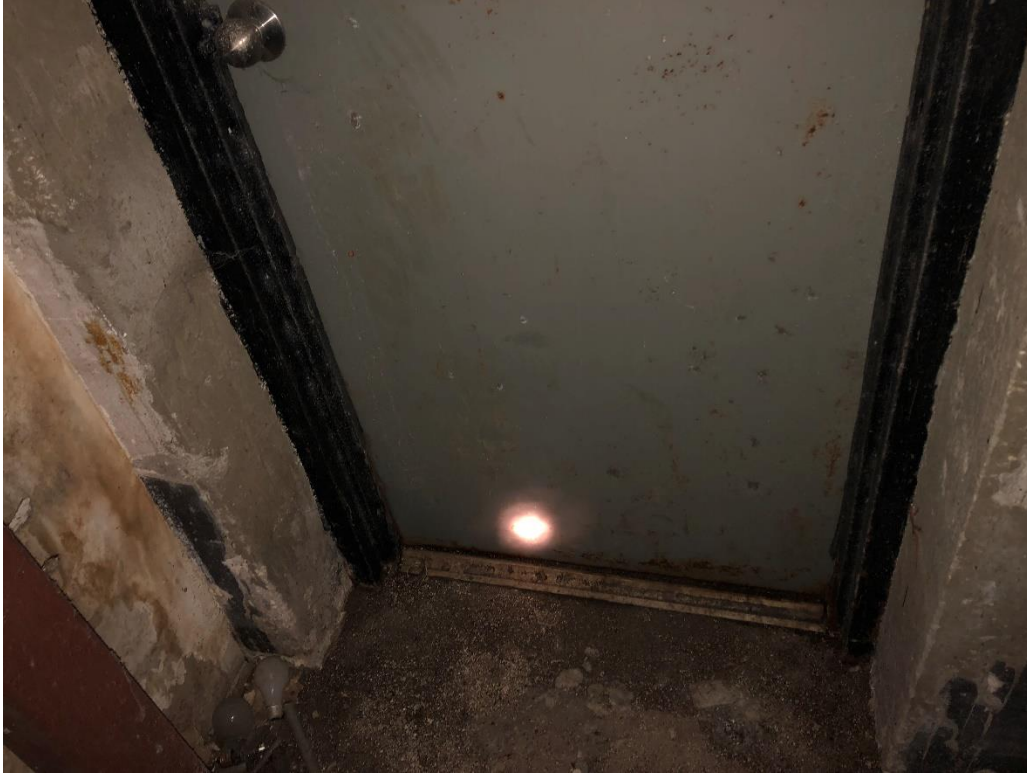
Photograph No. 77 – Lightly Corroded Exterior Door at Steel-framed Exit Staircase for Projection Room of West Cinema Theaters
