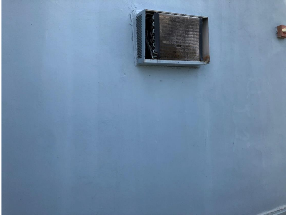
Photograph No. 17 – Uncovered Air Conditioning Unit in 2 nd floor Room at the South End of Building (Between east and West Theaters).
