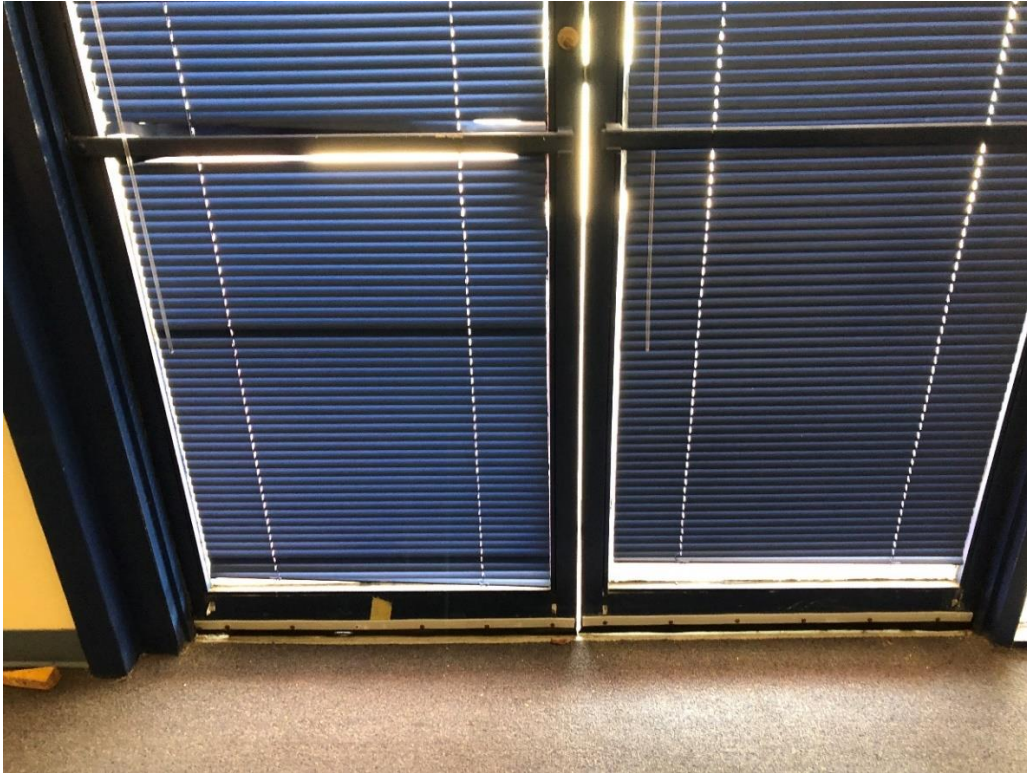
Photograph No. 75 – Considerable Gab between Pair of North Façade Doors
