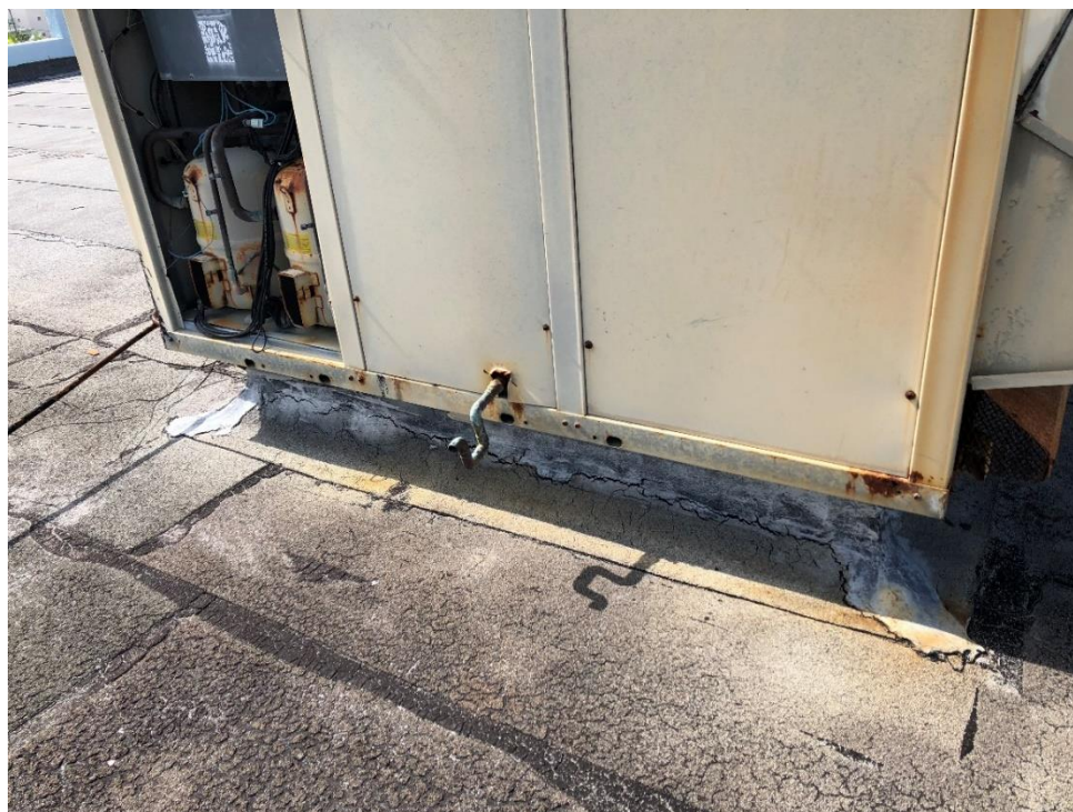
Photograph No. 63 – Package unit Unconnected to Roof Curb at Western Upper Roof
