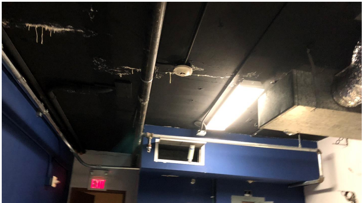
Photograph No. 28 – Efflorescence in Concrete Slab above Projection Room (East Side)
