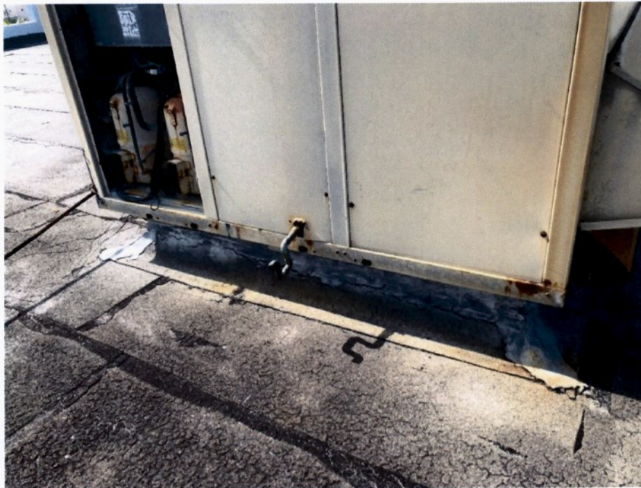
Photograph No. 63 – Package unit Unconnected to Roof Curb at Western Upper Roof
