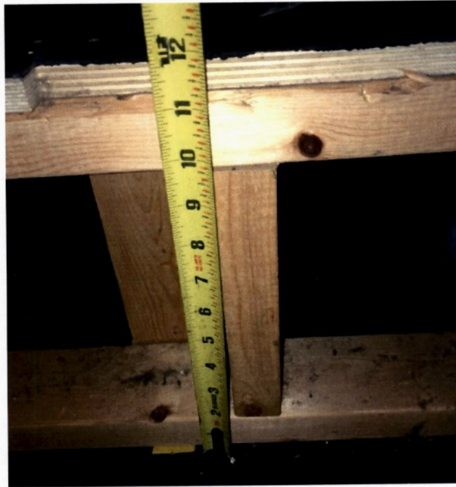
Photograph No. 9 – Built-up Wood Framing over Stage Platform for East Cinema Theater
