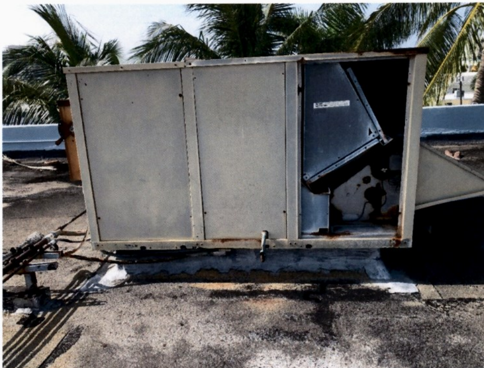
Photograph No. 64 – Package unit Unconnected to Roof Curb at Western Upper Roof
