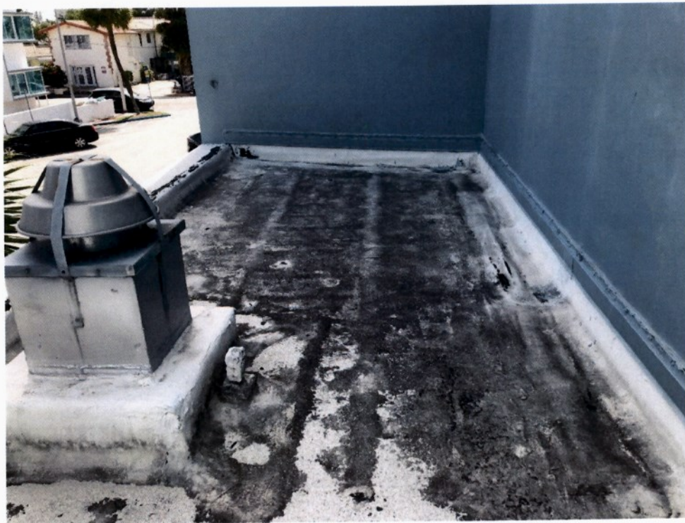
Photograph No. 24 – Deteriorated roofing at Lower Roof at the 2 nd Floor towards South Façade
