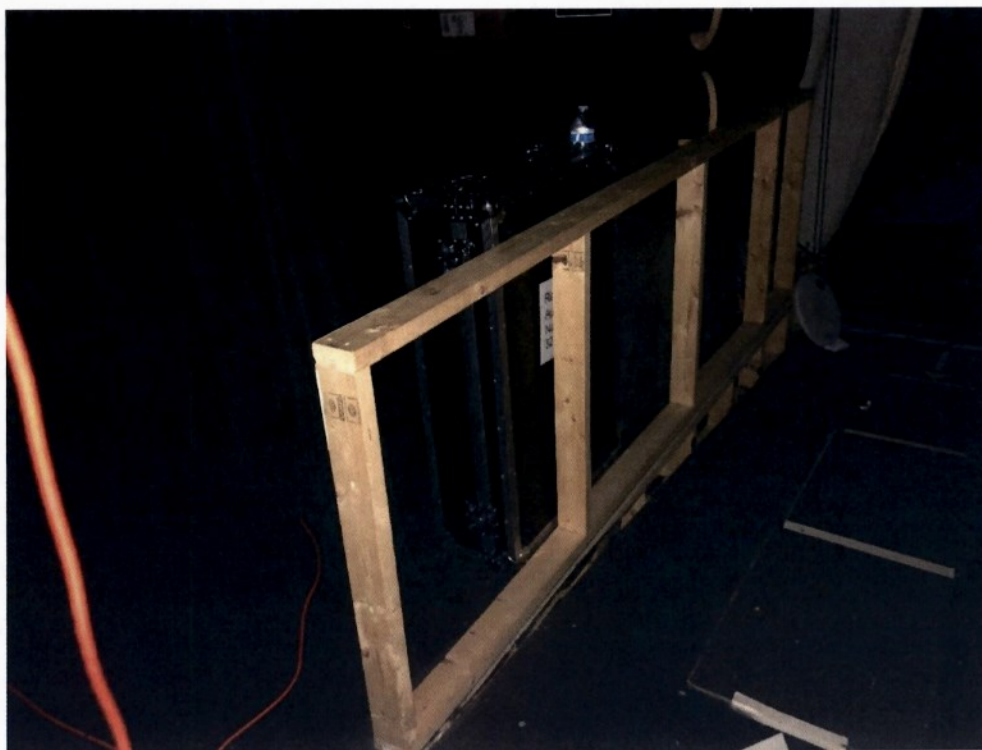
Photograph No. 37 – Loose Wooden Guardrail at East Cinema Theater
