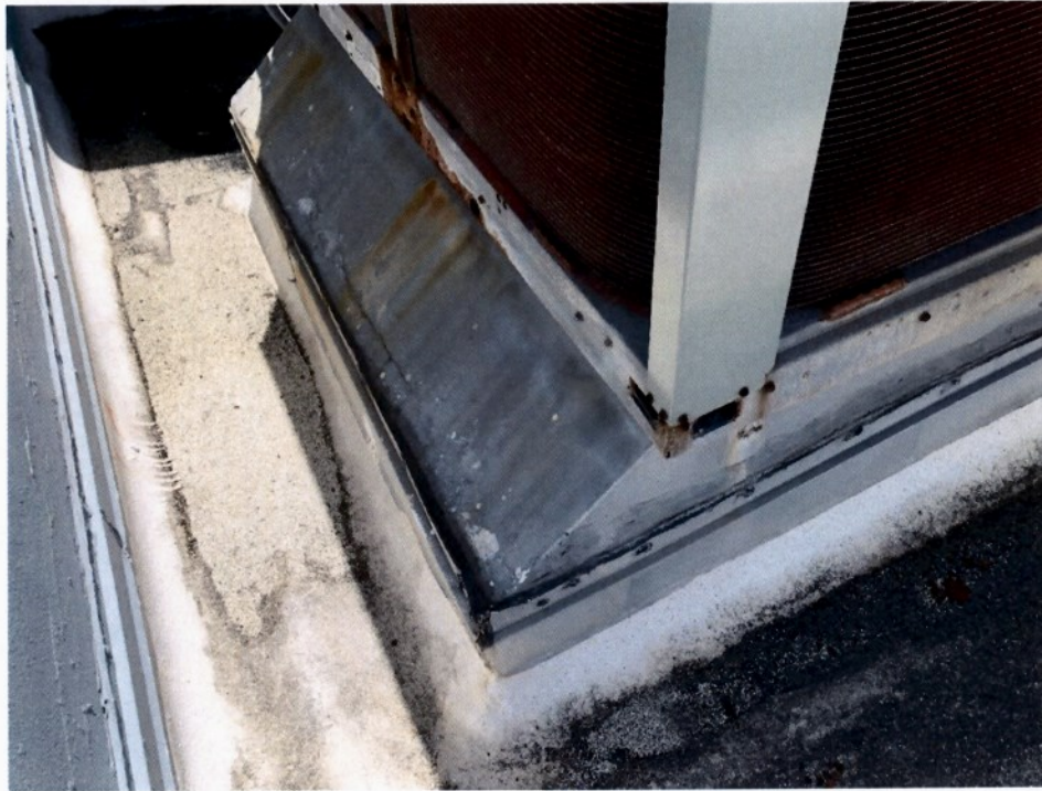
Photograph No. 65 – Package Unit Unconnected to Roof Curb at Low Roof between East and West Portions
