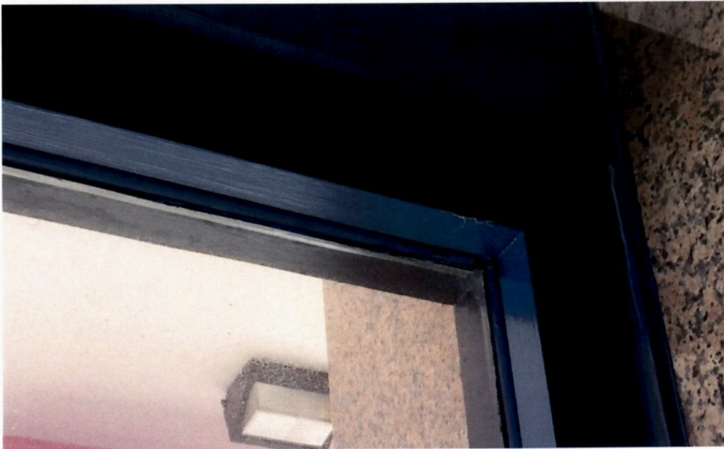
Photograph No. 74 – Missing Sealant at Corner of Fixed Window of North Façade
