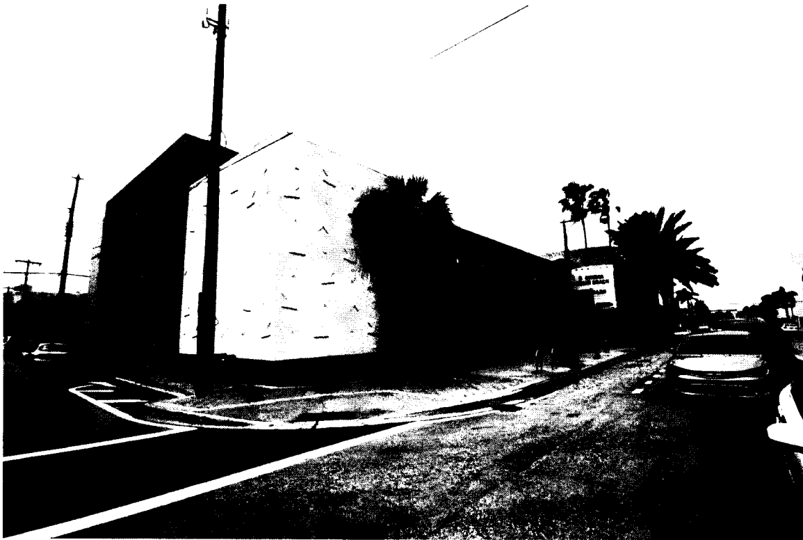
PHOTOGRAPH NO. 1 NORTHEAST CORNER OF BUILDING (NOTE STREET, SIDEWALK & DOOR ELEVATIONS. NOTE PROXIMITY OF STREET DRAINS)
