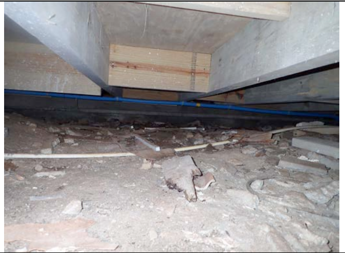
Photo 32 - Wood joist replacing concrete
