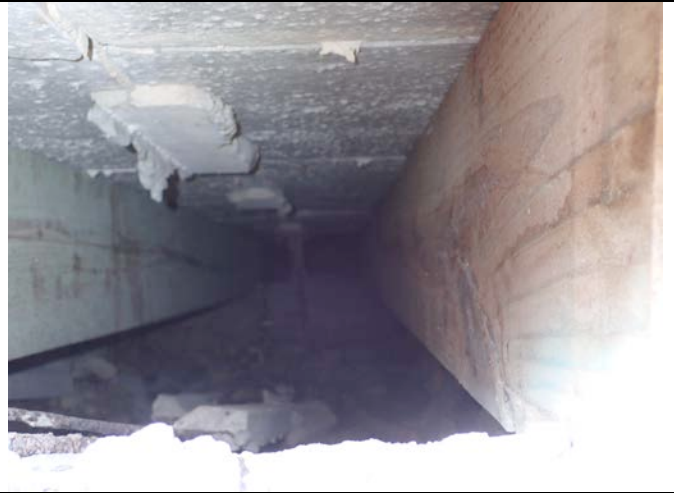
Photo 30 - Wood joist replacing concrete
