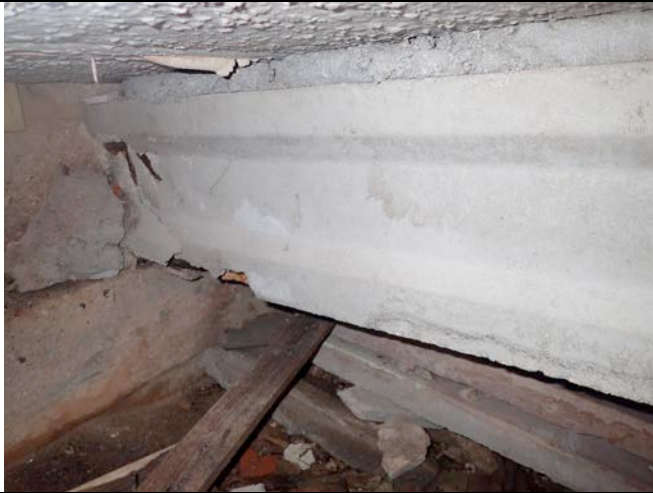
Photo 19 - Rebar corrosion and Concrete spalling of concrete joist system, and loss of bearing
