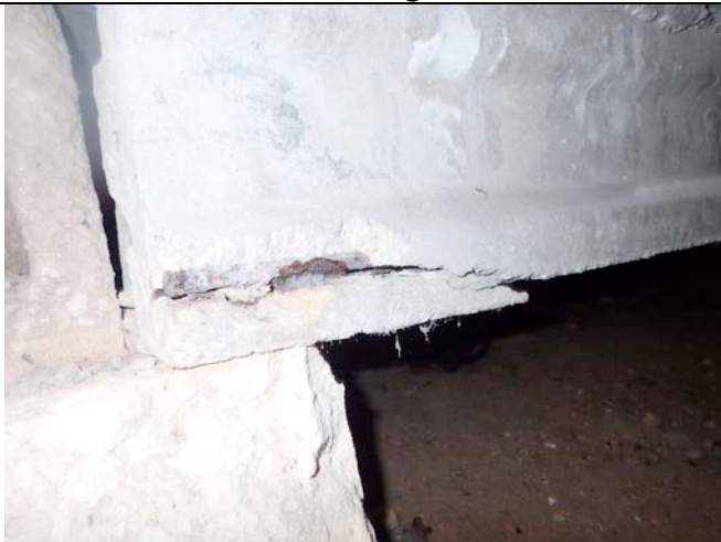
Photo 21 - Rebar corrosion and Concrete spalling of concrete joist system, and loss of bearing
