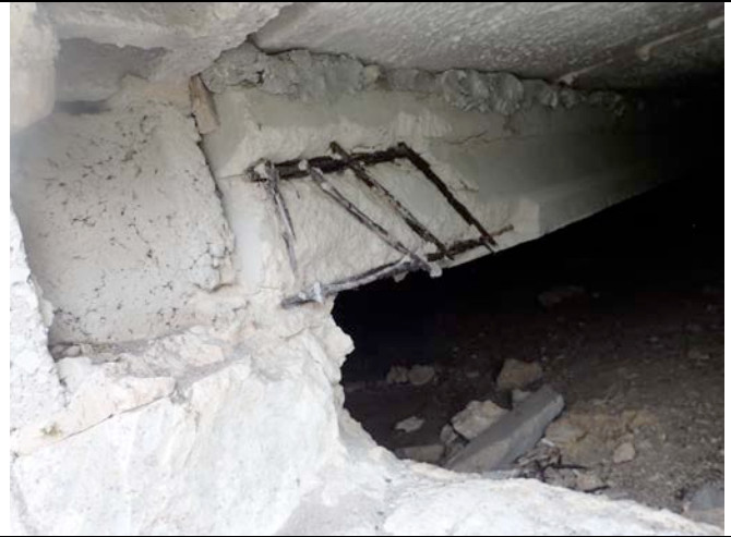
Photo 24 - Rebar corrosion and Concrete spalling of joist system, and loss of bearing
