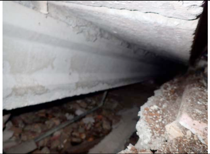
Photo 20 - concrete floor failure
