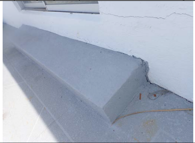
Photo 26 - cracking in exterior walls
