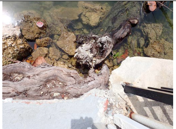
Photo 16 - Seawall deteriorated condition
