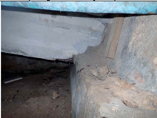
Photo 33 - Inadequate Previous repairs
