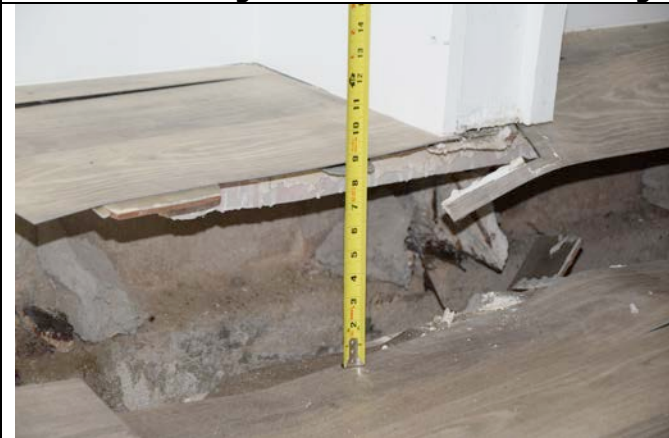
Photo 3 - failed joist system in 7935
