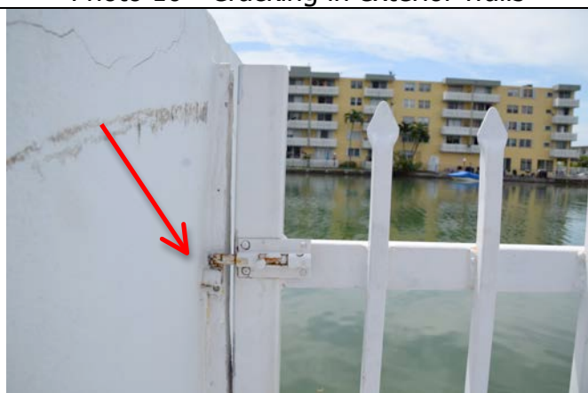
Photo 12 - settlement in wall, notice gate lock
