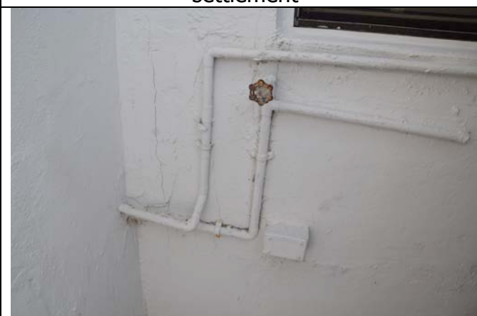
Photo 9 - Cracking in exterior walls
