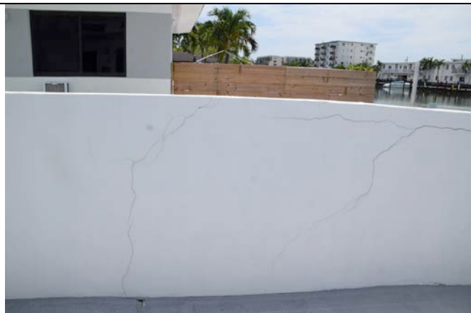
Photo 8 - Cracking of property wall due to settlement
