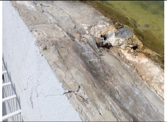
Photo 14 - Seawall deteriorated condition
