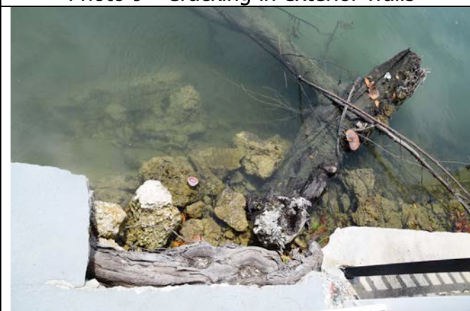
Photo 11 - Failed seawall
