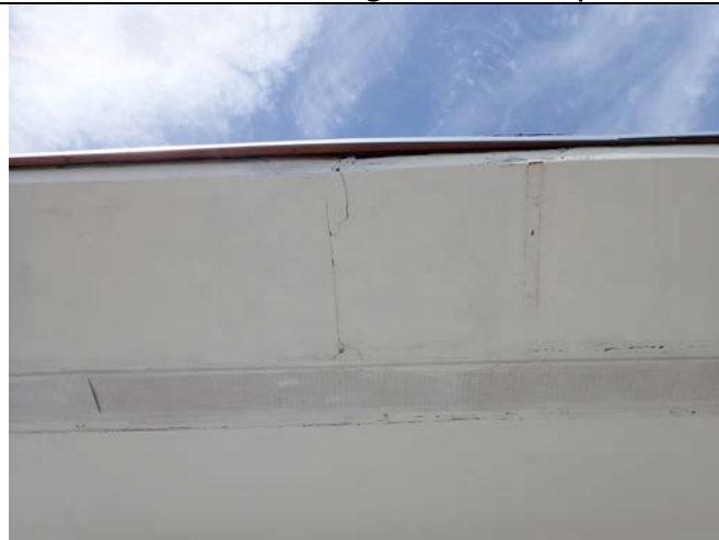
Photo 15 - Structure eave cracking
