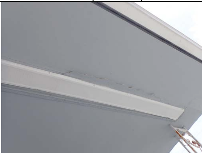
Photo 27 - cracking in soffits
