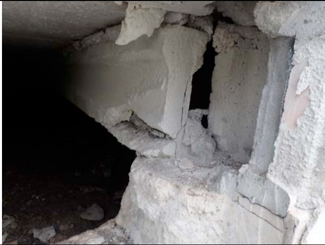
Photo 23 - Rebar corrosion and Concrete spalling of joist system, and loss of bearing
