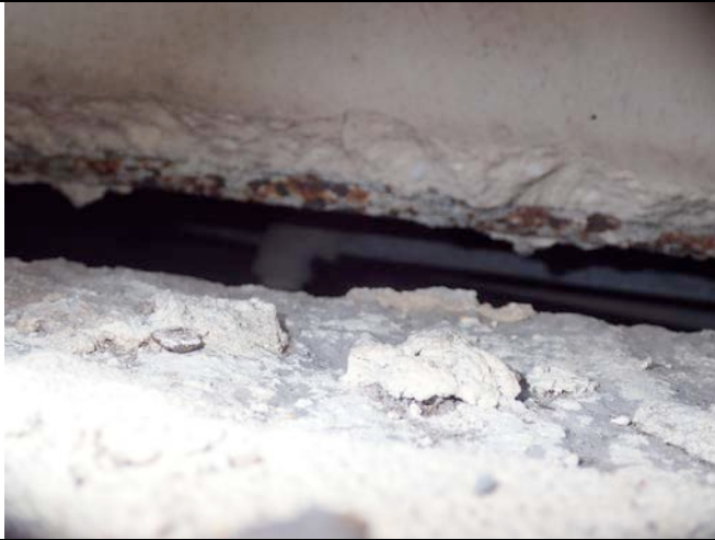
Photo 29 - Rebar corrosion and Concrete spalling of concrete joist system
