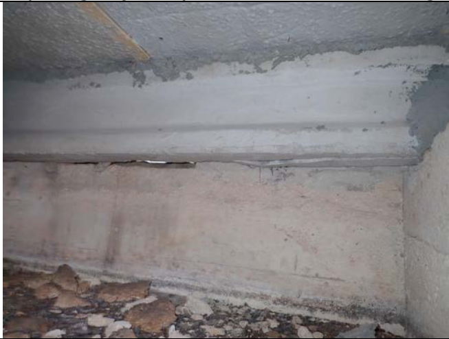
Photo 25 - previous repairs
