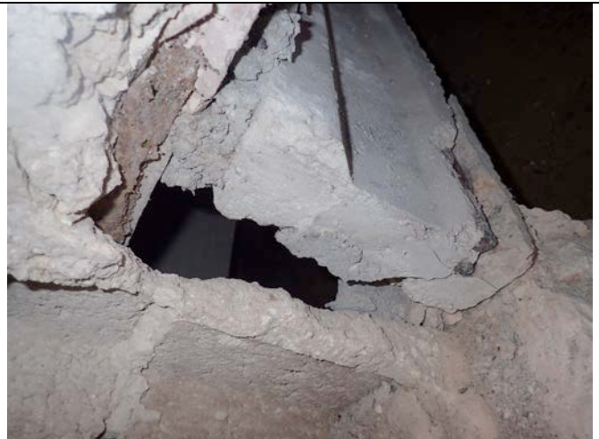
Photo 22 Rebar corrosion and Concrete spalling of concrete joist system, and loss of bearing
