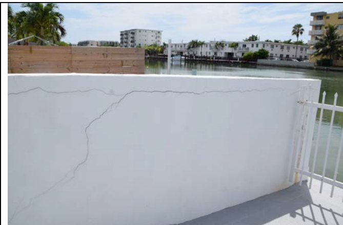
Photo 7 - Cracking of property wall due to settlement
