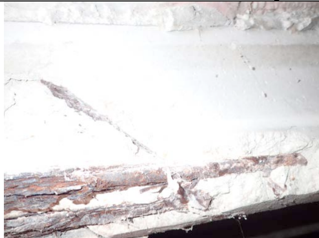
Photo 17 - Rebar corrosion and Concrete spalling of concrete joist system
