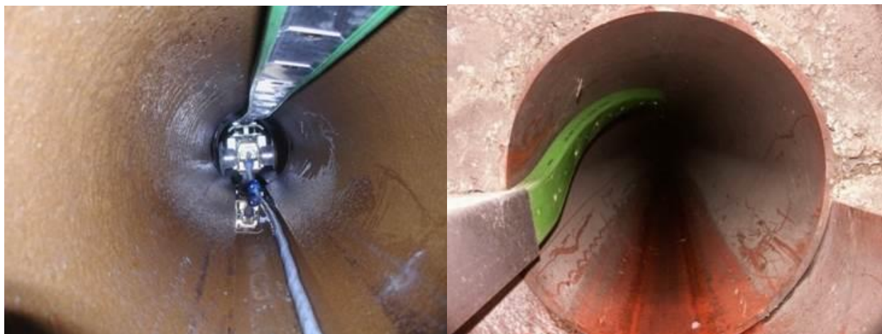
Figure 2-2: CableRunner technology installed in a non-accessible sewer of diameter less than 80 cm (30 in).
