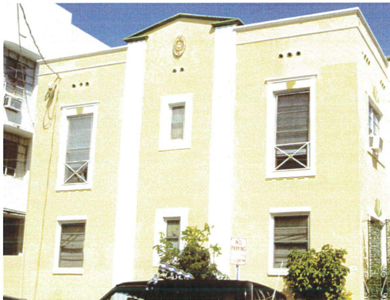
1999 Photograph, Sun King #1, South Elevation
