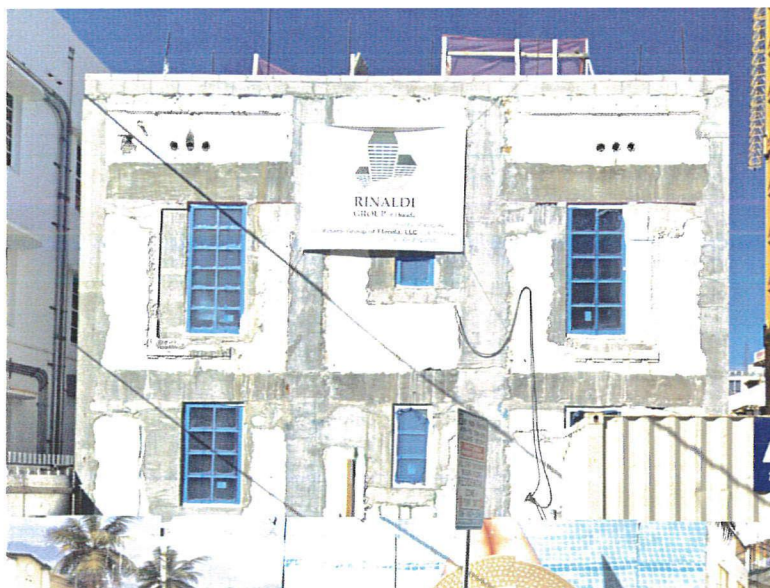
2008 Photograph, Sun King #1, South Elevation
