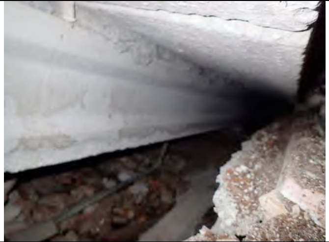
Photo 20 - concrete floor failure
