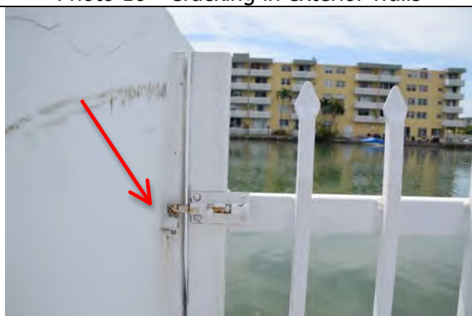
Photo 12 - settlement in wall, notice gate lock
