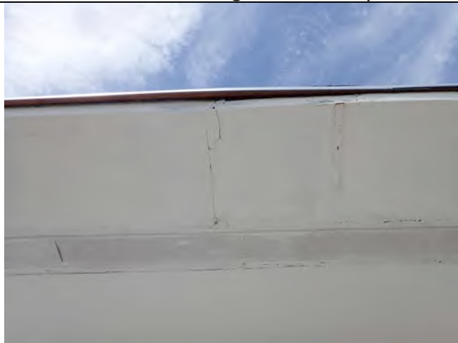
Photo 15 - Structure eave cracking
