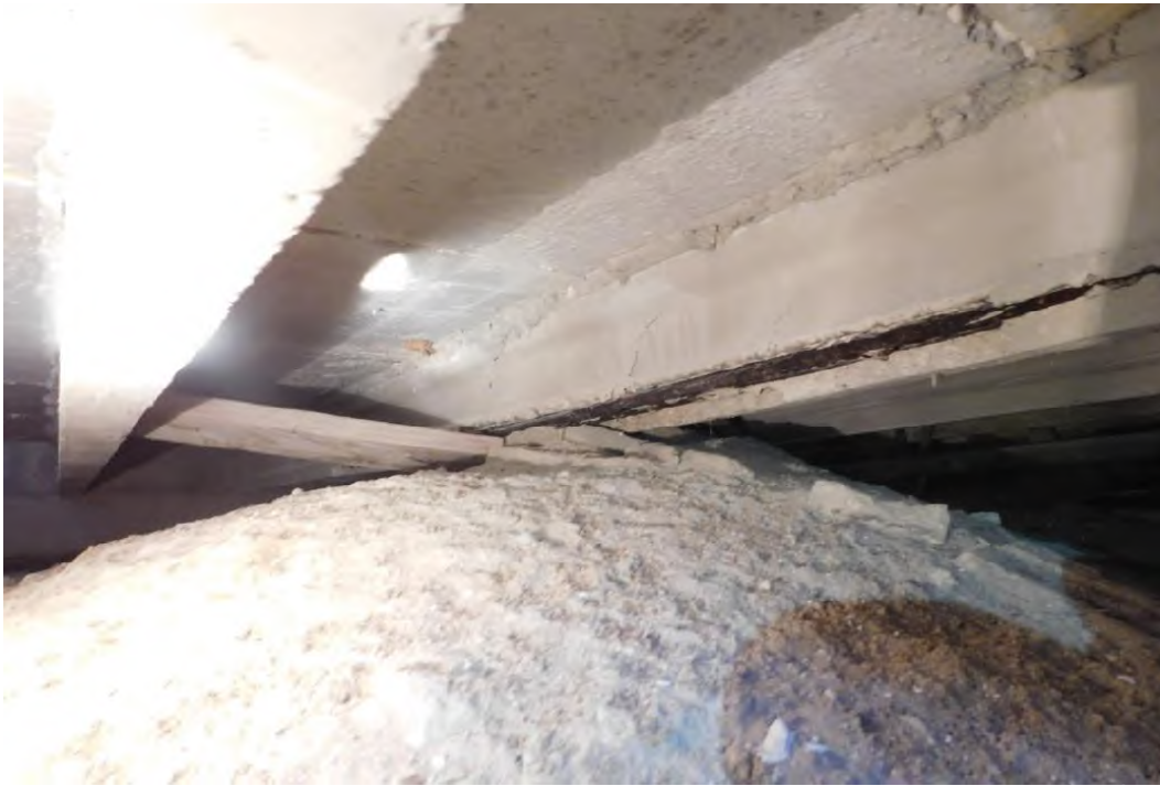
View of significant deterioration of floor joist at mid span section.
