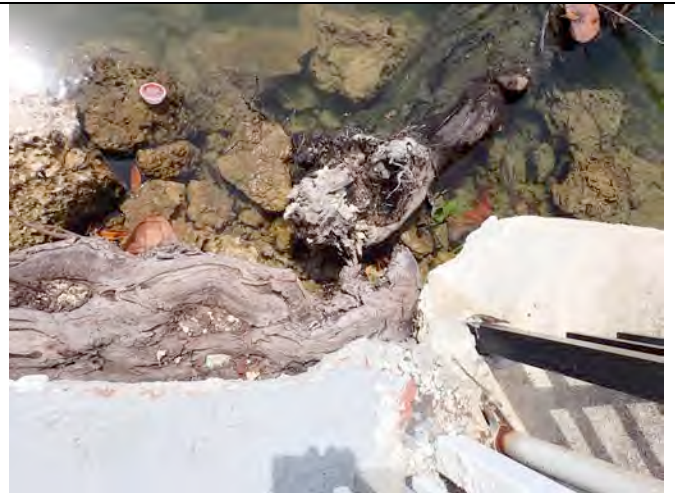
Photo 16 - Seawall deteriorated condition
