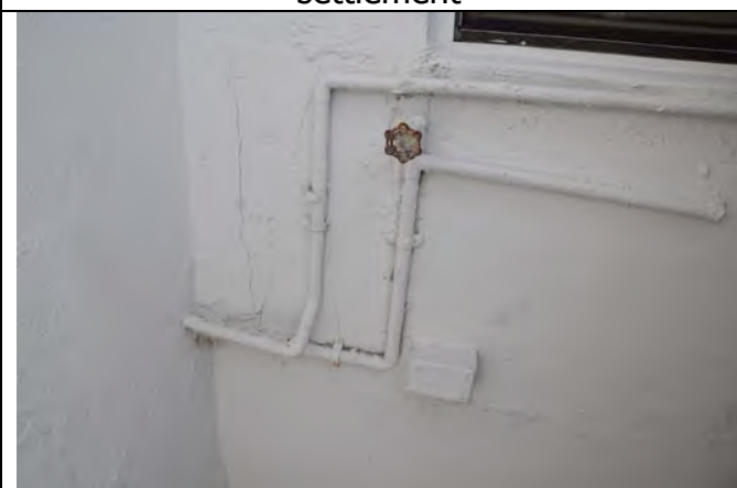
Photo 9 - Cracking in exterior walls
