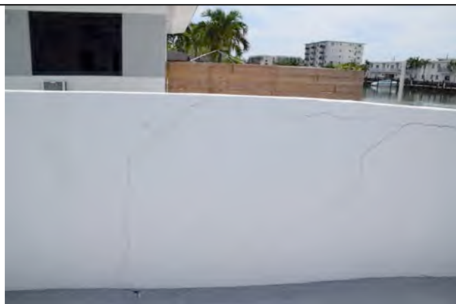
Photo 8 - Cracking of property wall due to settlement
