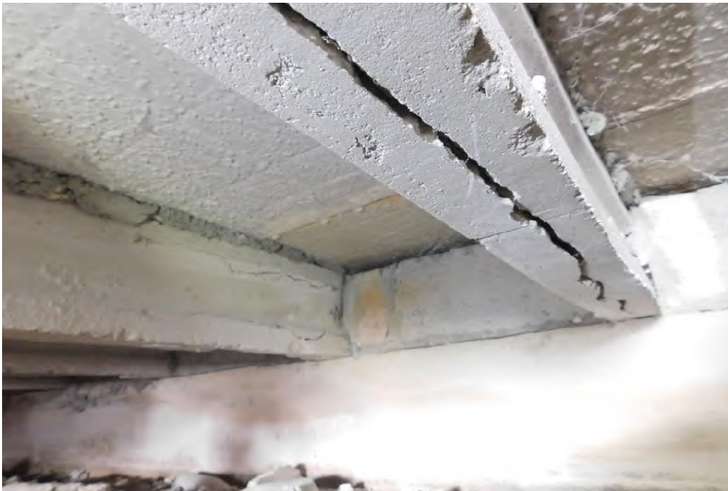
View of significant deterioration of floor joist at support section.
