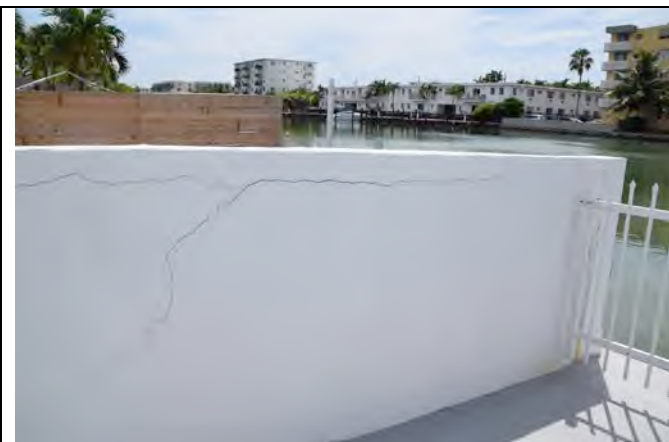
Photo 7 - Cracking of property wall due to settlement
