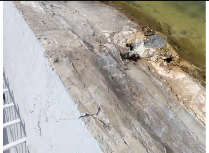
Photo 14 - Seawall deteriorated condition
