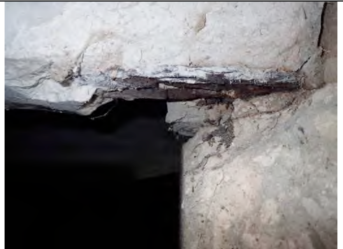
Photo 18 - Rebar corrosion and Concrete spalling of concrete joist system, and loss of bearing
