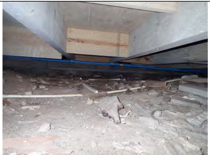
Photo 32 - Wood joist replacing concrete
