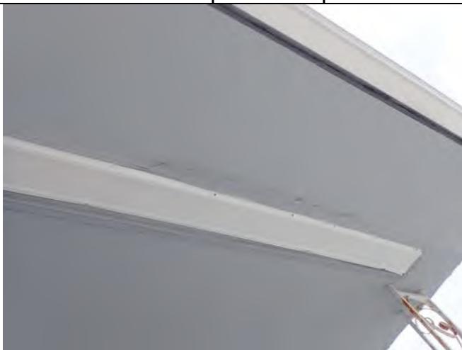
Photo 27 - cracking in soffits
