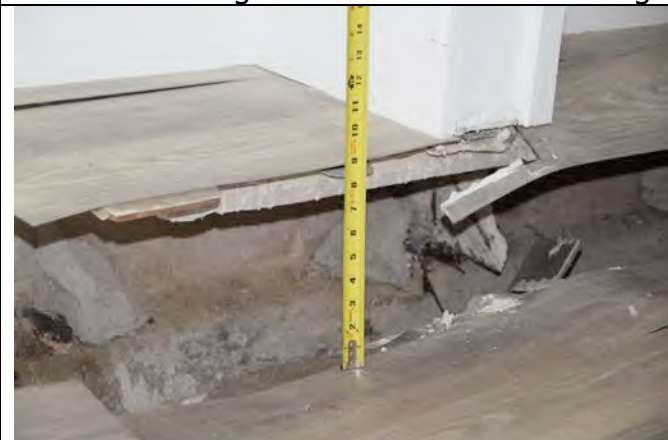
Photo 3 - failed joist system in 7935
