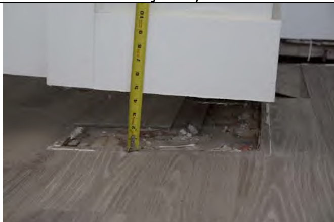
Photo 4 - failed joist system in 7935
