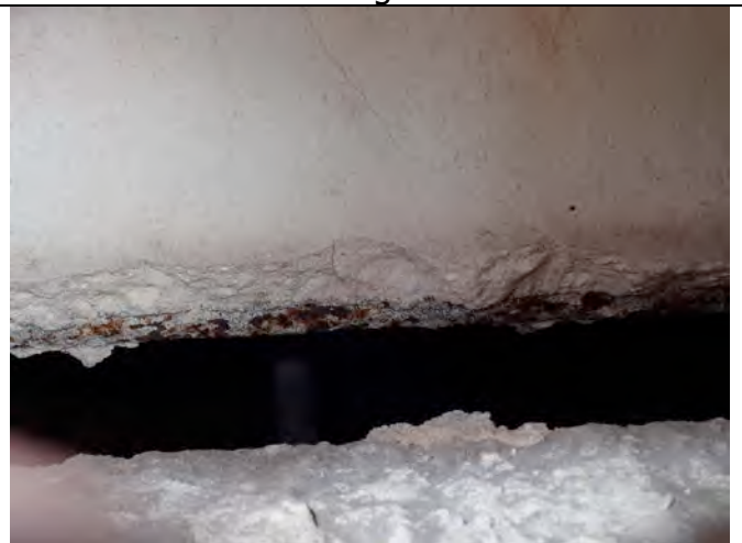
Photo 28 - Rebar corrosion and Concrete spalling of concrete joist system, and loss of bearing
