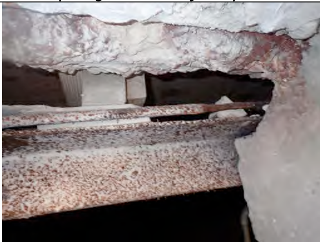
Photo 31 - Rebar corrosion and Concrete spalling of concrete joist system
