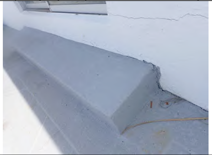
Photo 26 - cracking in exterior walls
