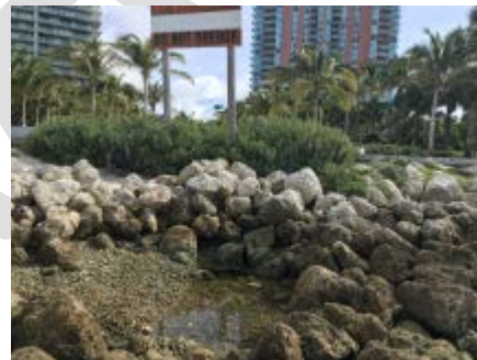
Figure 5: Rip-rap energy dissipation near outfall
