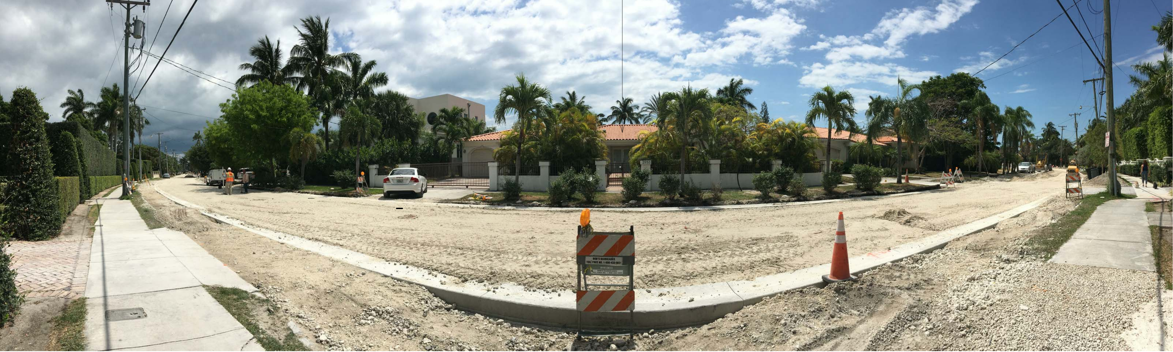
WEST SIDE OF N. BAY ROAD 04-25-2016
