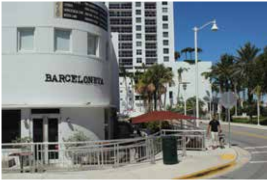
Barceloneta, a restaurant in Sunset Harbour, is surrounded by elevated streets and now has patio seating at the original street elevation.
