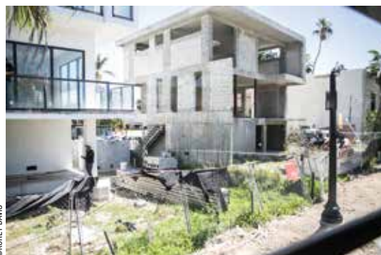
New construction in Miami Beach is designed with living space well above ground, allowing the ground floor to flood.
