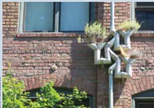
Environmental sculptor Buster Simpson designed several pieces for Vine Street, including this feature on a building facade, which helps filter rain and stormwater runoff.
