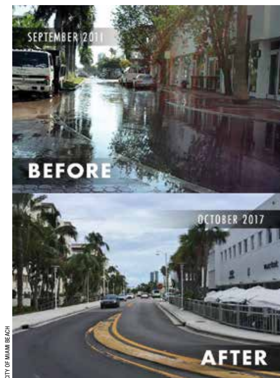
The improvements in Sunset Harbour are an example of one of Miami Beach's many stormwater successes.
