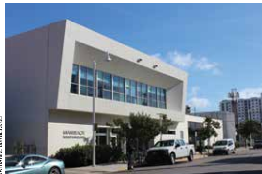
The Miami Beach Property Management Facility, constructed in 2009, was required to be certified LEED Gold.
