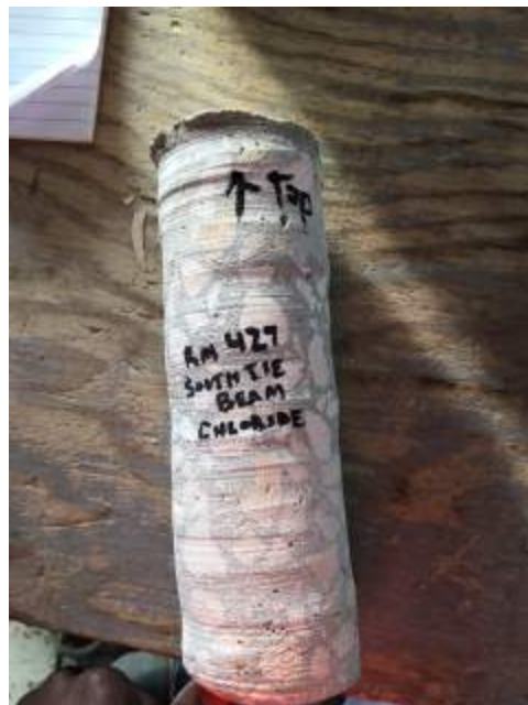
Figure 12: Core Sample – Chloride Test
