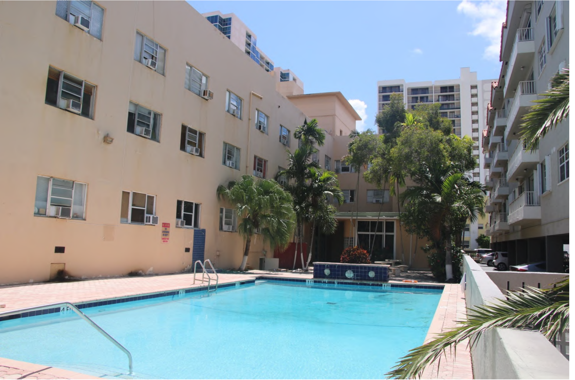
REAR (WEST) POOL AREA LOOKING EAST
