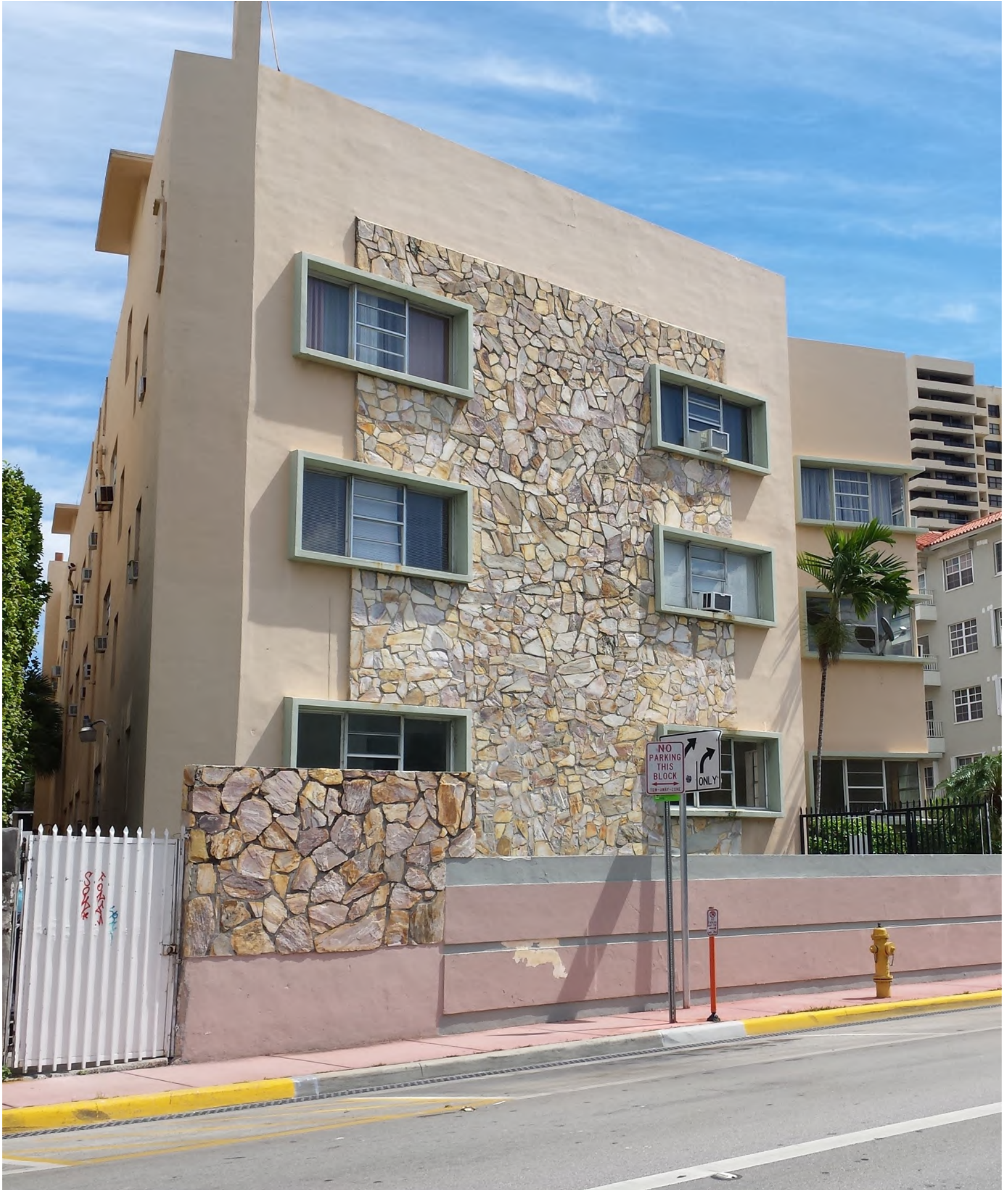
WEST (REAR) ELEVATION ALONG INDIAN CREEK DRIVE - PHOTOGRAPH 2016
