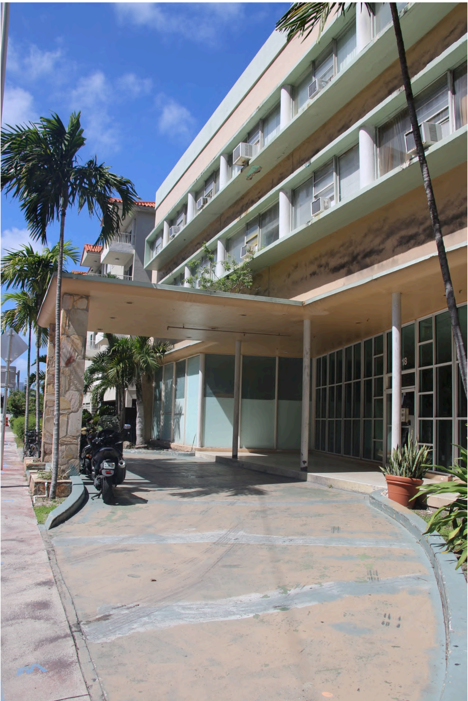
EAST (FRONT) ELEVATION LOOKING SOUTH
