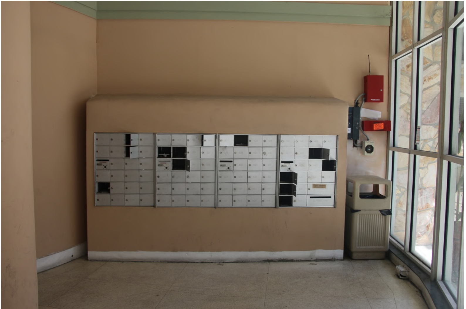
ABOVE: VIEW TOWARDS NON-HISTORIC MAILBOX ENCLOSURE AT LOBBY
