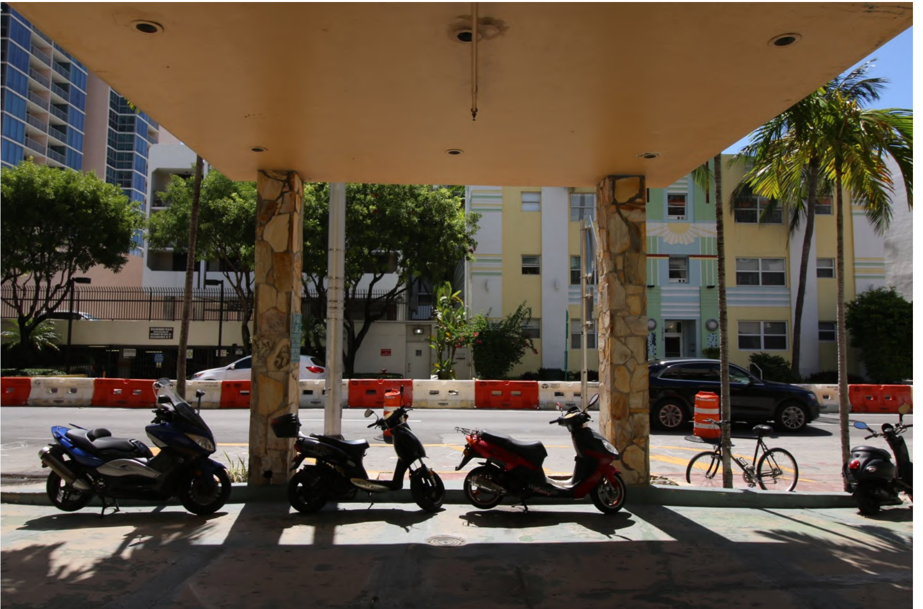
VIEW LOOKING WEST FROM LOBBY TO COLLINS AVENUE.
