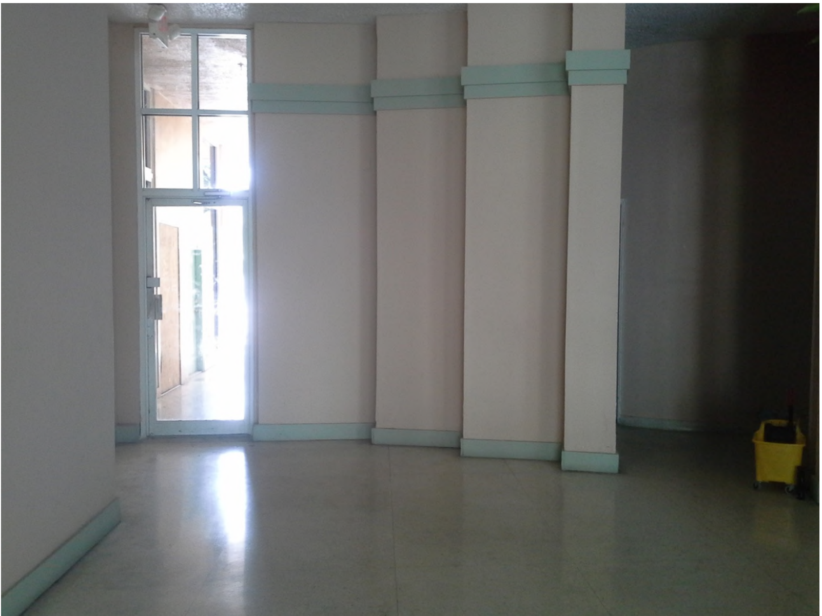
BELOW: HISTORIC SERRATED WALLS ADJACENT TO POOL ENTRANCE AT LOBBY
