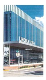
The white acrylic face of the letters will allow for the internal LED illumination to display and light the sign. The signage is proposed with 3'-0" high letters that span 19'-3" in length, for a total sign area of 58 SF. It is important to note that, at the recommendation of staff, the proposed 3'-0" high lettering matches in size and scale the approved 'Marshalls' building ID sign installed at the top of the building.
