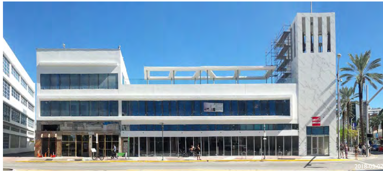
19.VIEW TOWARDS EAST FROM CORNER OF LINCOLN ROAD AND WASHINGTON AVENUE
