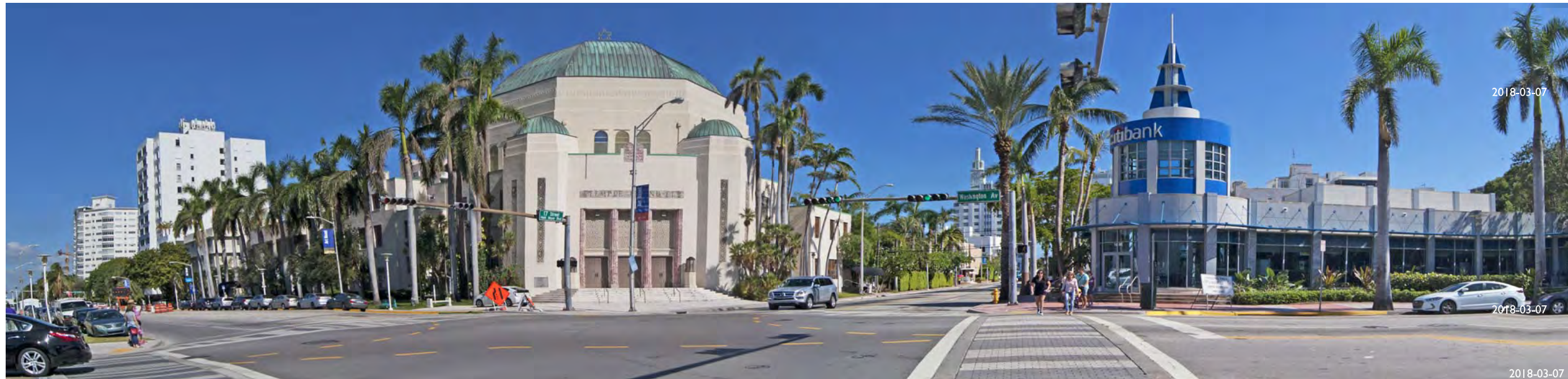
2018-03-07 12. INTERSECTION OF WASHINGTON AVENUE AND 17H STREET, VIEW OF PROPERTY
