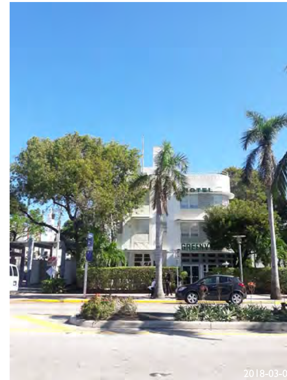
16.VIEW TOWARDS EAST OF GREENVIEW HOTEL
