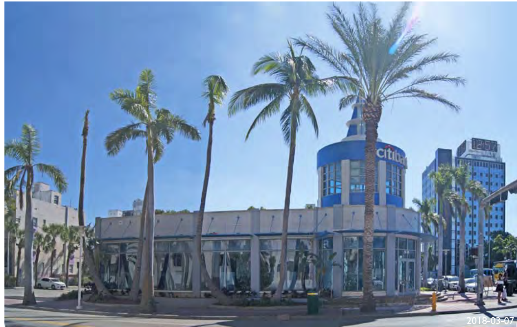
2018-03-07 3. SITE FACING 17TH STREET
