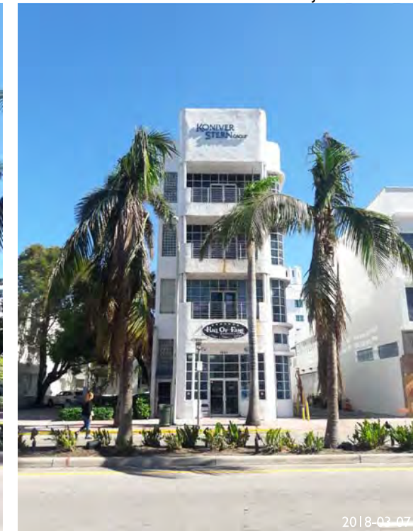
15.VIEW TOWARDS EAST OF OFFICE BUILDING
