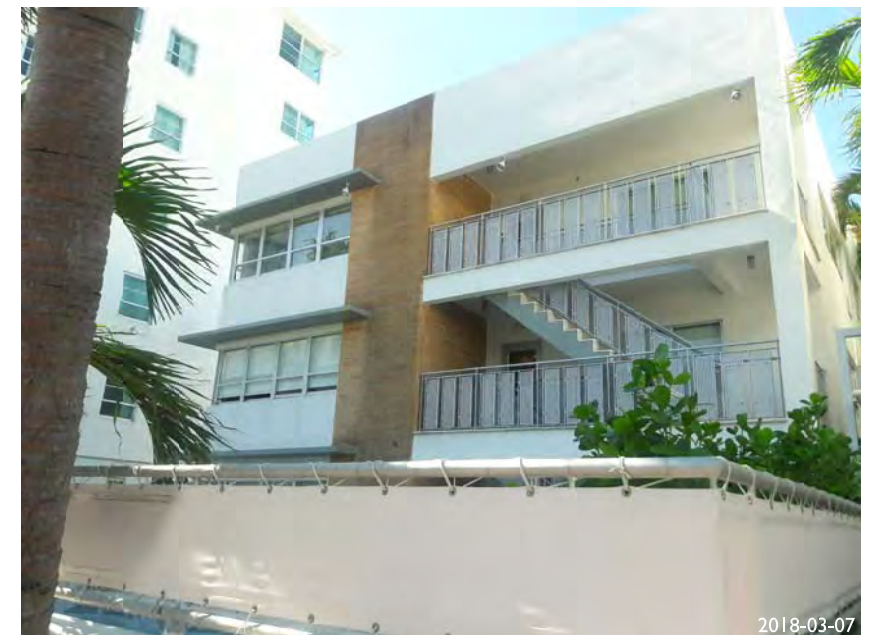
2018-03-07 9. VIEW OF CREST HOTEL AND SUITES FACING WEST
