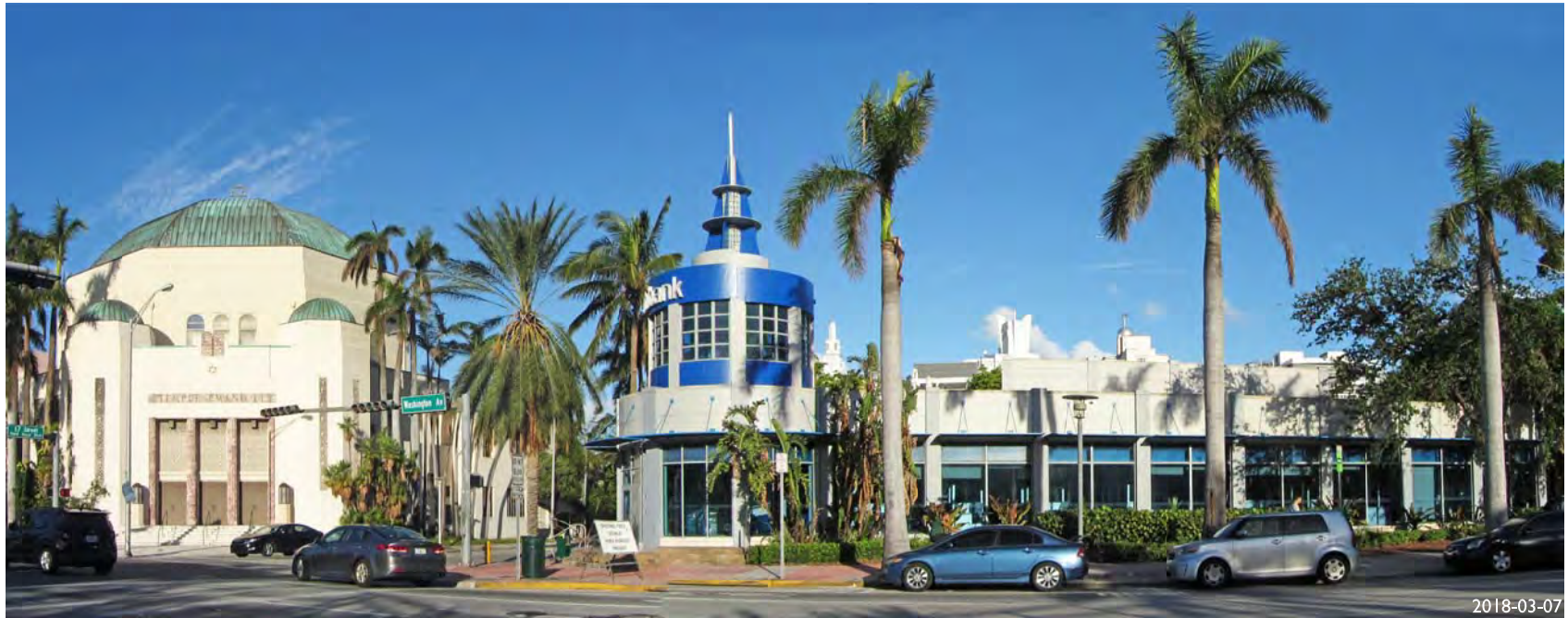
2018-03-07 2. SITE FACING WASHINGTON AVENUE
