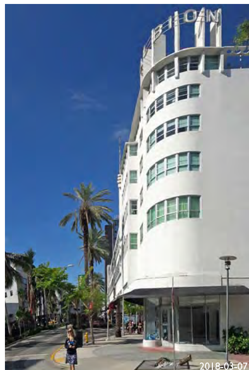
2018-03-07 11. VIEW OF THE ALBION HOTEL AND LINCOLN ROAD FACING WEST
