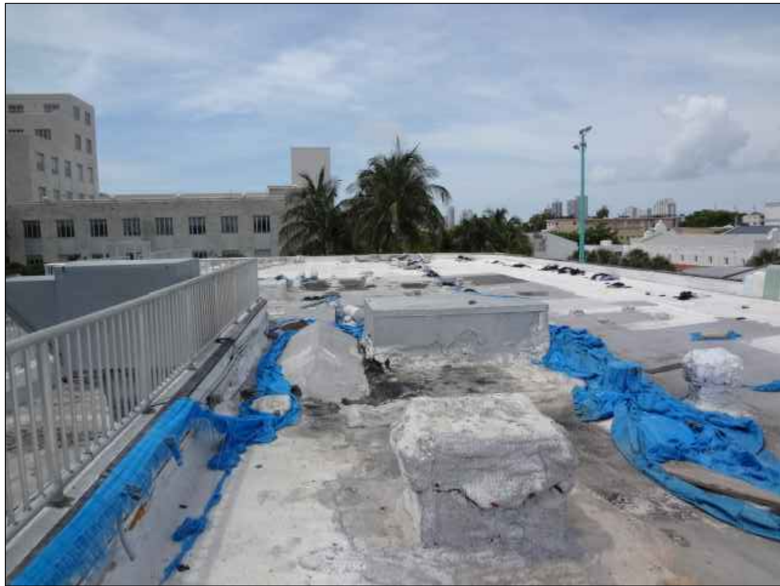
SUBJECT PROPERTY — ROOF LEVEL LOOKING NORTHWEST PICTURE 14
