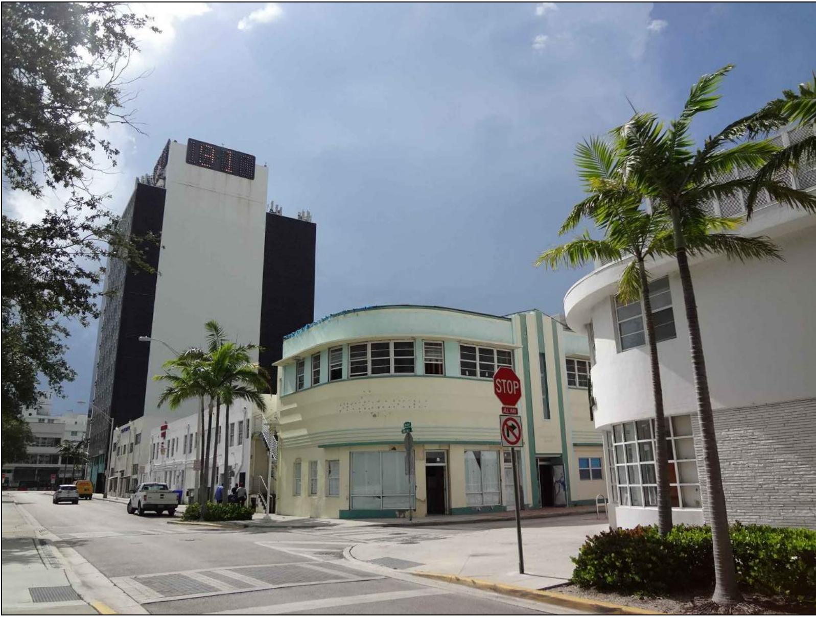
SUBJECT PROPERTY NORTH WEST ELEVATION PICTURE 1
