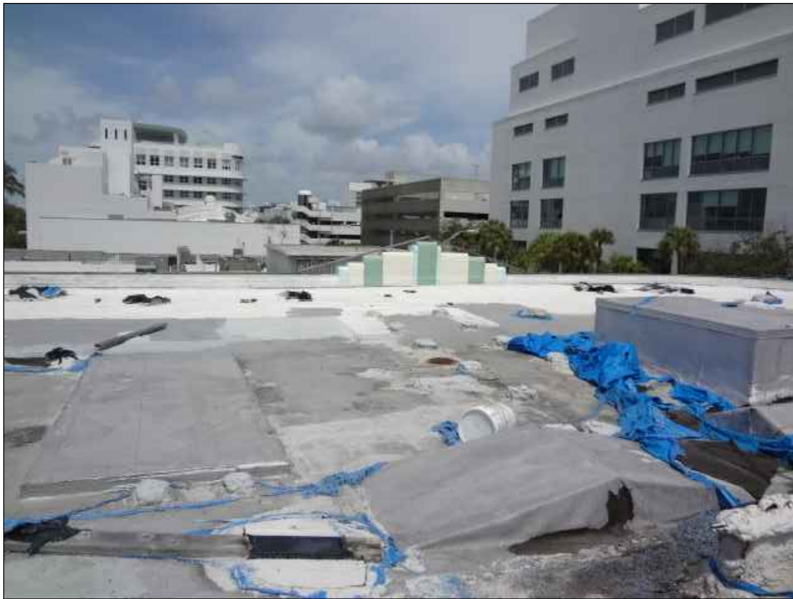
SUBJECT PROPERTY — ROOF LEVEL LOOKING SOUTH PICTURE 13
