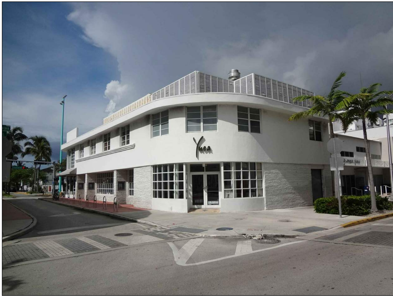
FROM SUBJECT PROPERTY LOOKING SOUTH EAST PICTURE 10
