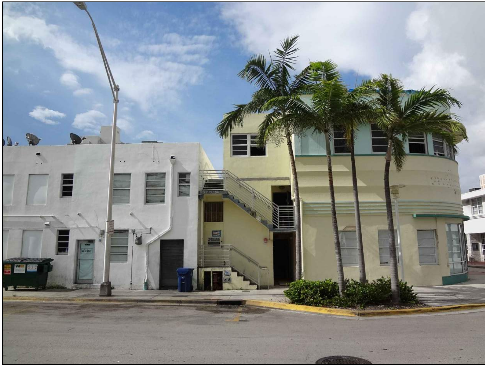
SUBJECT PROPERTY NORTH EAST ELEVATION PICTURE 3
