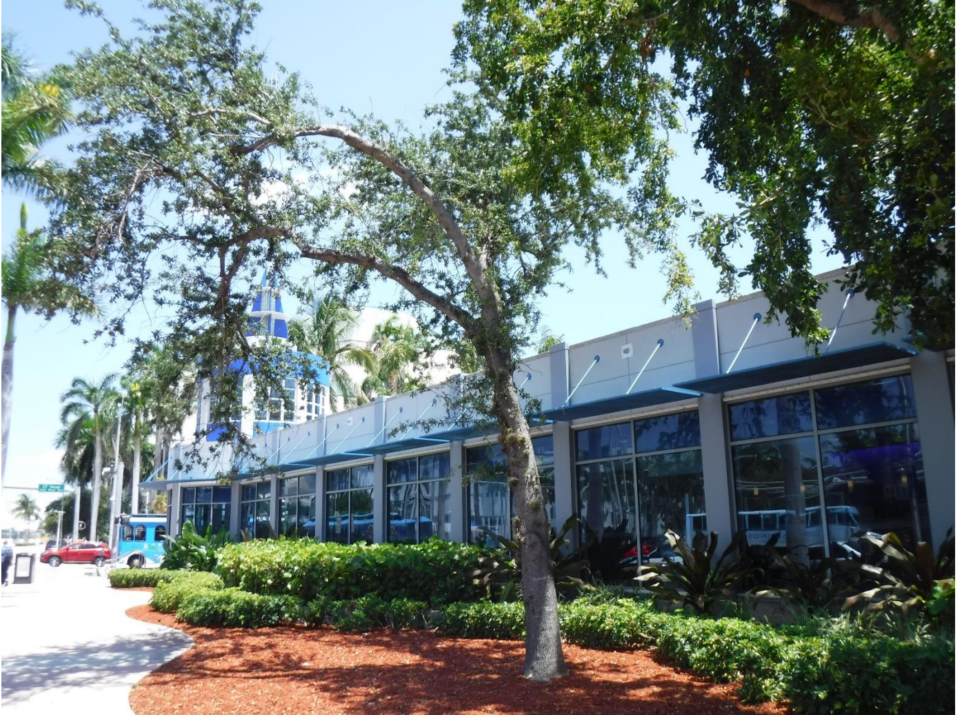
View looking North East
