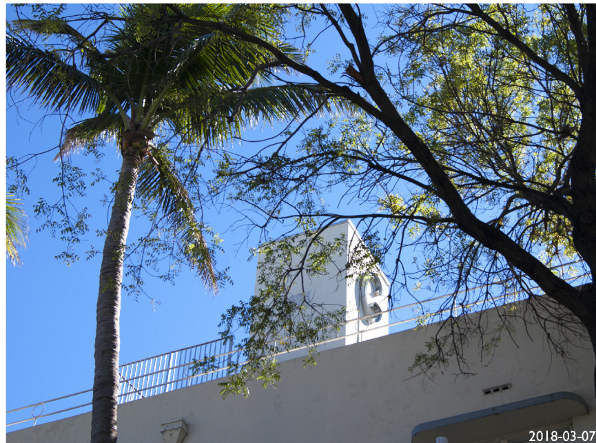
2018-03-07 10. VIEW TOWARDS NEIGHBORING STRUCTURES
