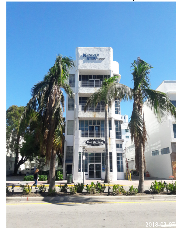
15.VIEW TOWARDS EAST OF OFFICE BUILDING
