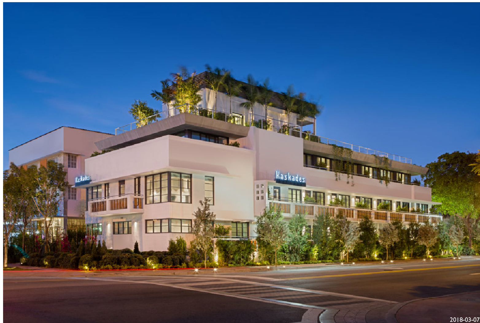
2. PHOTO OF THE EXISTING KASKADES HOTEL
