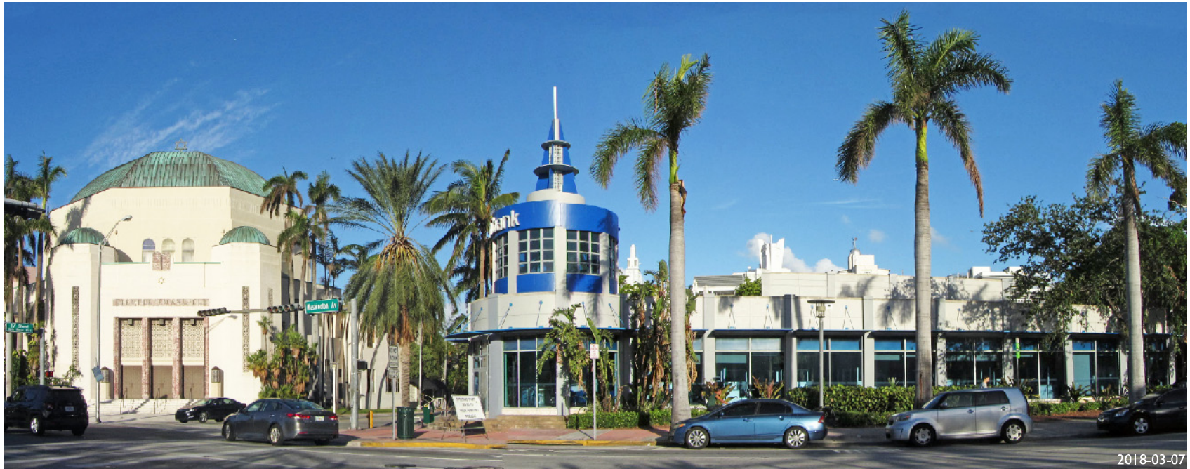
2018-03-07 2. SITE FACING WASHINGTON AVENUE
