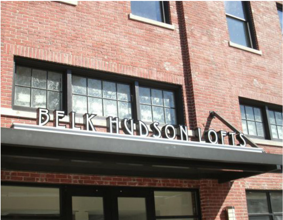
CANOPY-MOUNTED CHANNEL LETTER EXAMPLE (TOP MOUNTED)
