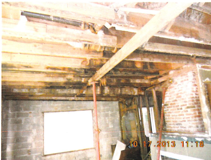
2nd. Floor framing- deterioration of existing Wood joists due to fire damage and water damage.
