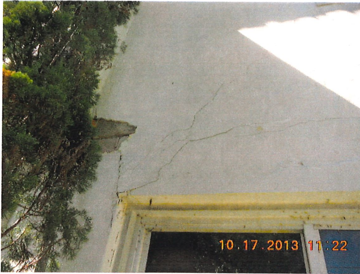
Front facade- evidence of structural crack indicating settlement
