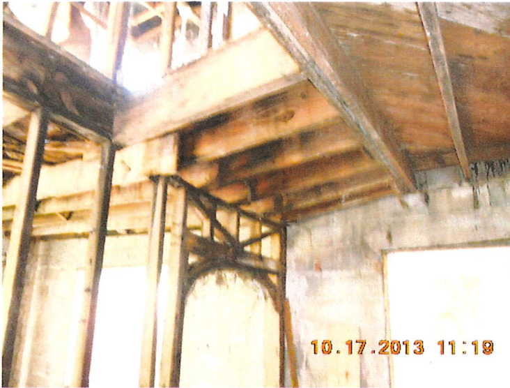
2nd. Floor framing- deterioration of existing Wood joists and buckling of bearing partition
