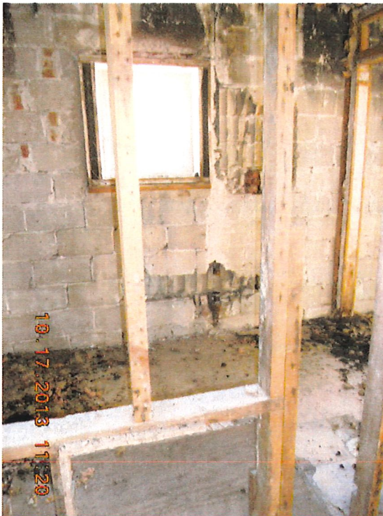
Ground floor masonry Wall- severe cut-out of existing masonry and no vertical reinforcing.
