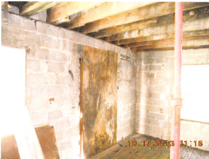
1st. Floor- no intermediate beam or tie-beam
