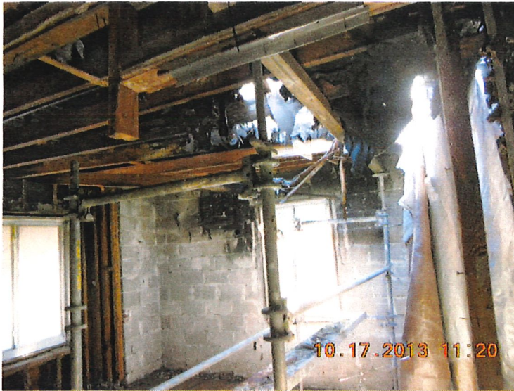
2nd. Floor- Roof truss damaged by fire.
