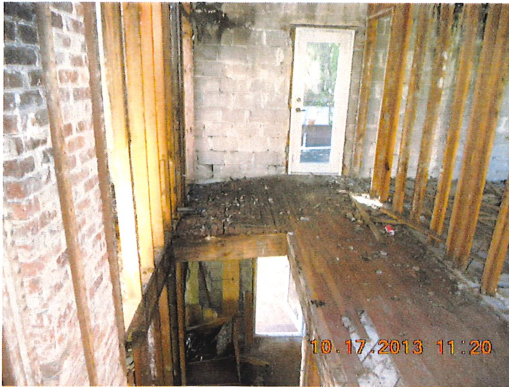
2nd. Floor framing- damaged by fire
