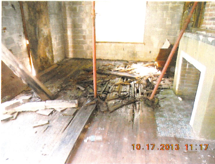
Ground floor damage to framing
