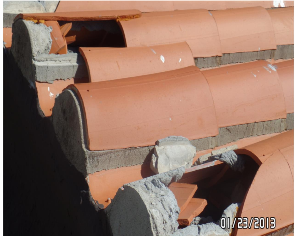
18. BROKEN ROOF TILES FROM EITHER FLYING DEBRIS OR WIND UPLIFT
