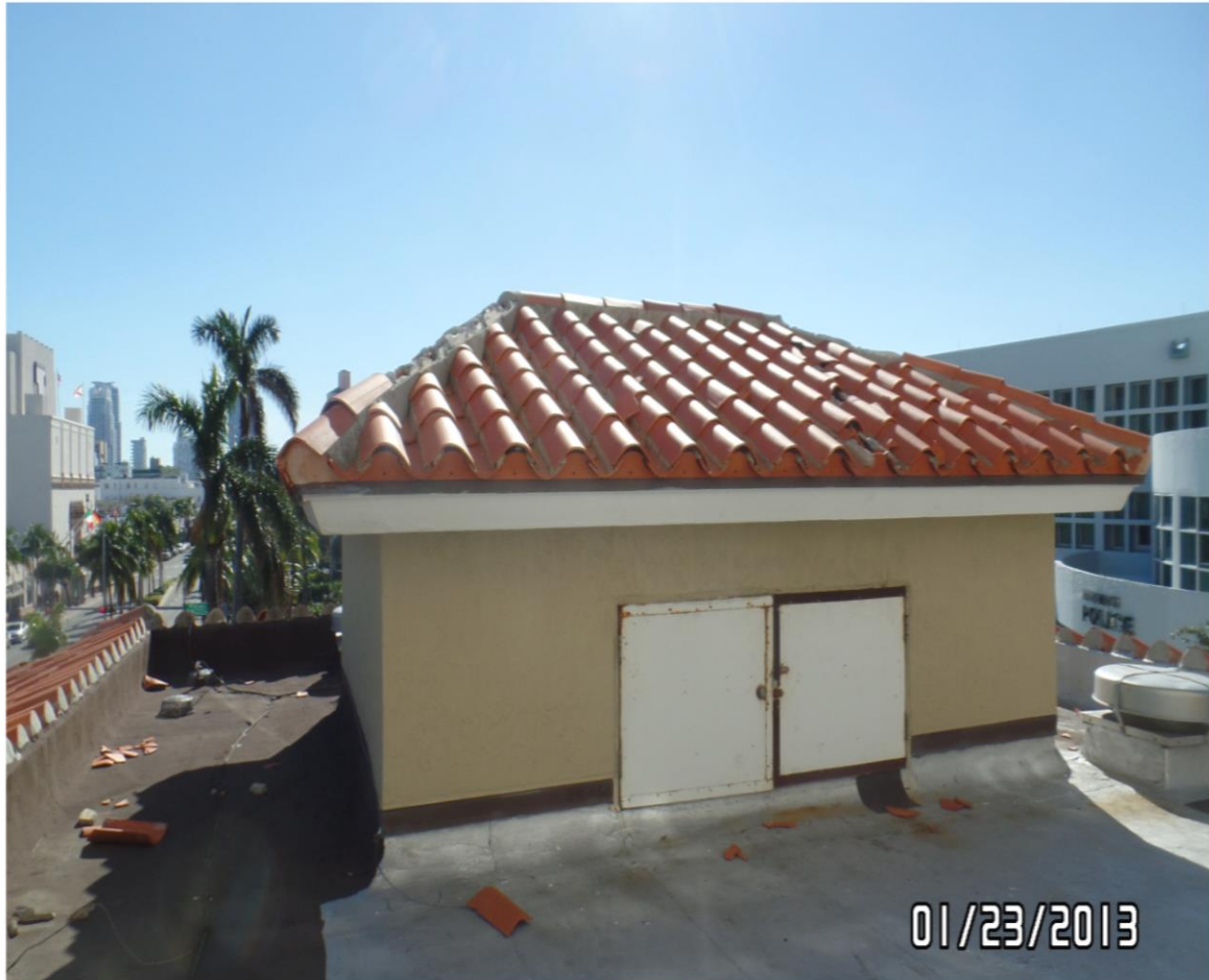
9. MISSING RIDGE TILES ON CENTER PENTHOUSE OVER COURTROOM 2-1
