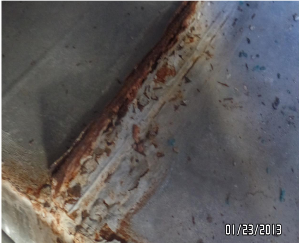
23. RUSTED METAL DUCTWORK IN EQUIPMENT ROOM
