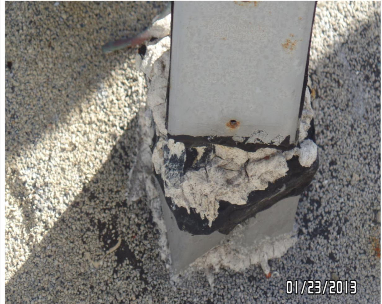
34. ELECTRICAL BOX SURROUNDED BY A FAILING PITCH PAN
