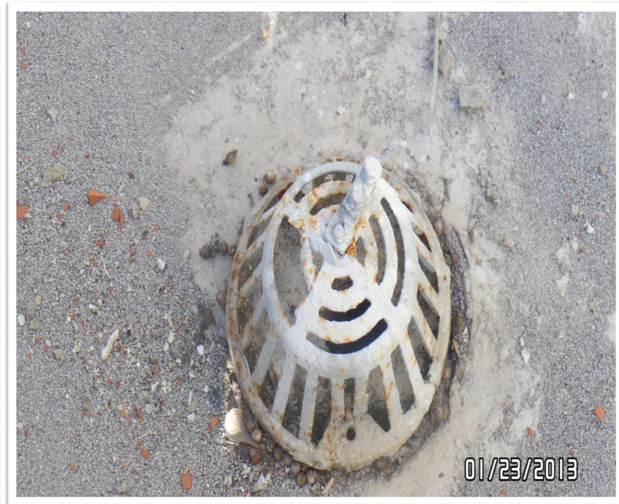
36. TYPICAL INTERNAL DRAIN
