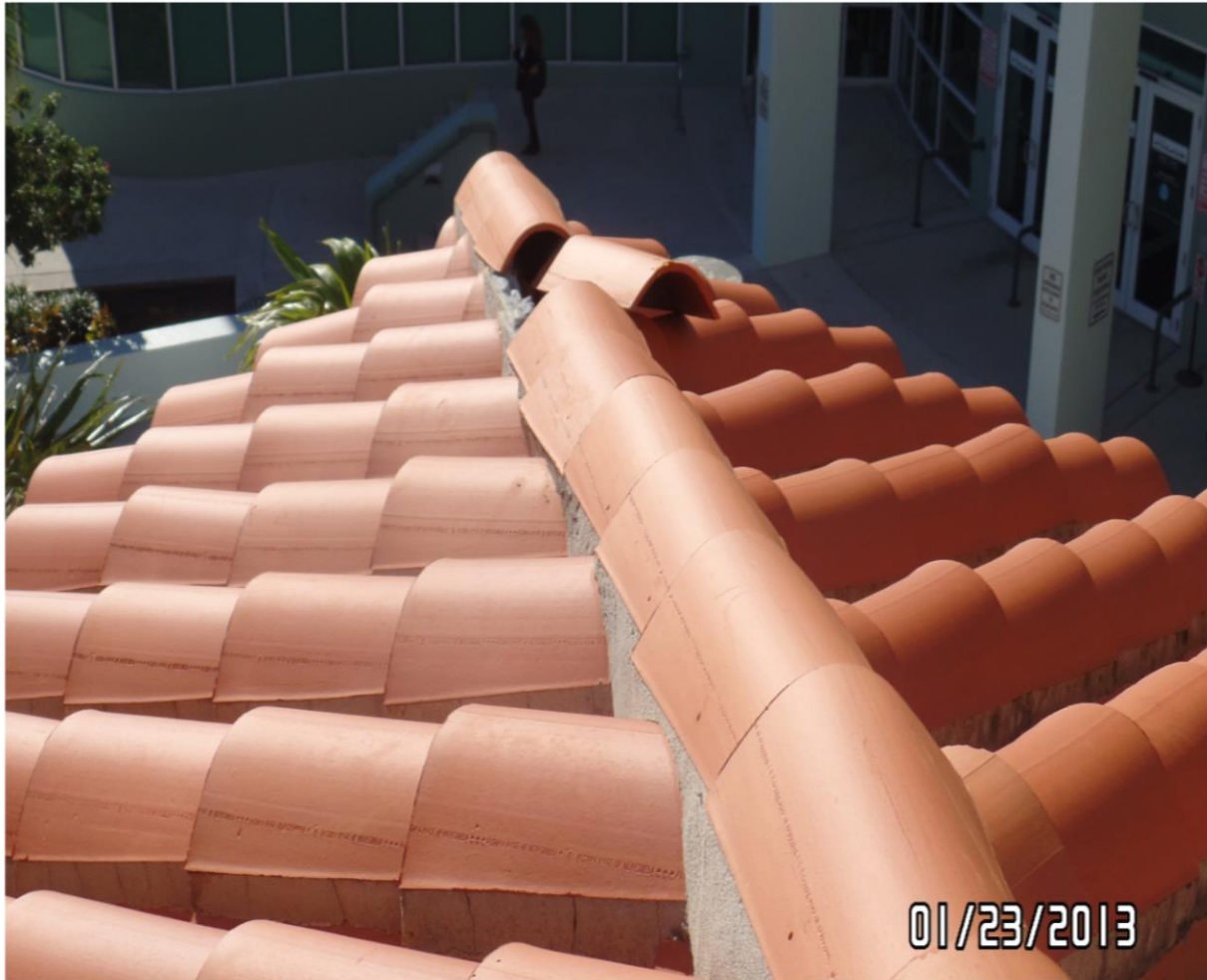
17. MISSING RIDGE CAP TILES
