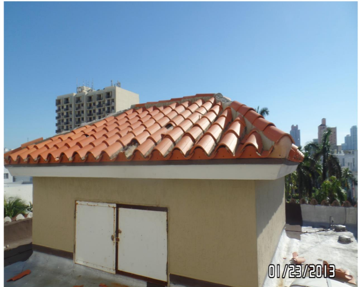
12. BROKEN AND MISSING TILES ON PENTHOUSE ROOF_2
