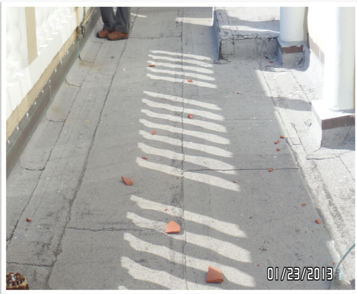
32. TILE DEBRIS AND WEATHERED MODIFIED BITUMEN MEMBRANE
