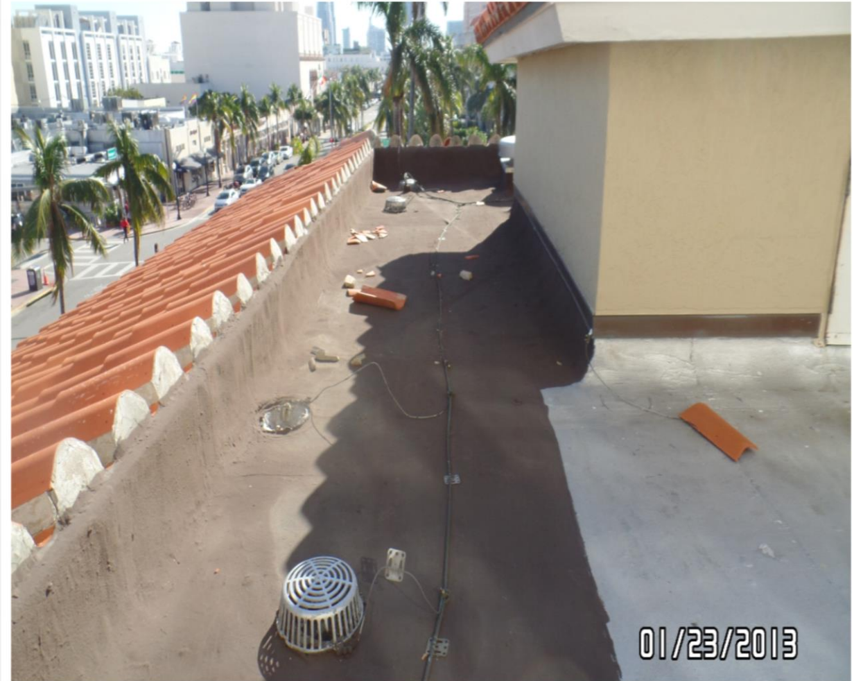
10. MISSING DRAIN GRATE COVER AND BROKEN BARREL TILES ON ROOF OVER COURTROOM AREA 2-1
