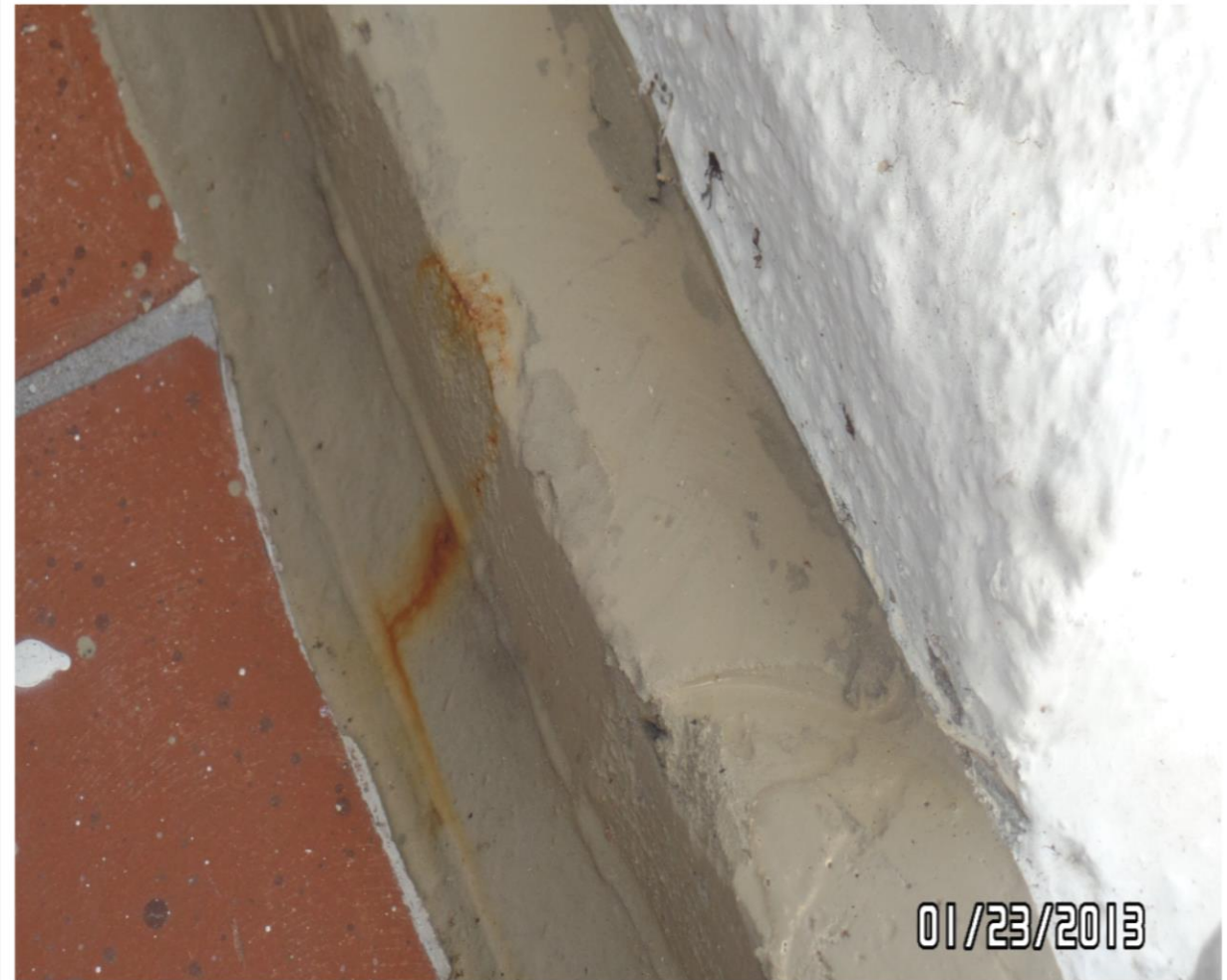
28. RUST COMING FROM WATER INTRUSION OF THE 8 TH FLOOR BALCONY DECK
