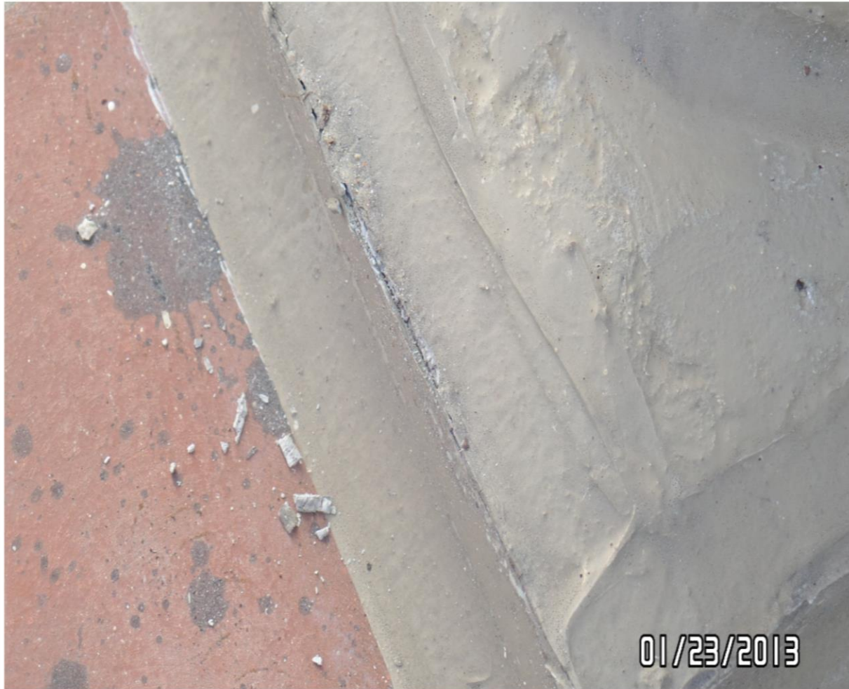
25. MASONRY CRACKS IN CONCRETE COLUMNS OF 8 TH FLOOR WEST
