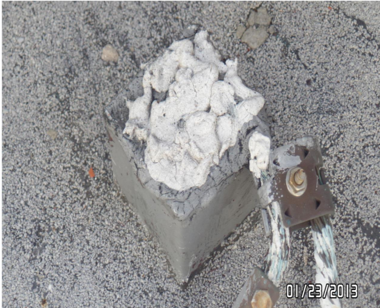
33. FAILING CAULKING AND PITCH PAN FILLER THAT IS TYPICAL ON THIS ROOF SECTION
