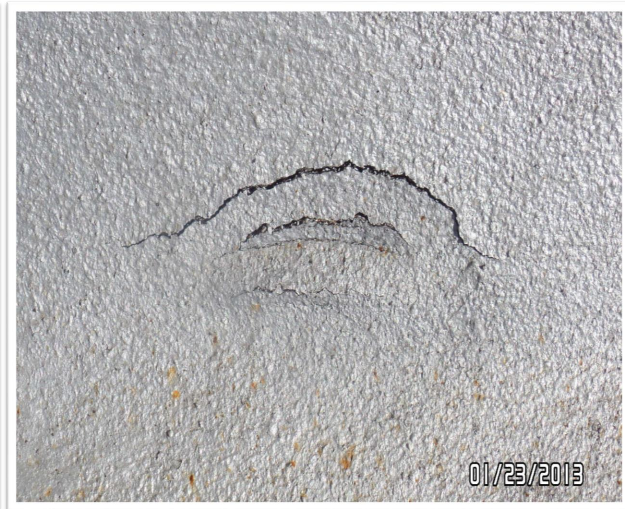
16. HOLE IN BASE FLASHING SYSTEM OF SOUTH ROOF
