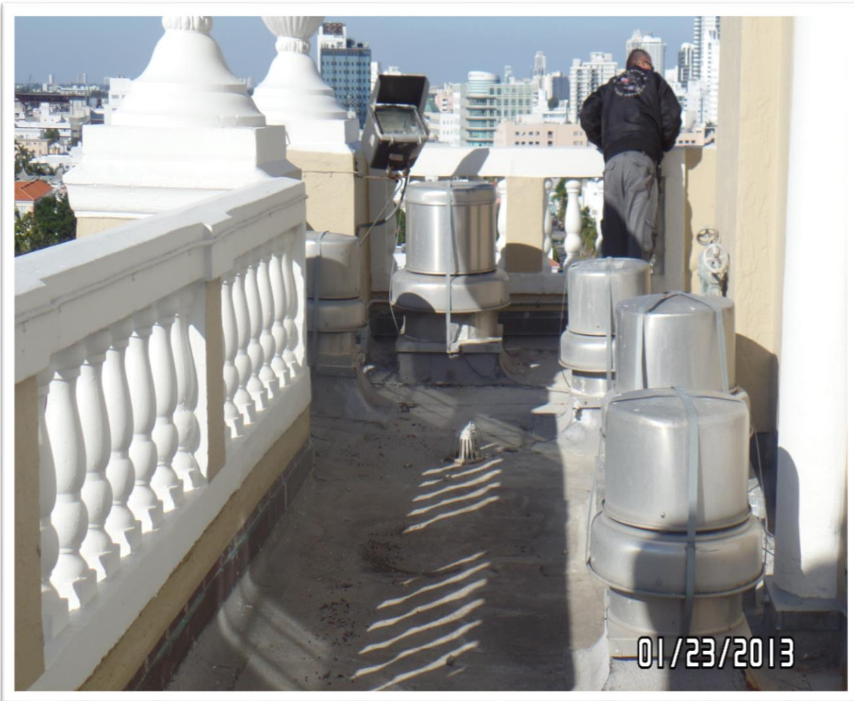
35. OVERVIEW OF MECHANICAL VENTS MOUNTED ON 9 TH FLOOR ROOF
