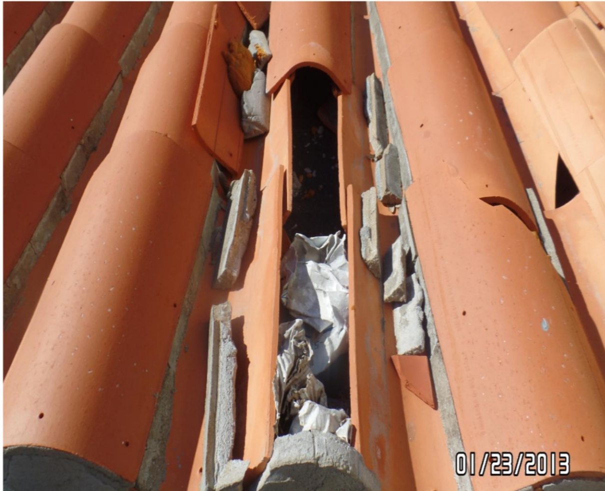
13. BROKEN AND MISSING TILES ON PENTHOUSE ROOF_3
