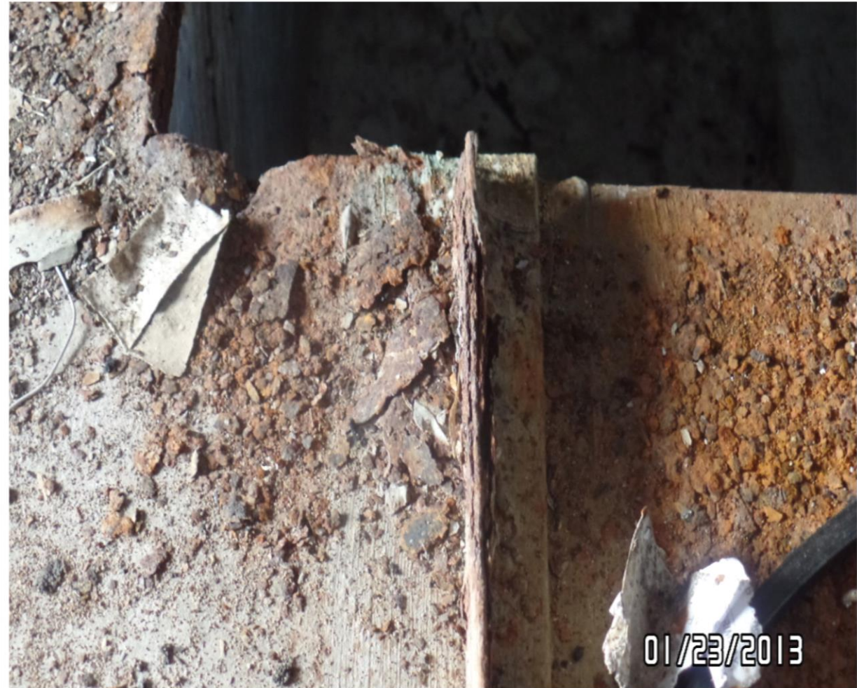
22. RUSTED DUCT SECTIONS WITHIN EQUIPMENT ROOM PENTHOUSE OVER COURTROOM 2-1
