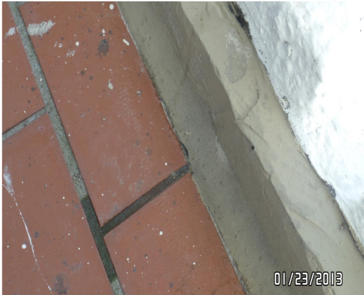
27. TILE AT OUTSIDE WALL IS SHOWING SIGNS OF WATER LEAKAGE
