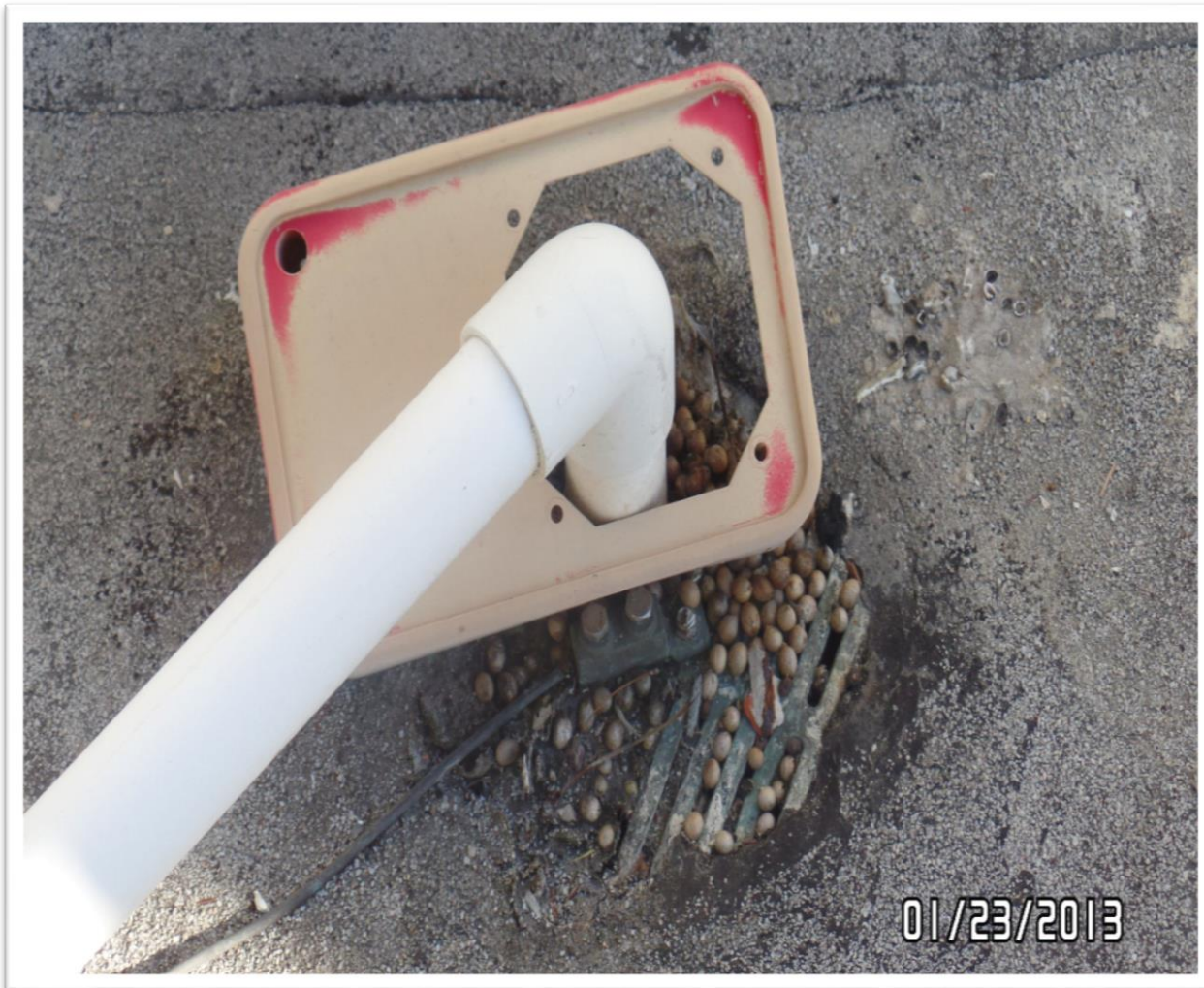
31. BLOCKED INTERNAL DRAIN WITH SEEDS ON THE 9 TH FLOOR ROOF
