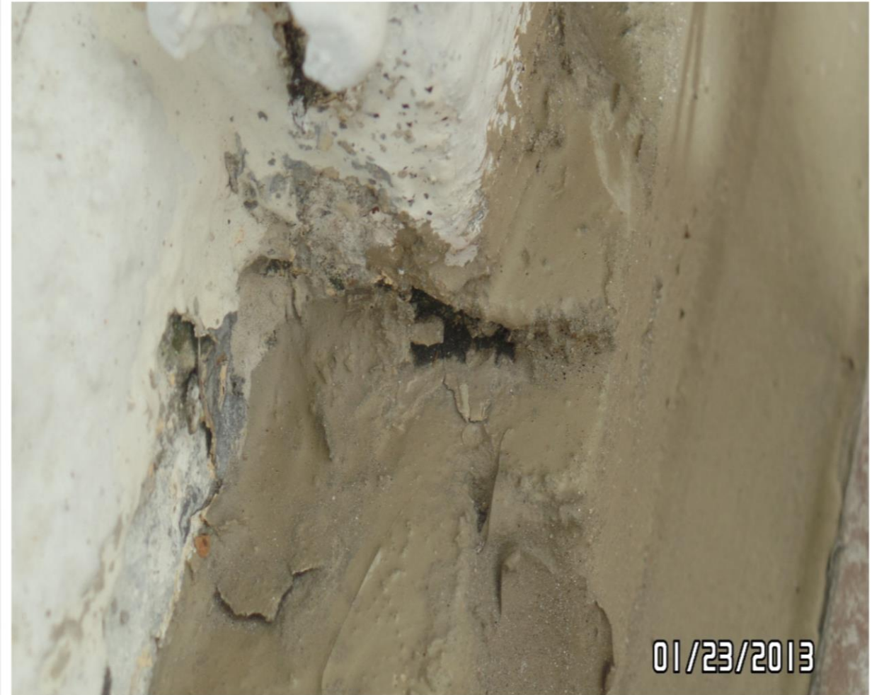
26. FLASHING OPENINGS AT PERIMETER OF BALCONY ON THE 8 TH FLOOR WEST
