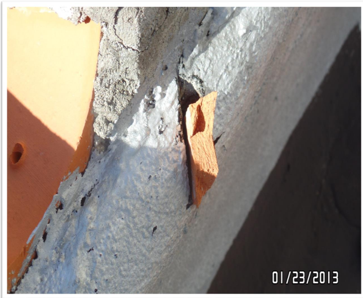
15. TILE IMPALED IN BASE FLASHING SYSTEM FROM HURRICANE IRMA- SOUTH ROOF
