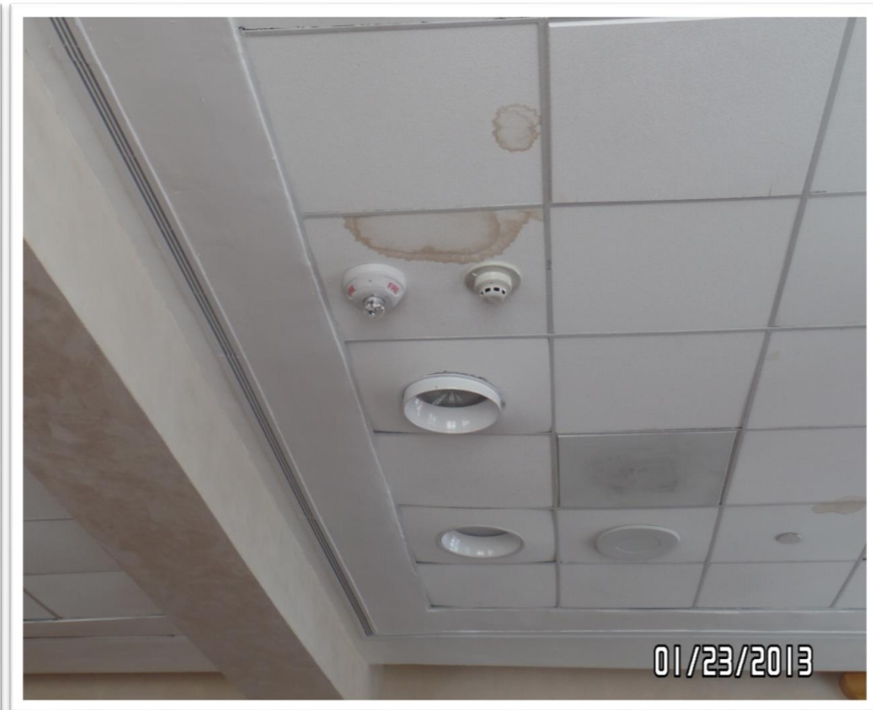
4. LEAK IN CEILING_1 IN COURTROOM 2-1
