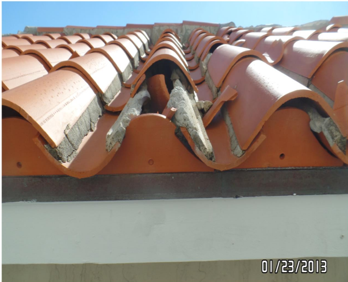
11. BROKEN AND MISSING BARREL TILES ON PENTHOUSE ROOF_1
