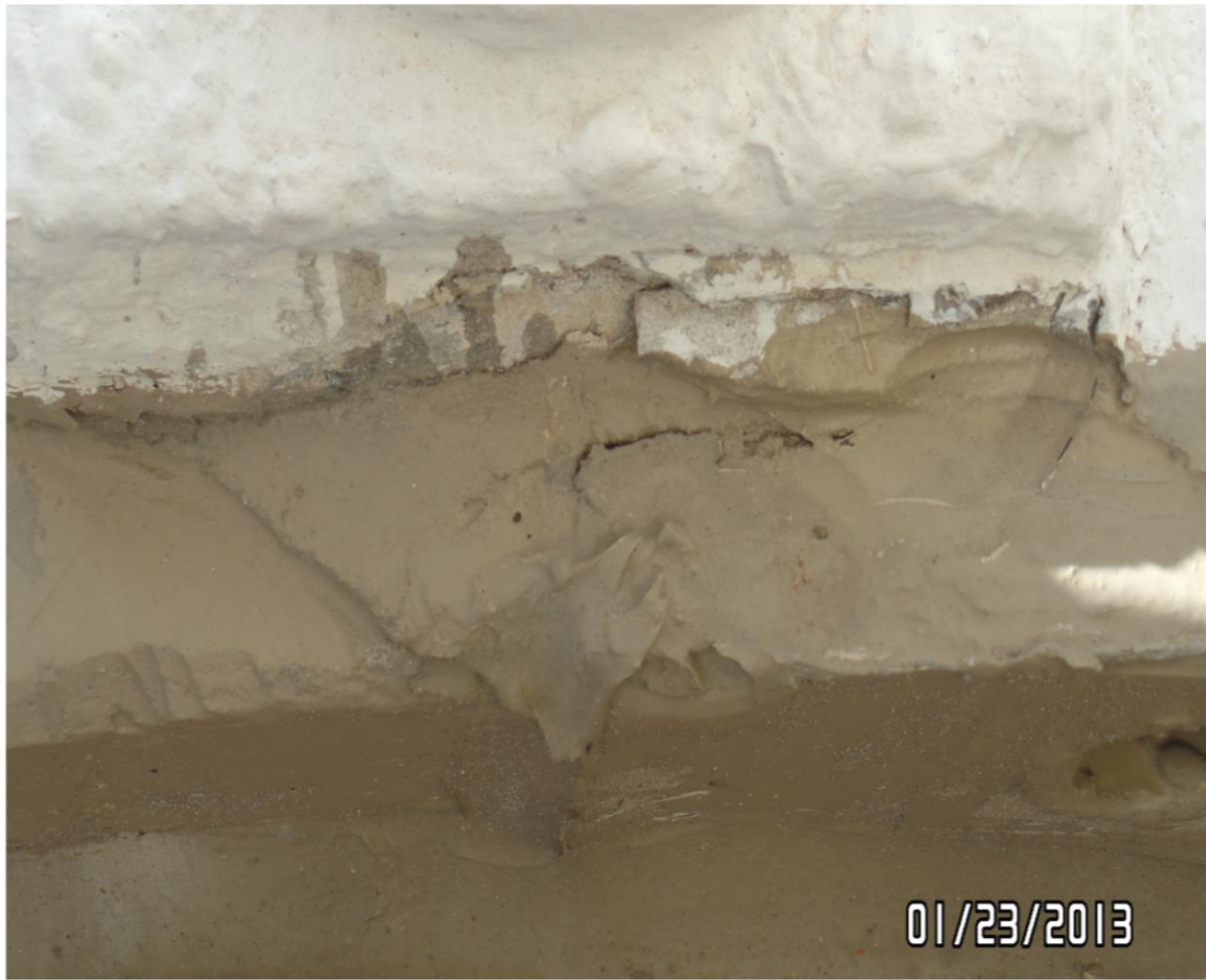
29. CRACKS IN THE OUTSIDE BALCONY FLASHING PERIMETER
