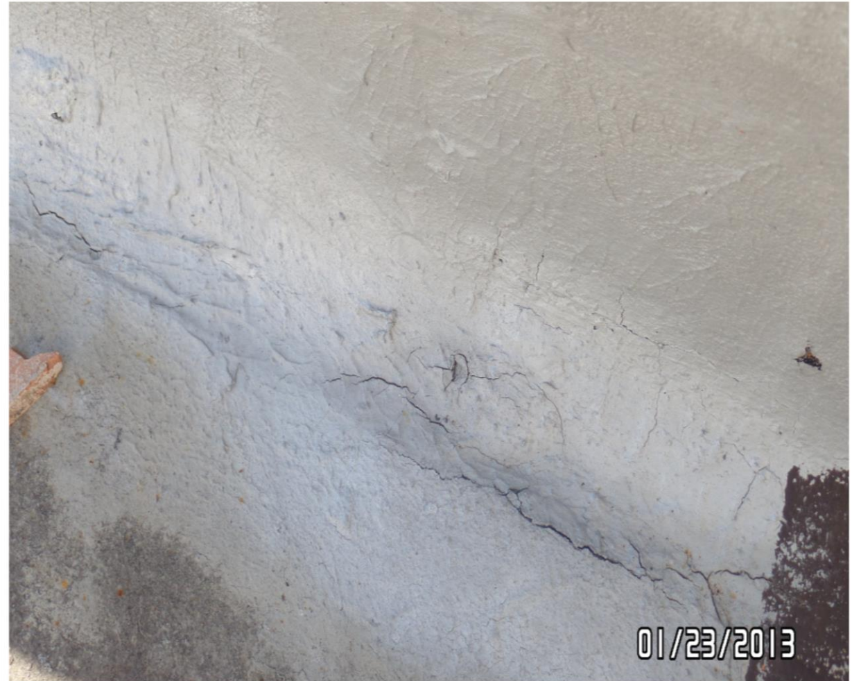
14. CRACKS, HOLES AND DETERIORATION IN BASE FLASHING SYSTEM DUE TO AGE AND UV EXPOSURE
