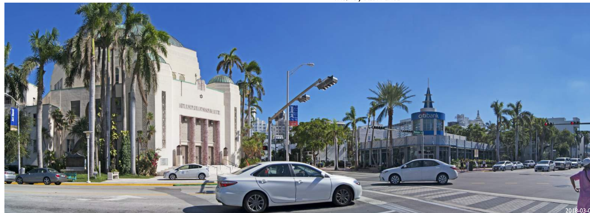
4. INTERSECTION OF WASHINGTON AVENUE AND 17H STREET, VIEW OF PROPERTY
