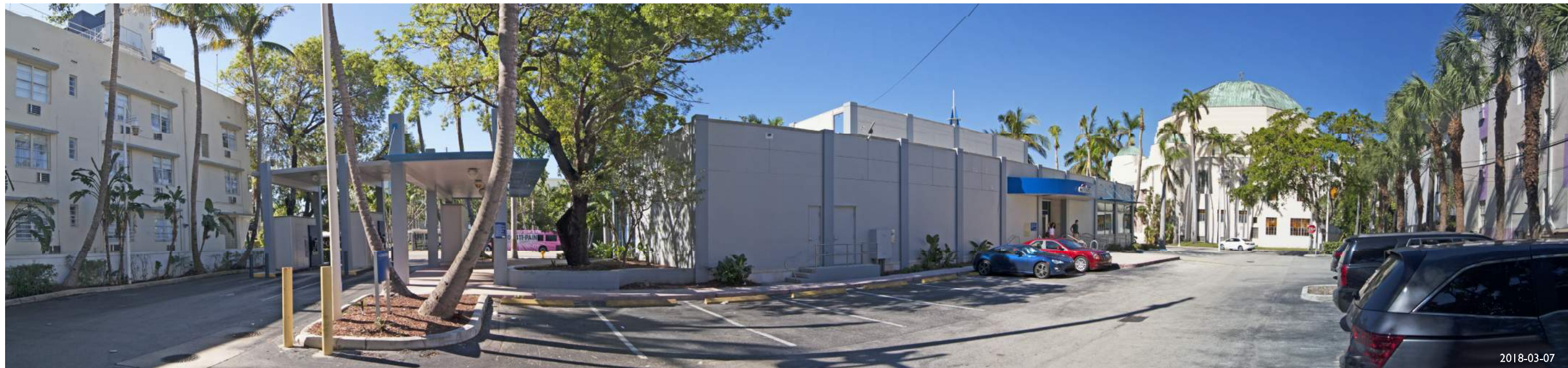
12. VIEW TOWARDS NEIGHBORING STRUCTURES FROM THE CITIBANK PARKING
