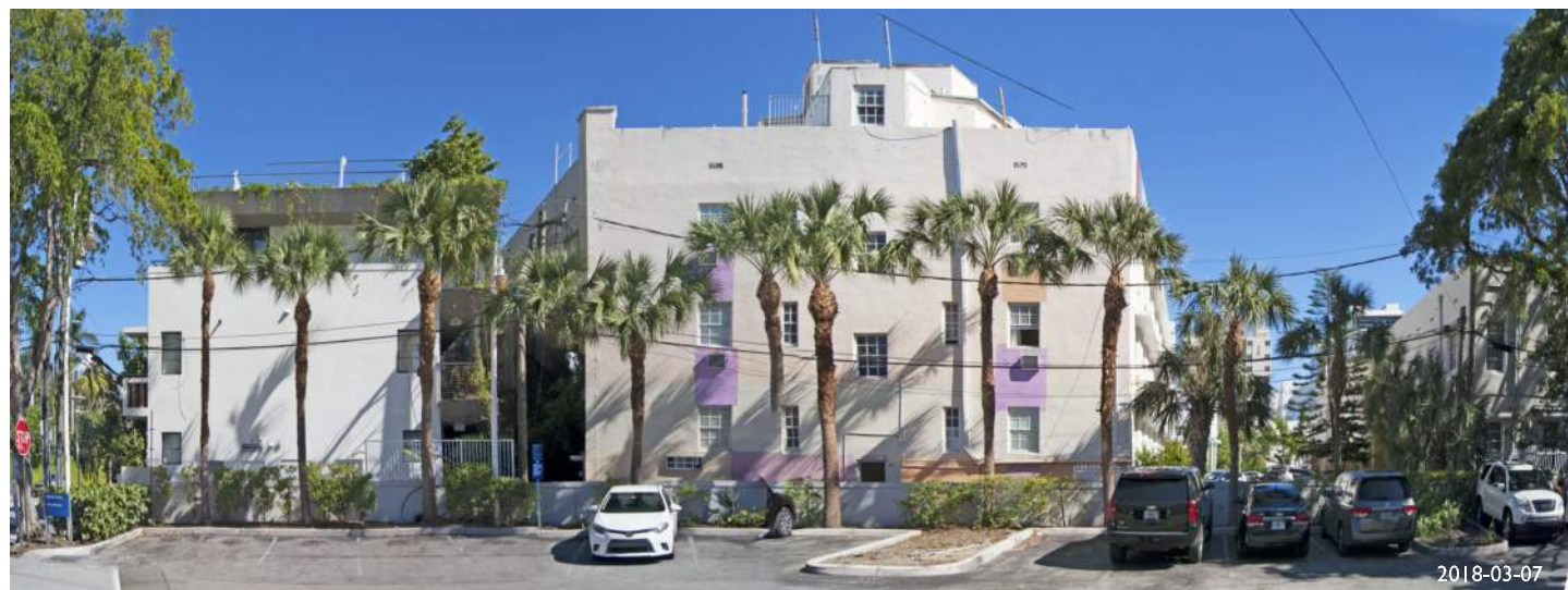
9. VIEW TOWARDS NEIGHBORING STRUCTURES FROM THE CITIBANK PARKING
