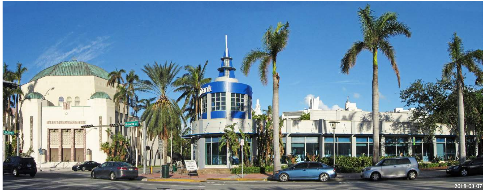
2018-03-07 2. SITE FACING WASHINGTON AVENUE
