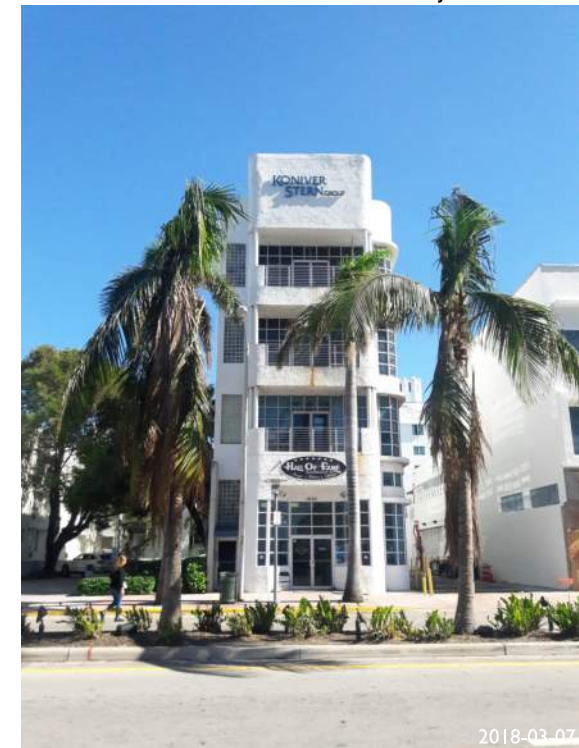
15.VIEW TOWARDS EAST OF OFFICE BUILDING
