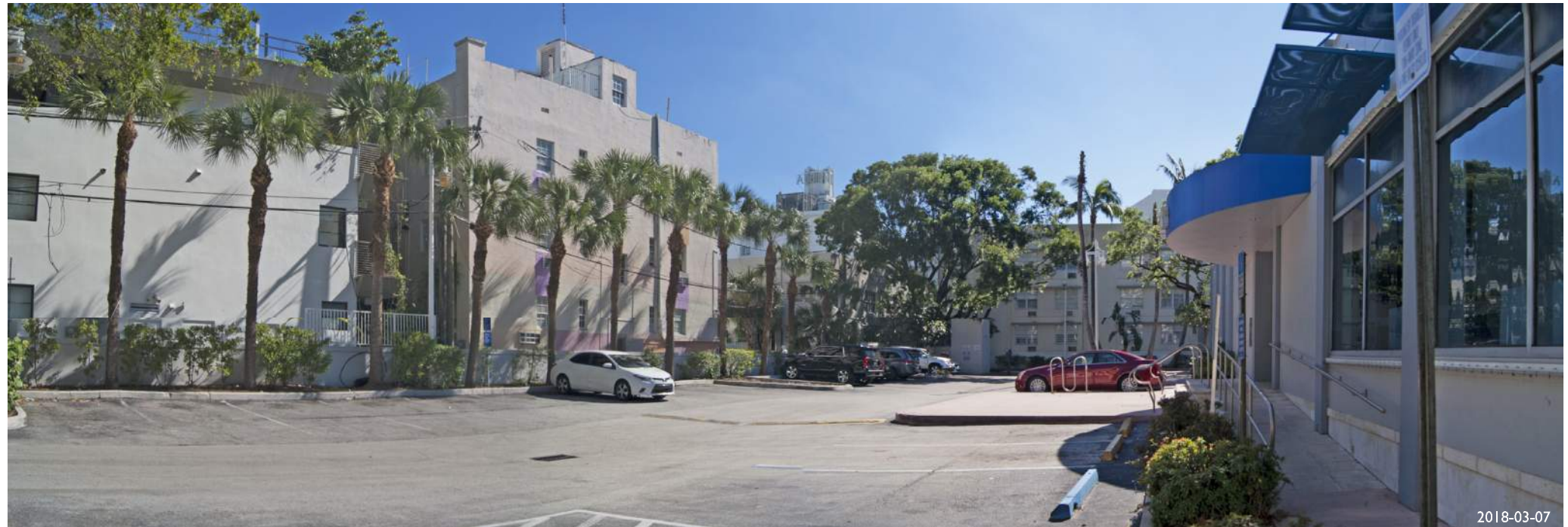
11. VIEW TOWARDS NEIGHBORING STRUCTURES FROM THE CITIBANK PARKING
