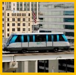
Automated People Mover Vehicle (APM)
