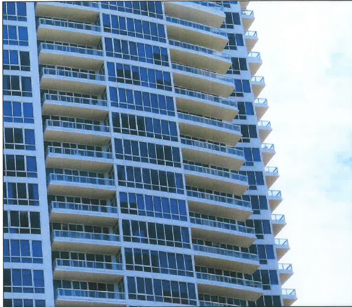
EXISTING CONDITION CLOSE UP
