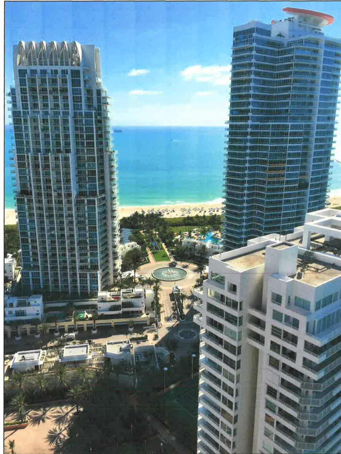
NORTH AND SOUTH TOWER
