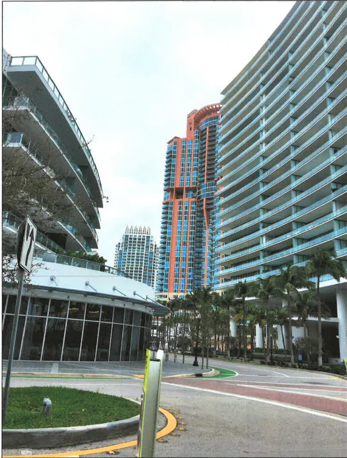
WEST END OF SOUTH POINTE DRIVE
