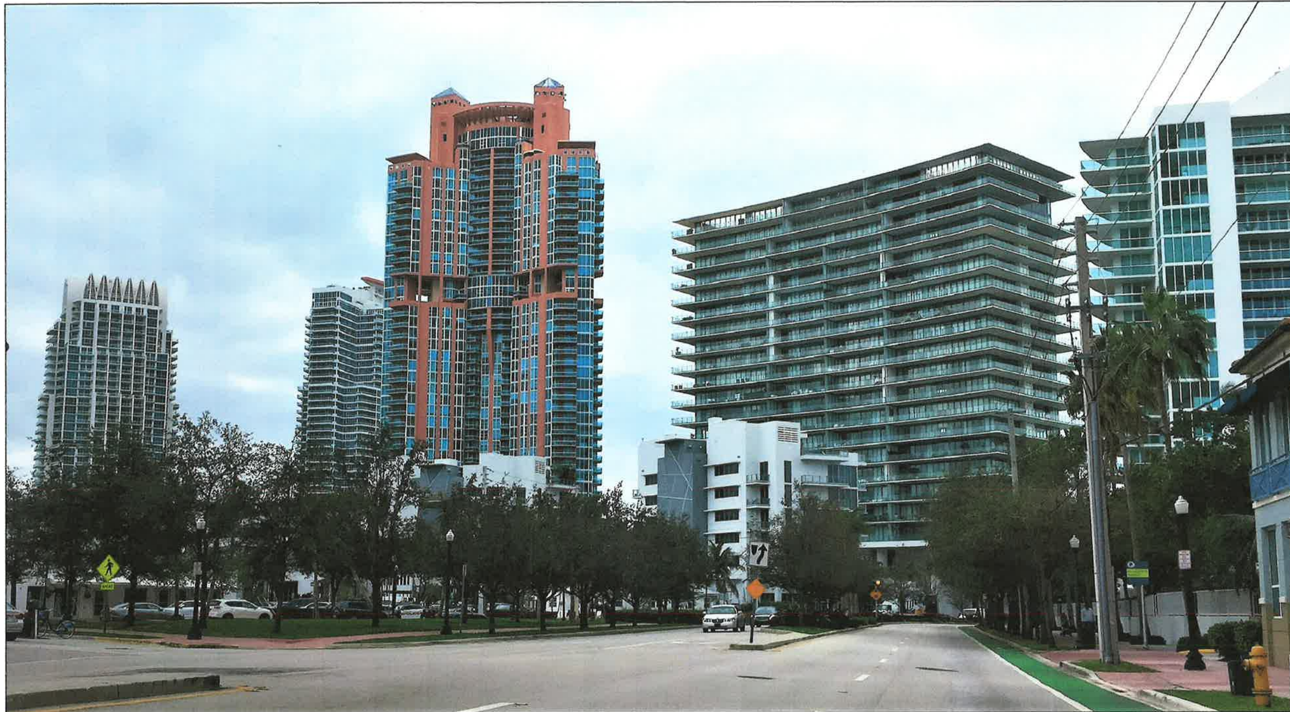
SOUTH POINTE DRIVE
