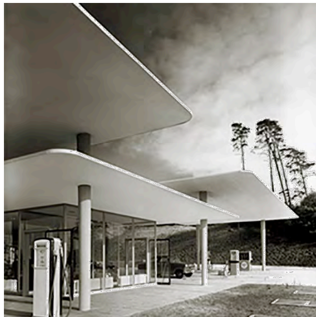
SI TAPERED CANOPIES: WHITE SMOOTH-COAT STUCCO
