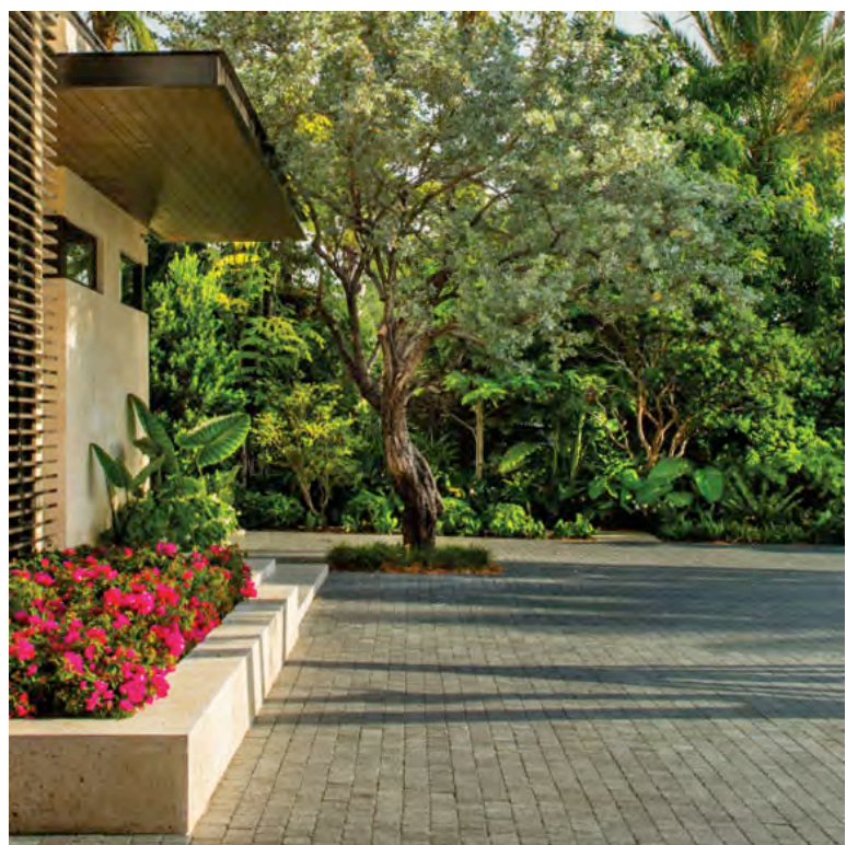
ST3 DRIVEWAY: GREY GRANITE COBBLESTONES
