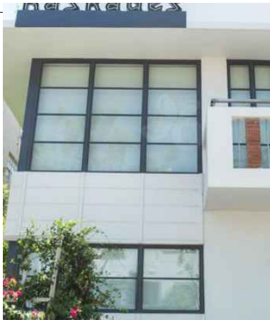
ALUMINUM GLASS STOREFRONT WITH BLACK ANODIZED FINISH TO MATCH EXISTING
