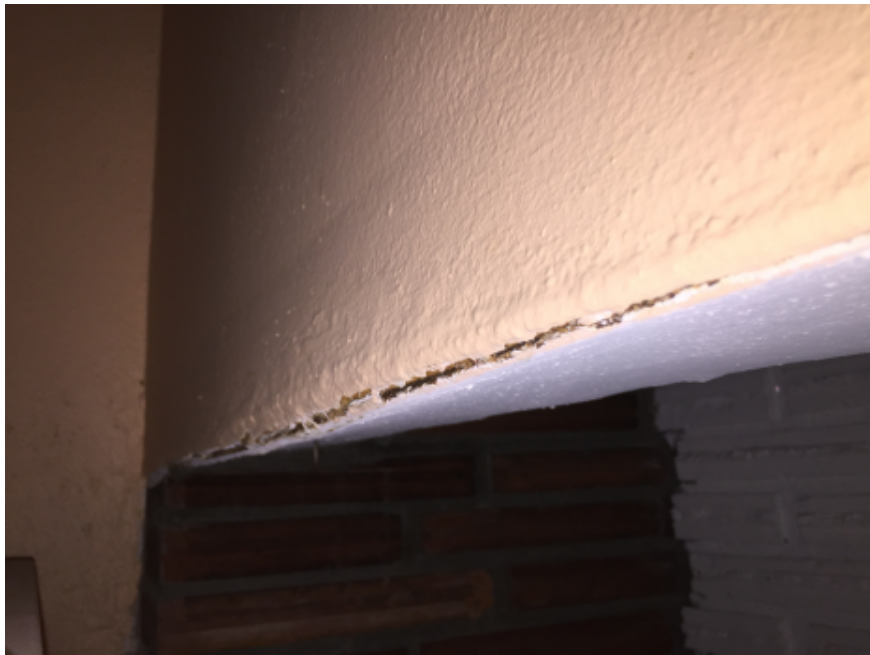
Photo #7: Interior header showing damaged finishing from possible structural damage.
