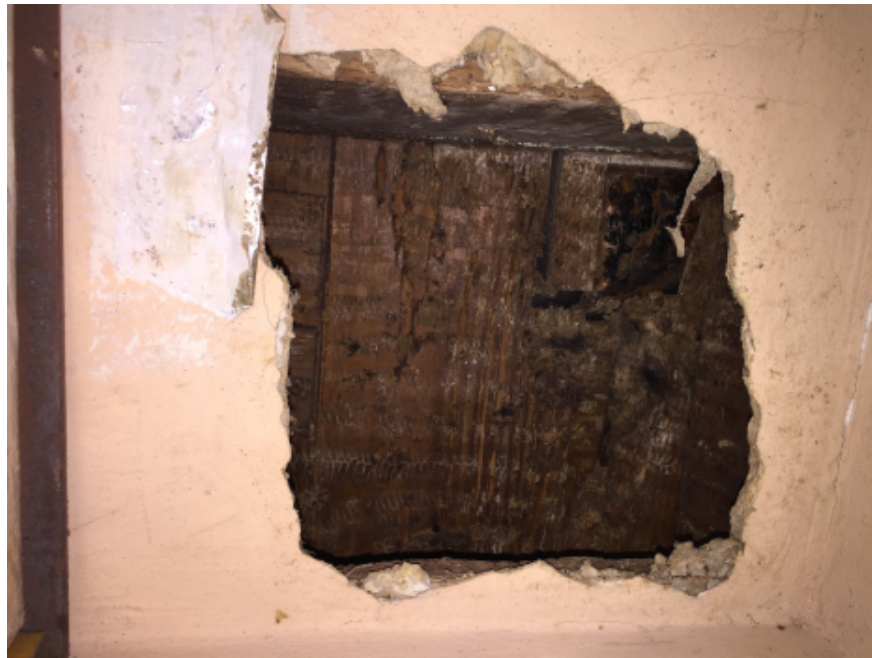
Photo #15: Roof sheathing with signs of water intrusion.
