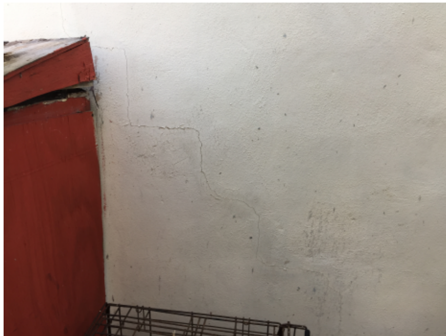
Photo #1: Step ladder cracks on CMU wall at West side of residence
