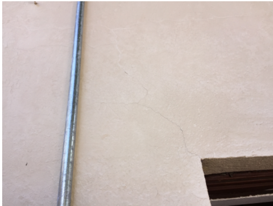
Photo #2: Crack at upper left corner of window opening at West side of residence
