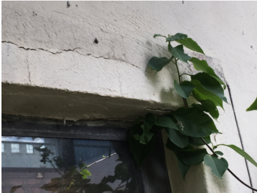
Photo #4: Header showing big cracks and spalled concrete at upper right corner
