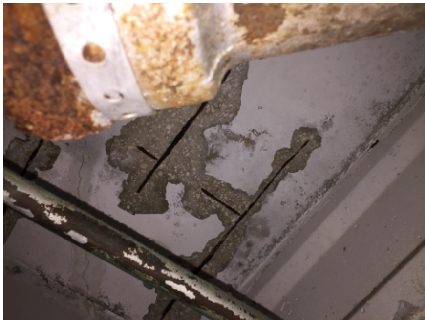
Photo #10: Concrete spalled and exposed bottom reinforcement of 2 nd floor slab due to corrosion.
