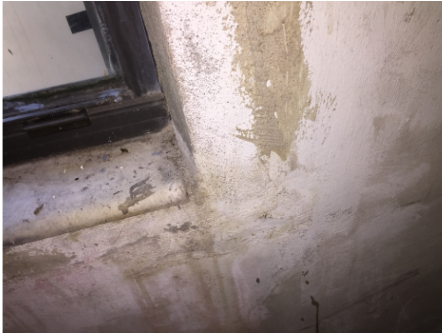
Photo #13: Patching from previous repair work.
