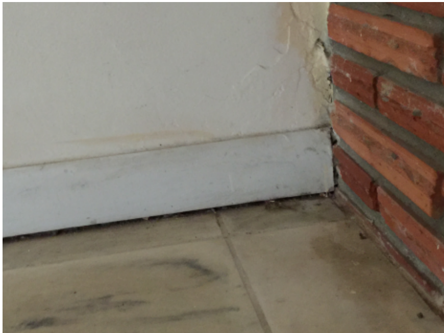
Photo #8: Gap between base board and top of finished floor is indicative of ground floor slab settlement.
