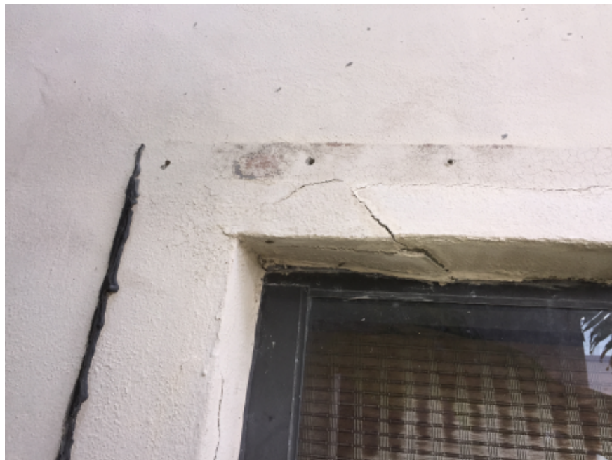
Photo #3: Header showing big cracks and spalled concrete at upper left corner
