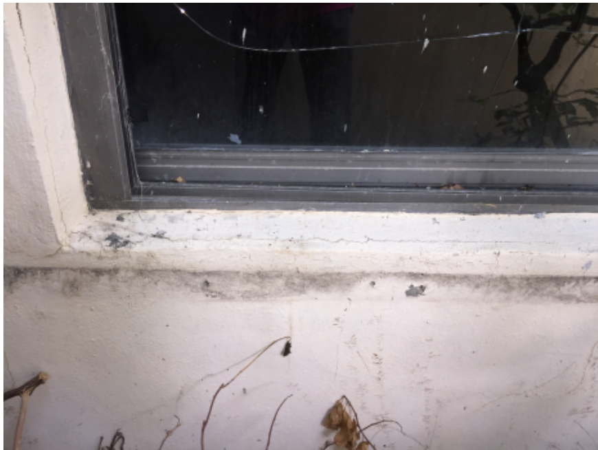
Photo #5: Cracks at sill and jamb of window opening
