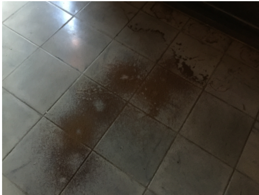
Photo #17: Wood residues at floor. Sign of insects activity.
