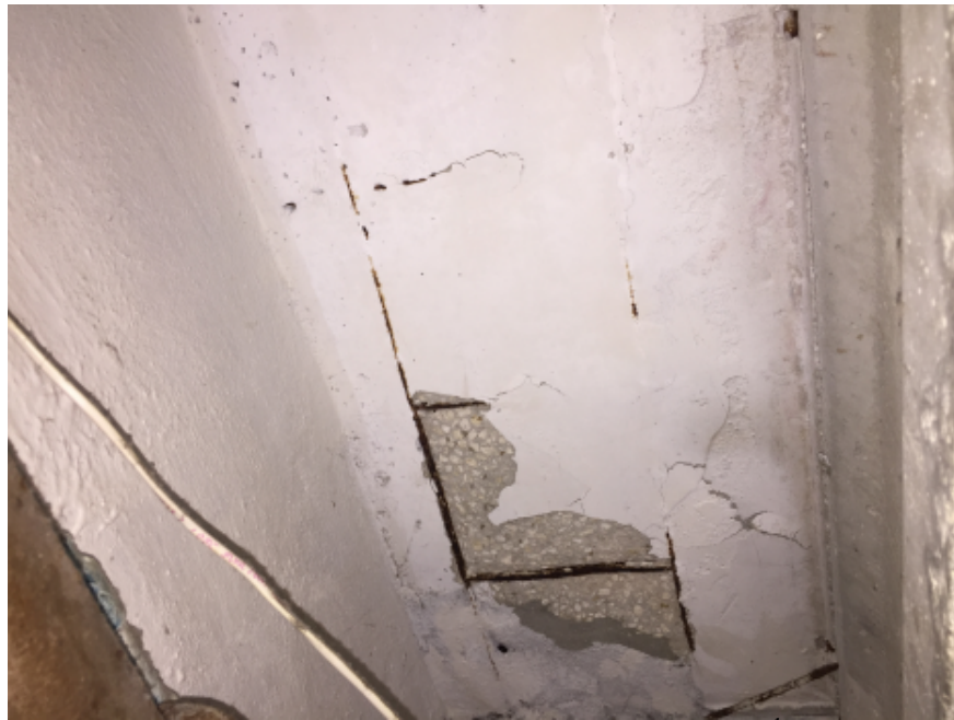
Photo #11: Concrete spalled and exposed bottom reinforcement of 2 nd floor slab due to corrosion.
