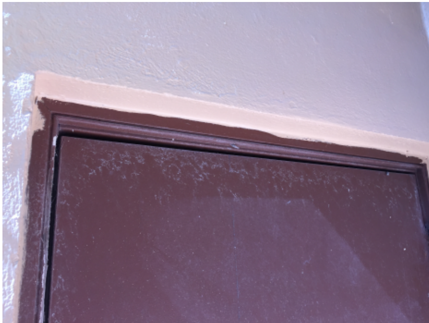
Photo #14: Uneven top and jambs of door plus difficulty to operate are signs of differential settlement.
