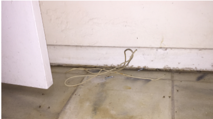
Photo #9: Gap between base board and top of finished floor is indicative of ground floor slab settlement.
