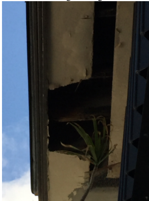
Photo #16: Roof overhang with signs of water intrusion and deterioration at tip of framing members.
