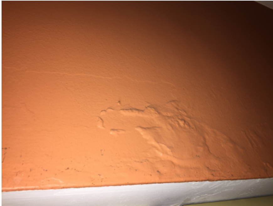
Photo #6: Water blisters at interior side of envelope walls. Evidence of water intrusion.
