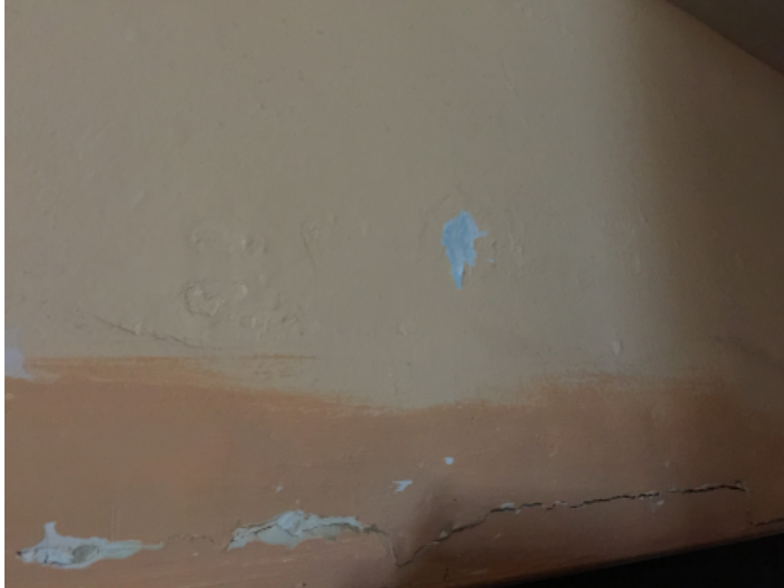
Photo #8: Interior header showing damaged finishing from possible structural damage.
