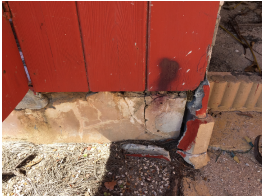
Photo #12: Spalled concrete at top of stem wall. Indicative of corrosion process.
