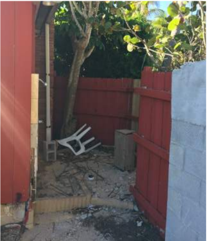
IMG 2: EXISTING WOOD FENCE FACING NORTH
