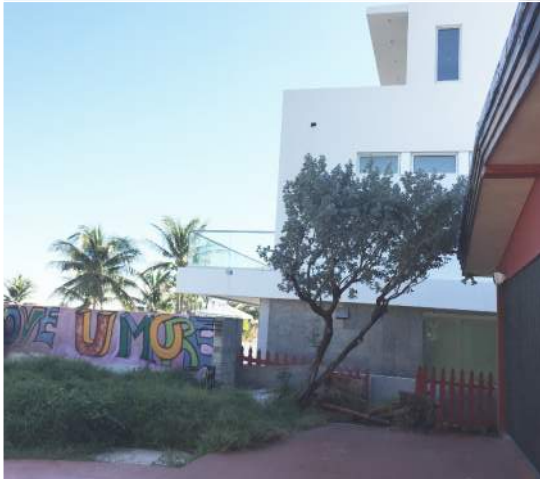
IMG 5: EXISTING CONCRETE WALL AND WOOD FENCE FACING SOUTH
