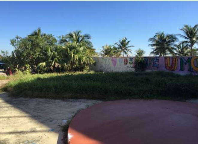
IMG 4: EXISTING CONCRETE SLAB AND CONCRETE WALL FACING SOUTH
