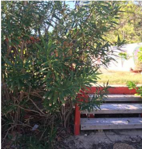
IMG 2: EXISTING CONCRETE SLAB AND WOODEN STAIRS
