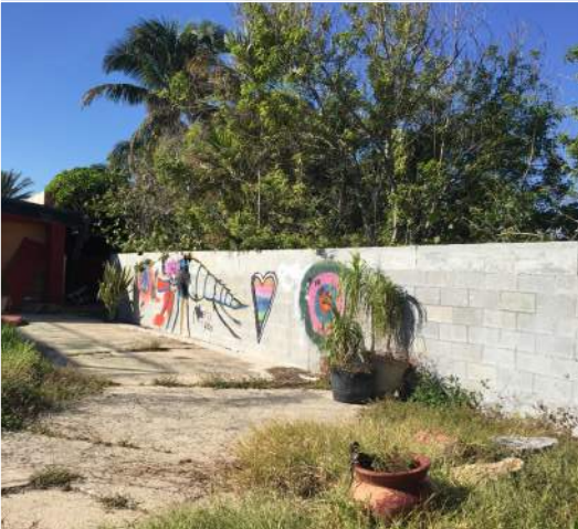
IMG 1: EXISTING CONCRETE WALL FACING NORTH
