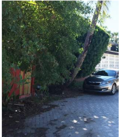
IMG 6: EXISTING WOOD FENCE FACING NORTH
