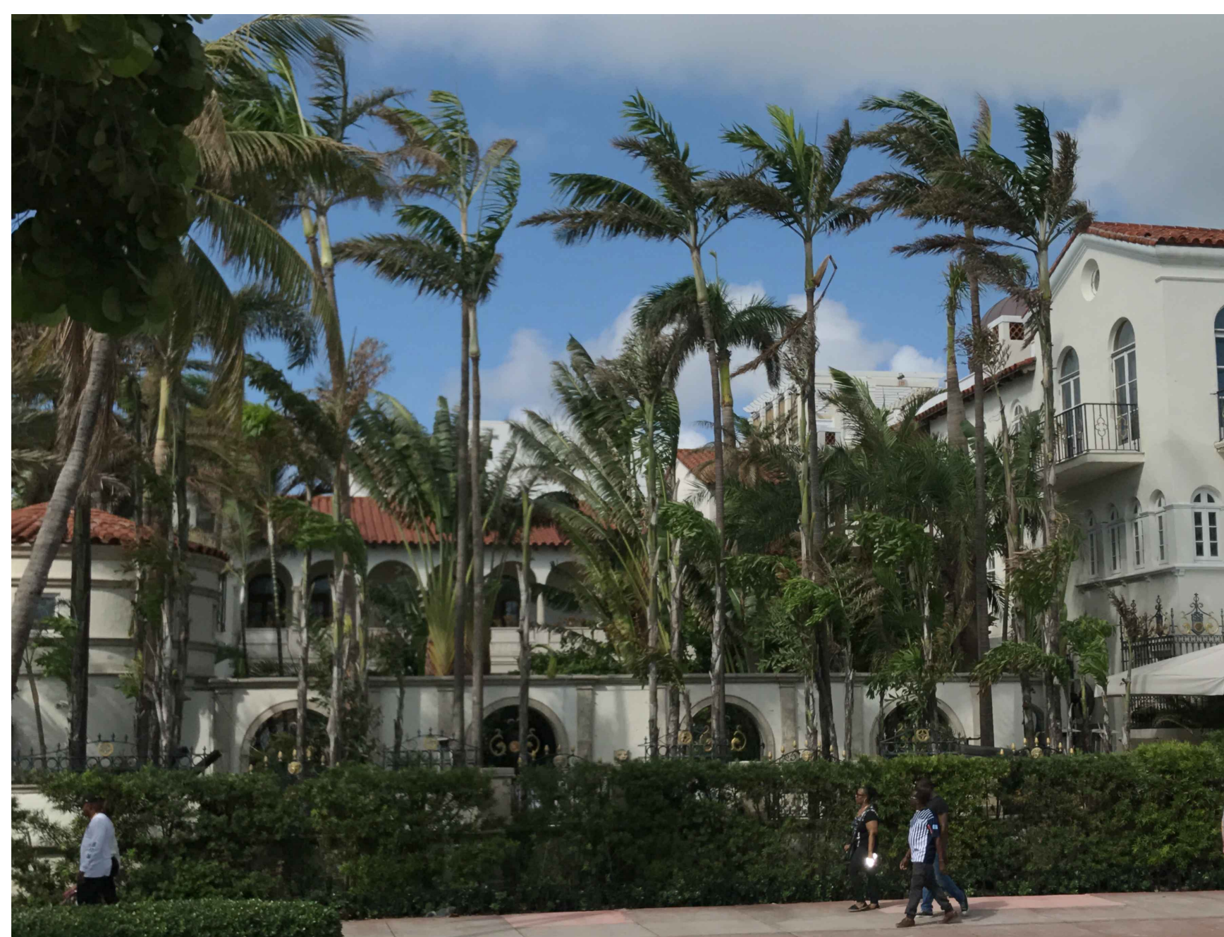
A. VIEW FROM OCEAN DRIVE. TALL MONTGOMERY PALMS + FISHTAILS IN POOR CONDITION TO BE REMOVED
