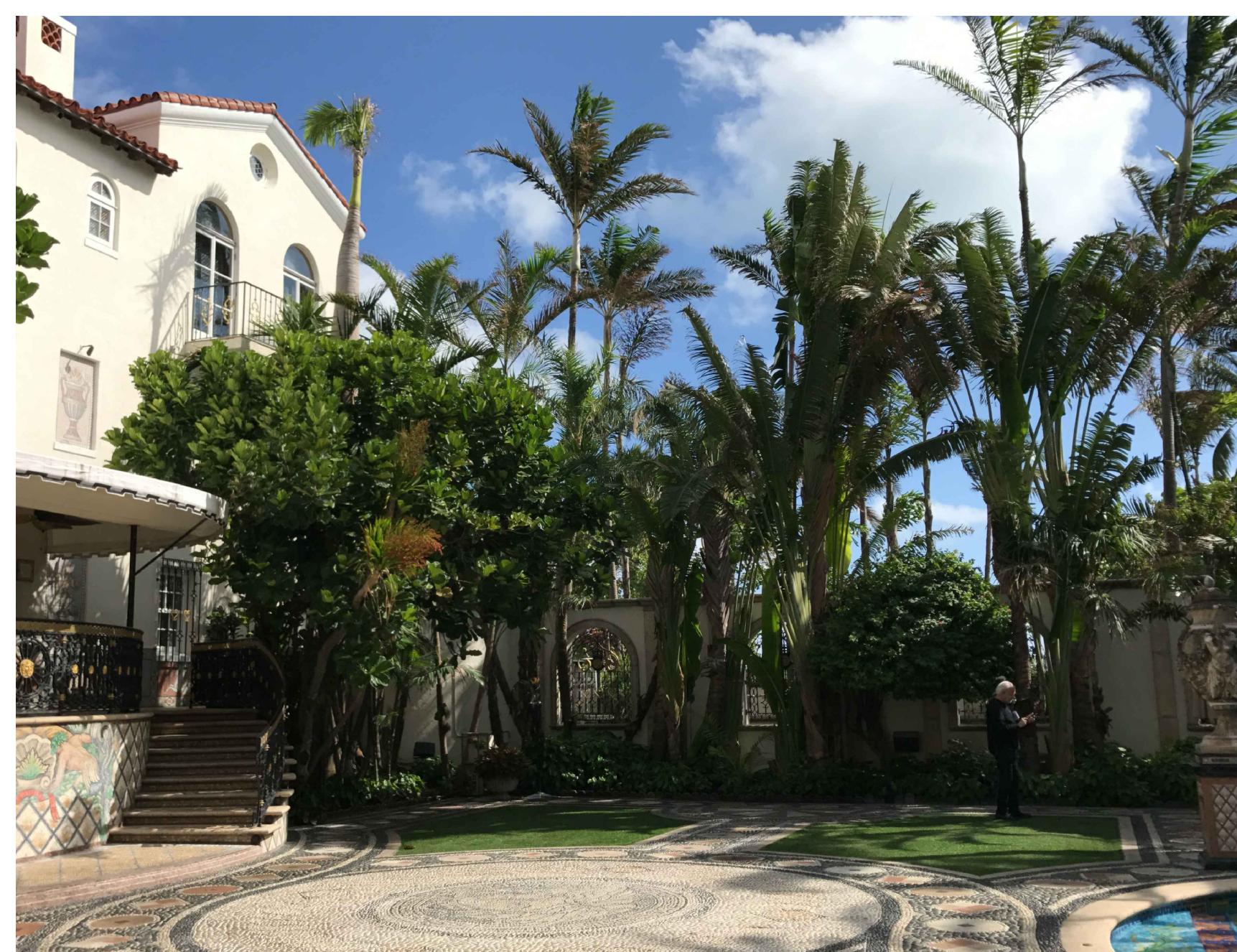
E. VIEW FROM WEST SIDE OF COURTYARD LOOKING EAST TO PLANTER IN FRONT OF WALL THAT IS TO BE REMOVED.
