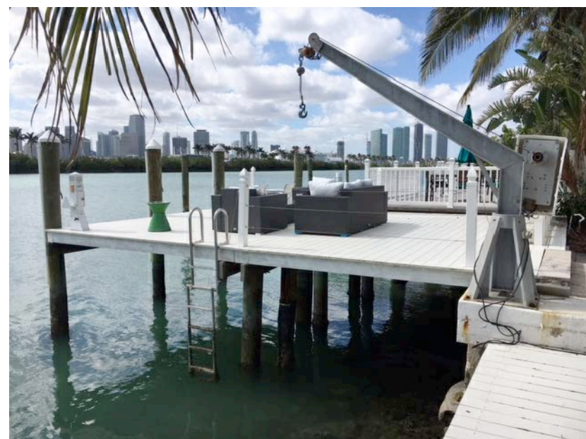
EXISTING DOCK TO REMAIN
