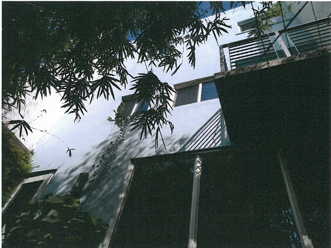
Existing Rear (west) Elevations (close-up)
