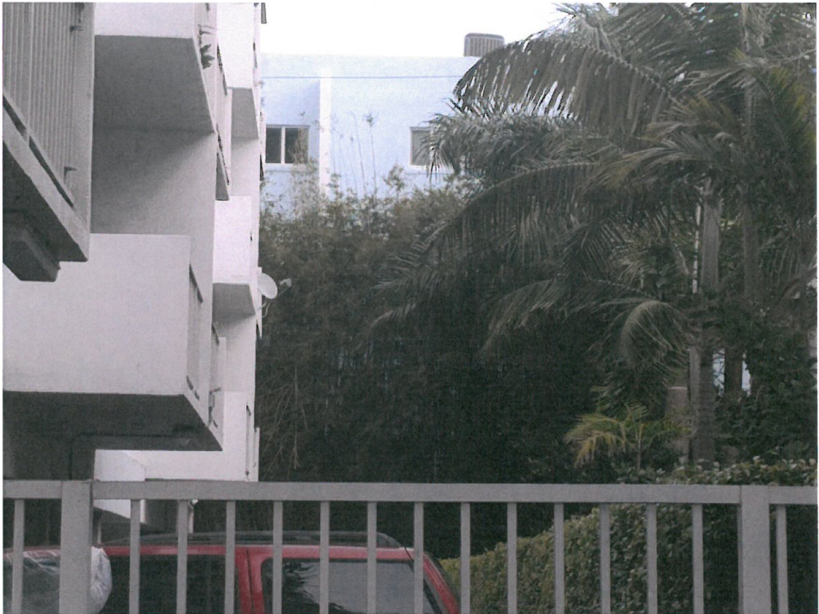
Existing Rear from Alton looking east
