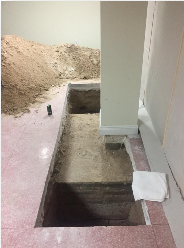
EXPLORATION OF EXISTING FOUNDATION AT PARTIAL BASEMENT
