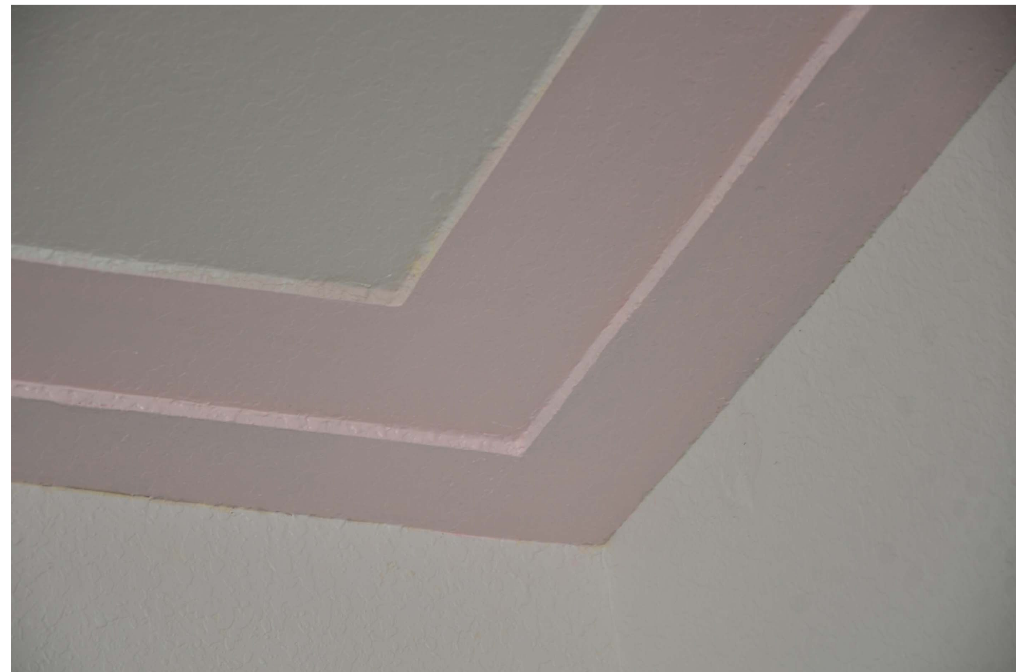
HISTORIC CEILING MOLDINGS AT LOBBY KEYNOTE 8
