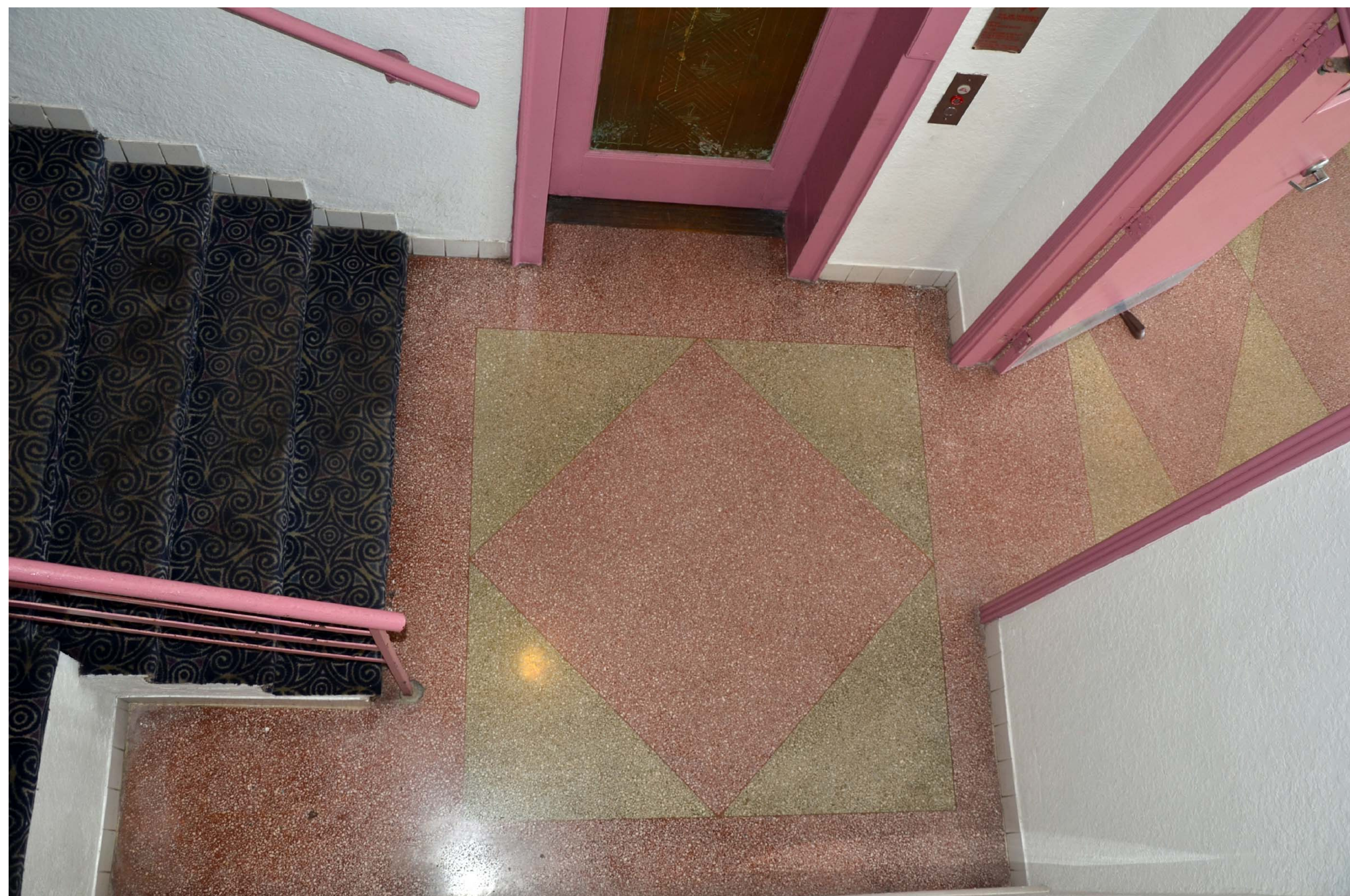
HISTORIC TERRAZZO AT ELEVATOR LOBBY - KEYNOTE 6
