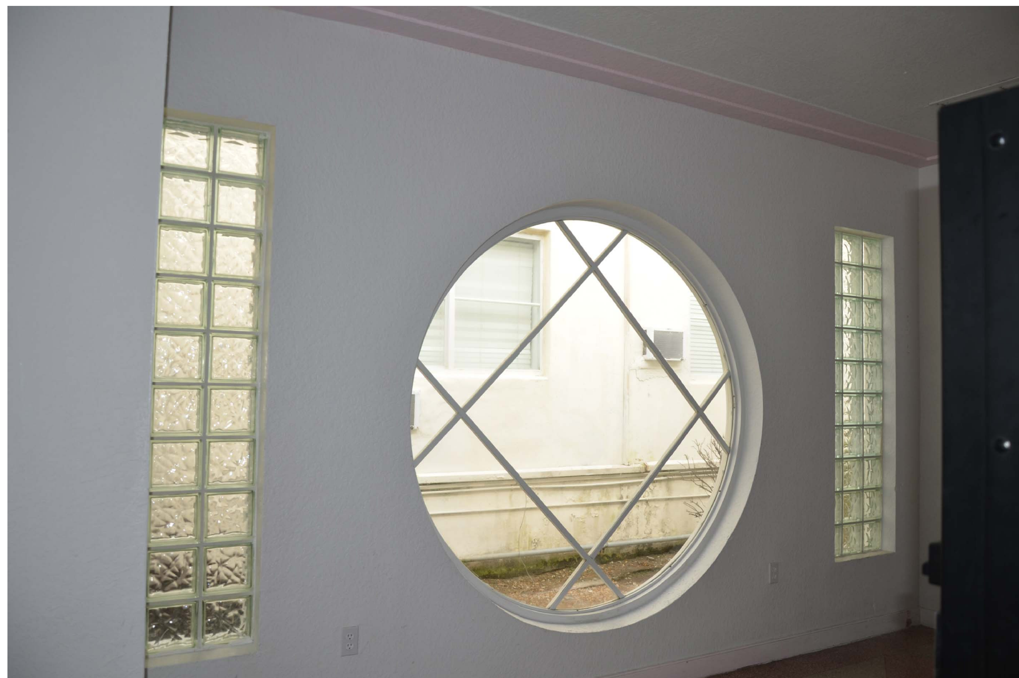
HISTORIC ROUND WINDOW FLANKED BY GLASS BLOCK LIGHTS
